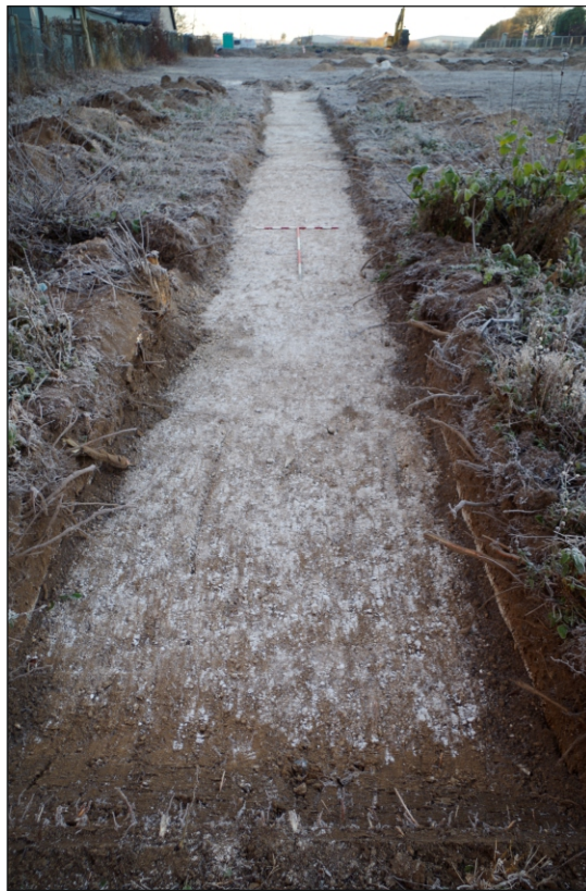
Plate 2: Trench 1 viewed from the south-west
