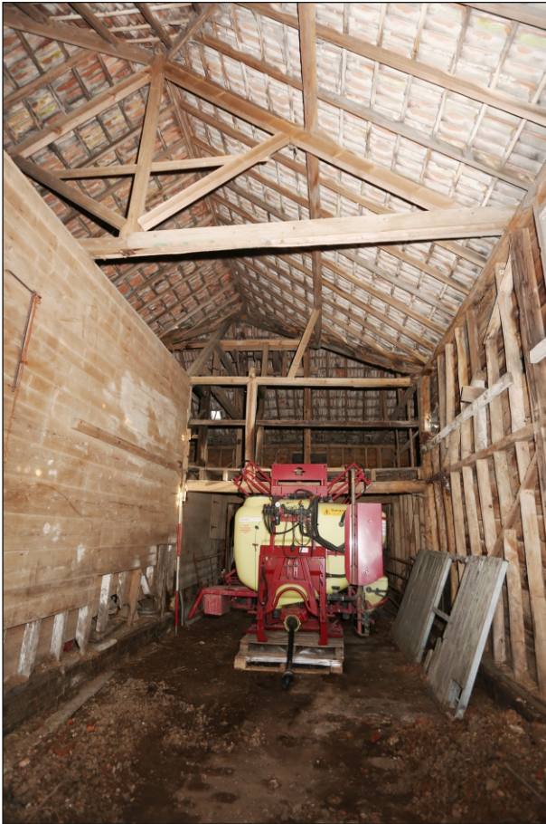
Plate 11: Building 2 large space viewed from the west
