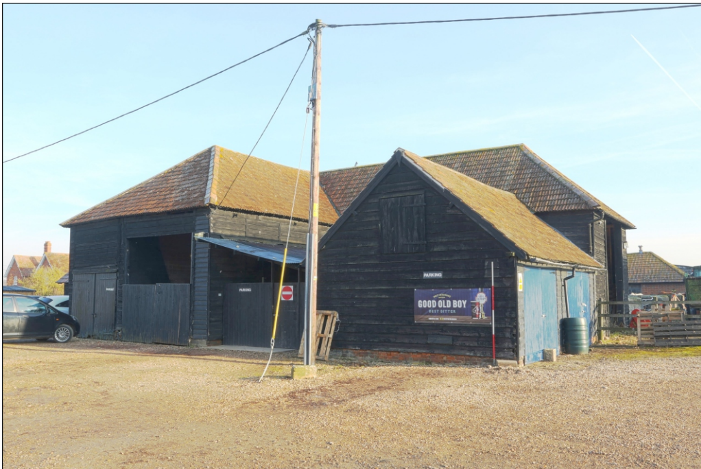
Plate 2: Redundant agricultural buildings viewed from the south-west. Buildings 2, 12 and 11 (left to right) in the foreground and Building 1 behind
