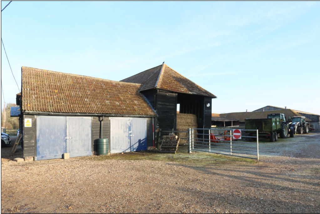
Plate 1: Redundant agricultural buildings viewed from the south-west. Buildings 11 and 1 in the foreground
