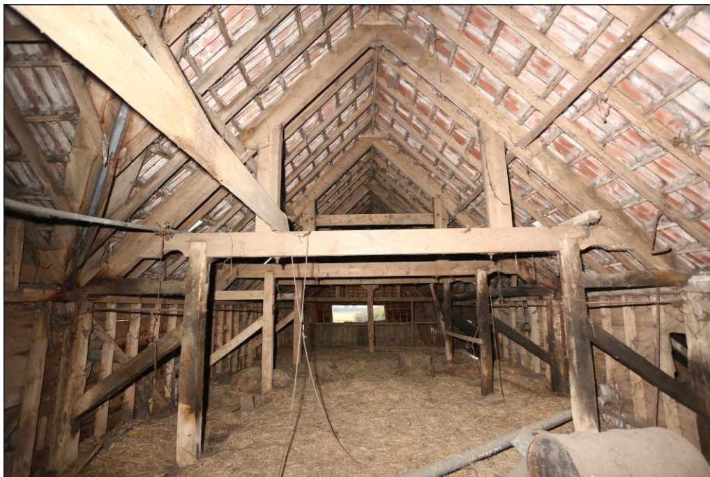
Plate 16: Building 3 first floor viewed from the north. Note the grease stained aisle timbers and holes cut for a line shaft
