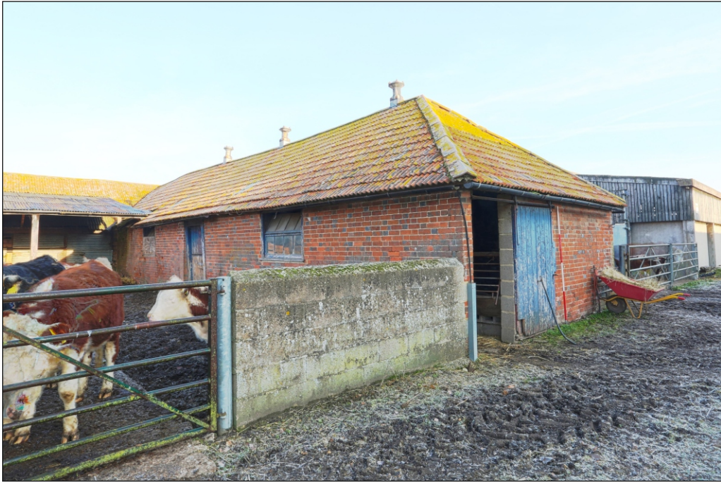
Plate 7: Redundant agricultural buildings viewed from the south-west, specifically Building 7
