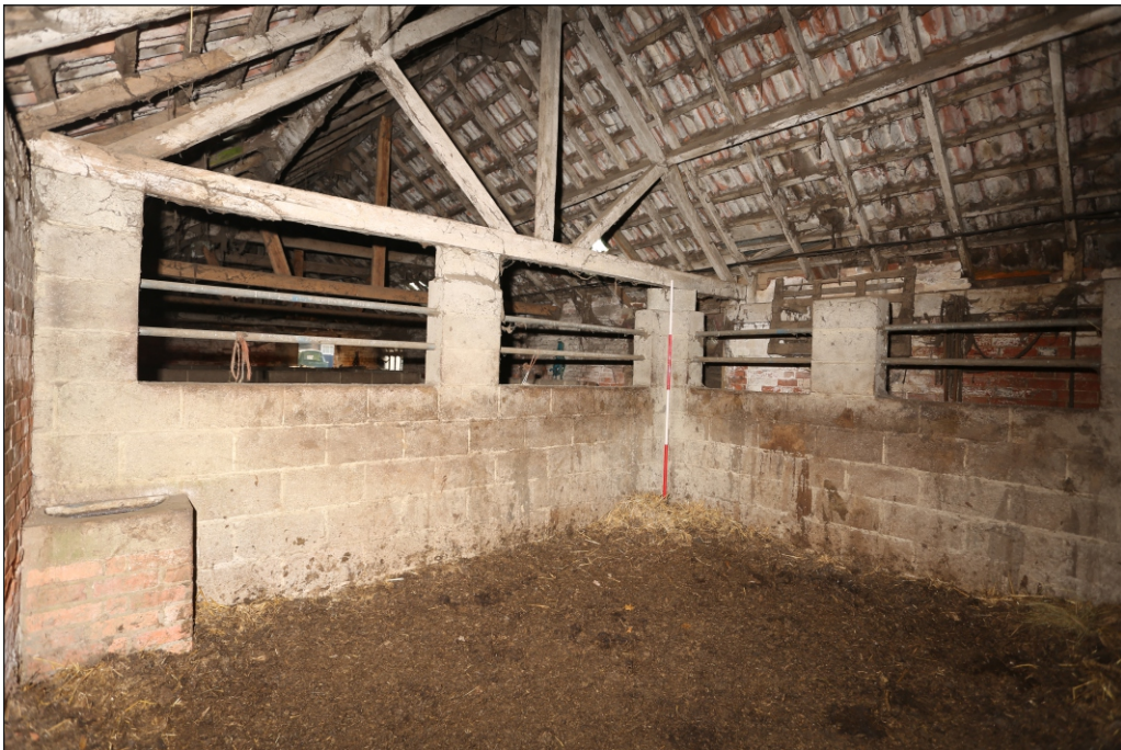
Plate 22: Building 7 north pen viewed from the north-east
