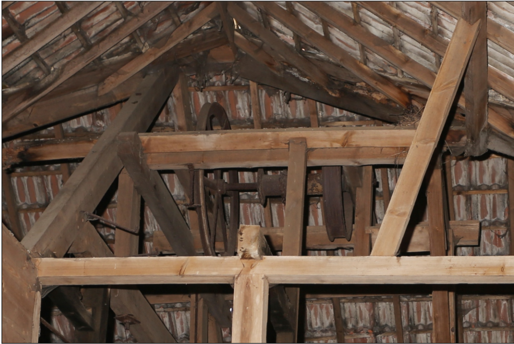
Plate 13: Building 2 wheel mechanism on the first floor viewed from the south
