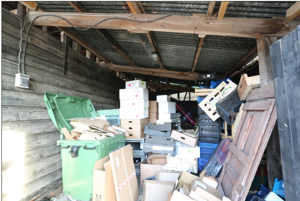
Plate 27: Building 12 viewed from the west
