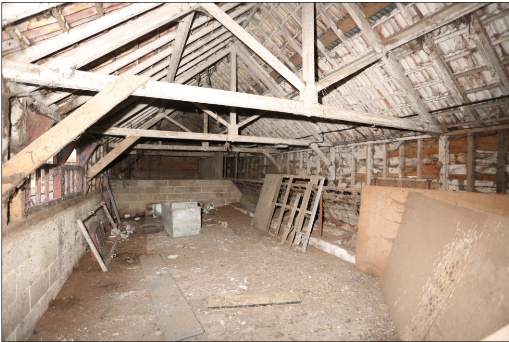
Plate 20: Building 5 ground floor viewed from north-west
