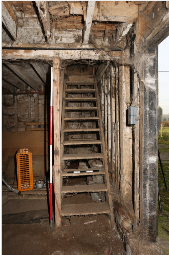
Plate 15: Building 3 staircase viewed from the east
