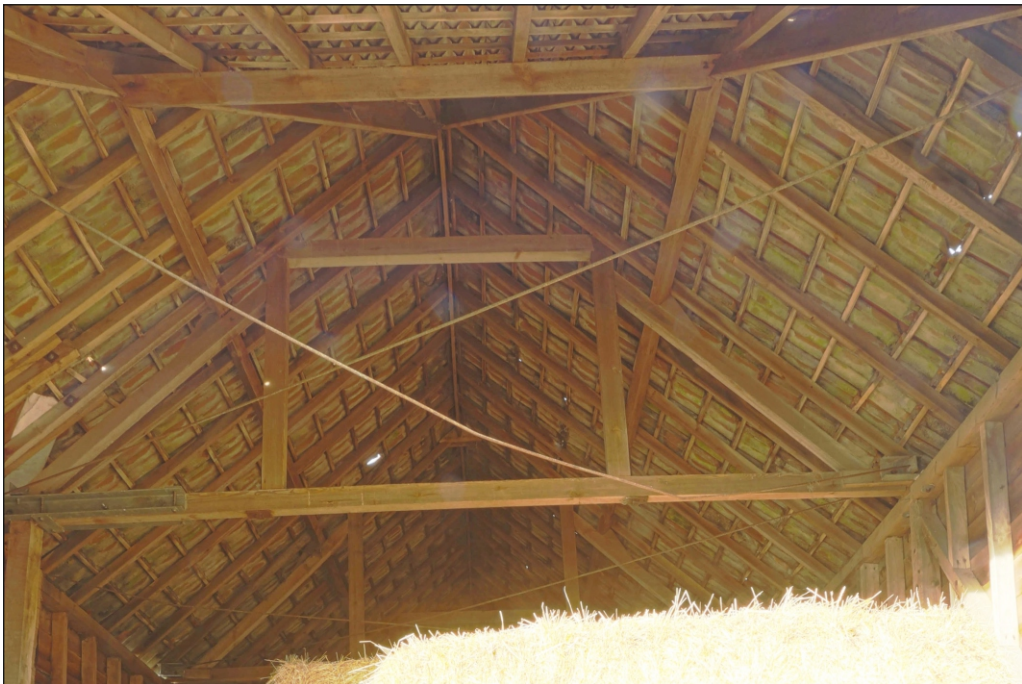
Plate 10: The roof structure within Building 1, viewed from the south
