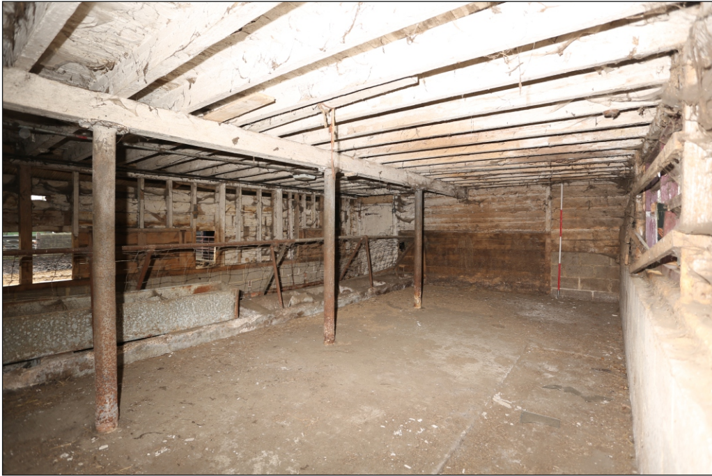
Plate 17: Building 4 ground floor viewed from the north-east
