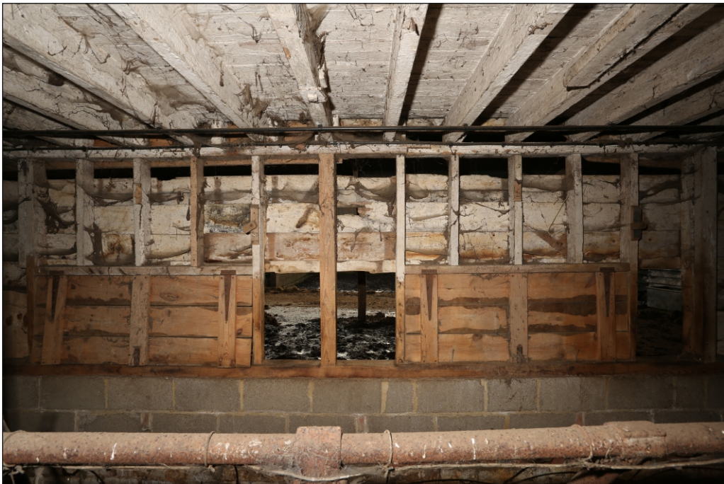
Plate 18: Building 4 inserted hatches in the south wall, viewed from the north
