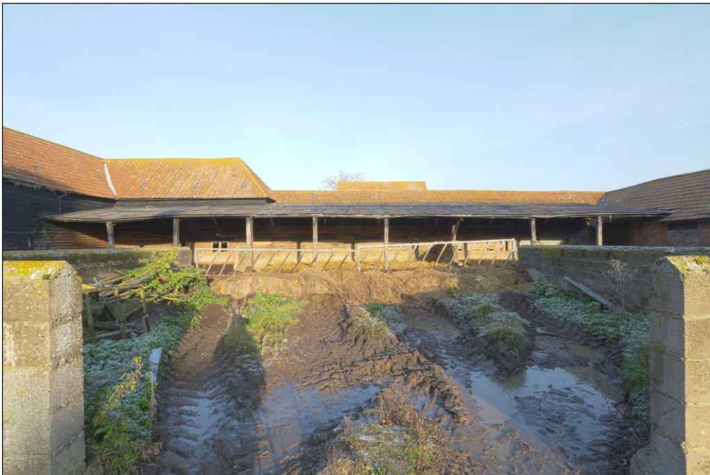
Plate 8: Redundant agricultural buildings viewed from the south showing the central yard and Building 8
