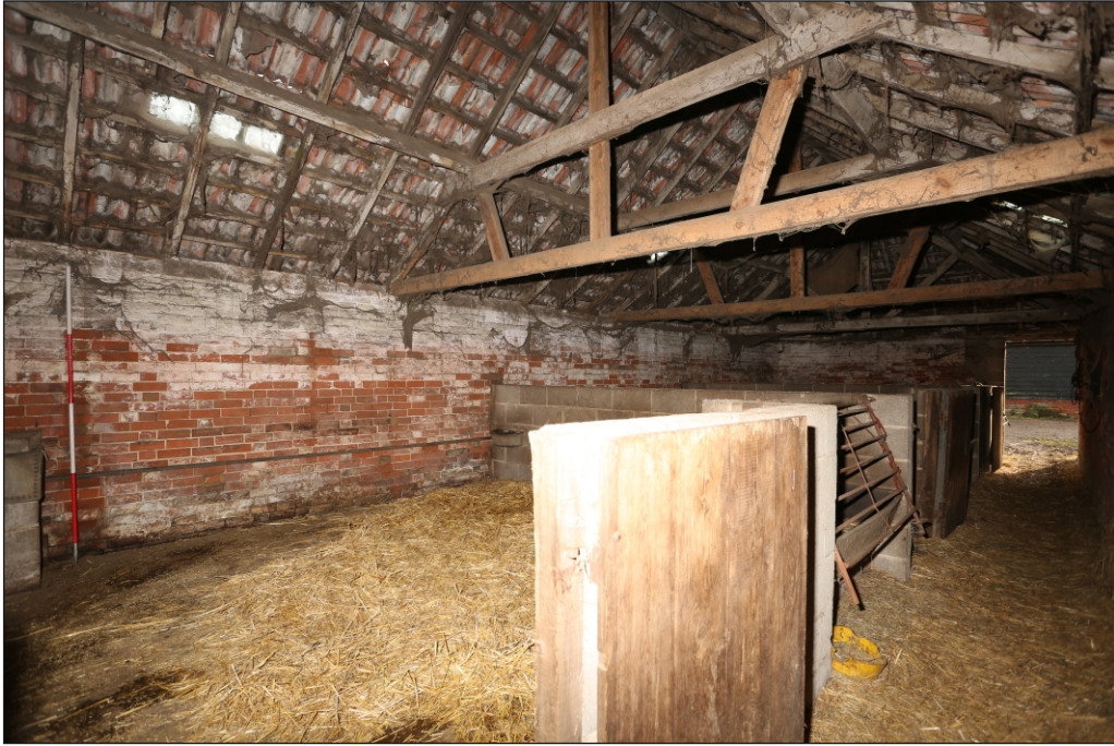
Plate 23: Building 7 pens (except the north one) viewed from the north-west
