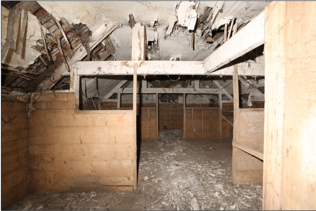
Plate 19: Building 4 first floor viewed from the west
