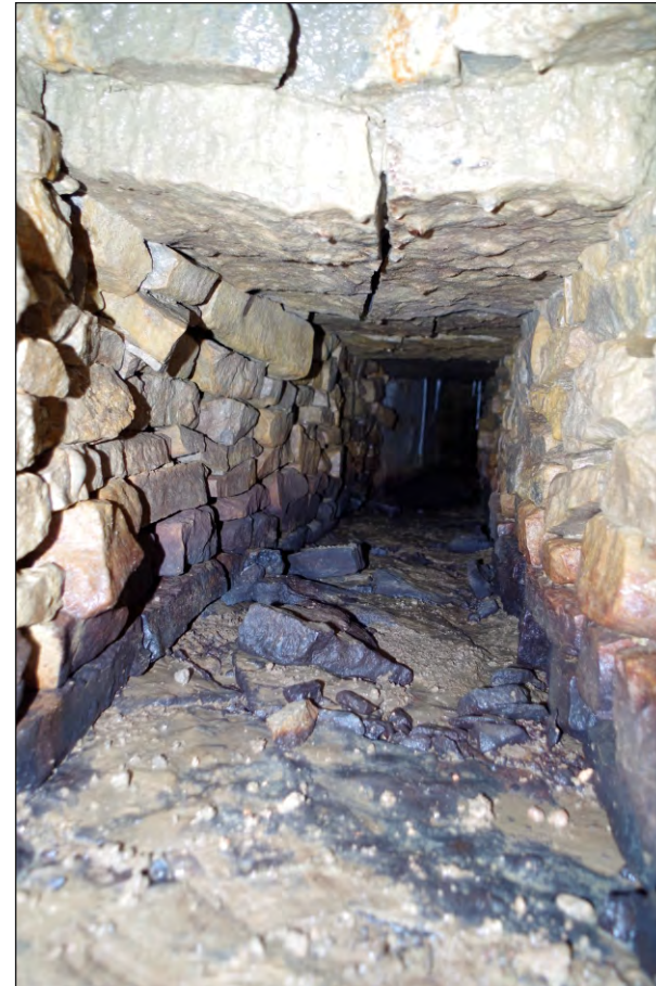
Plate 2: View north along interior of drain 002
