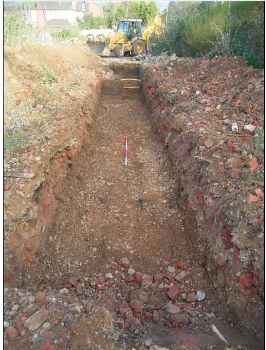
Plate 2: Trench 3 from the south-east
