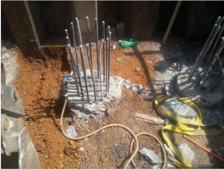
Plate 3: Partial removal of former pile
