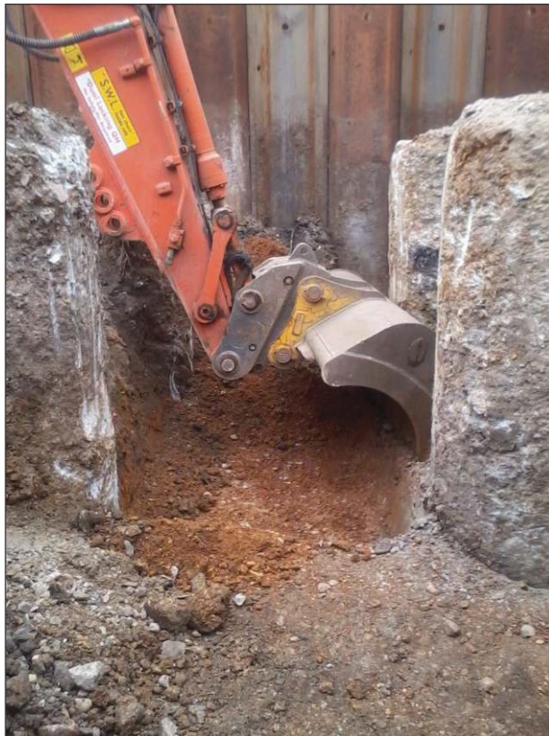
Plate 2: Ground reduction around existing piles
