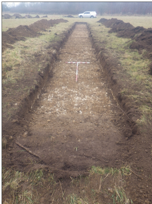
Plate 4: Trench 5 from the north east
