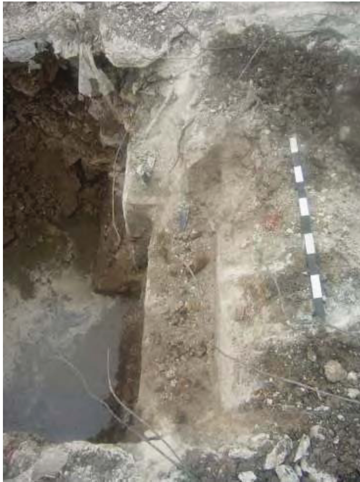
Plate 1. Trench 1 concrete haunching from the west
