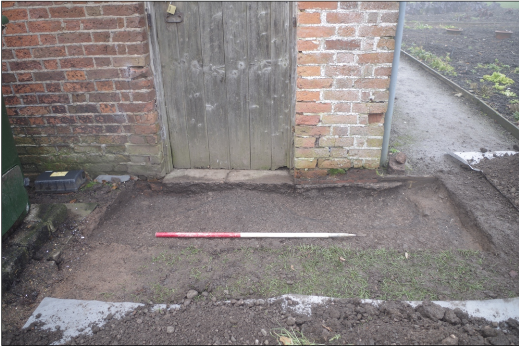
Plate 1: Trench 1, view from east
