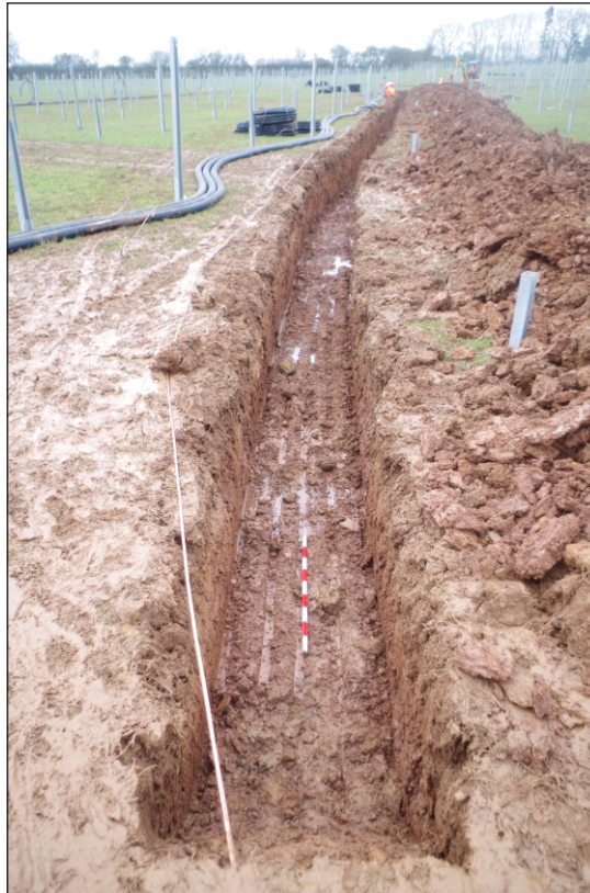
Plate 1: Overview of length of Trench 1, interior of Site, looking north-west, 1 x 1 m scale
