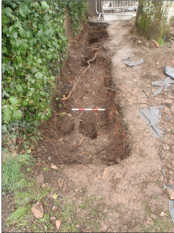
Plate 3: Trench 2 showing heavy root disturbance, looking east, 0.50m scale
