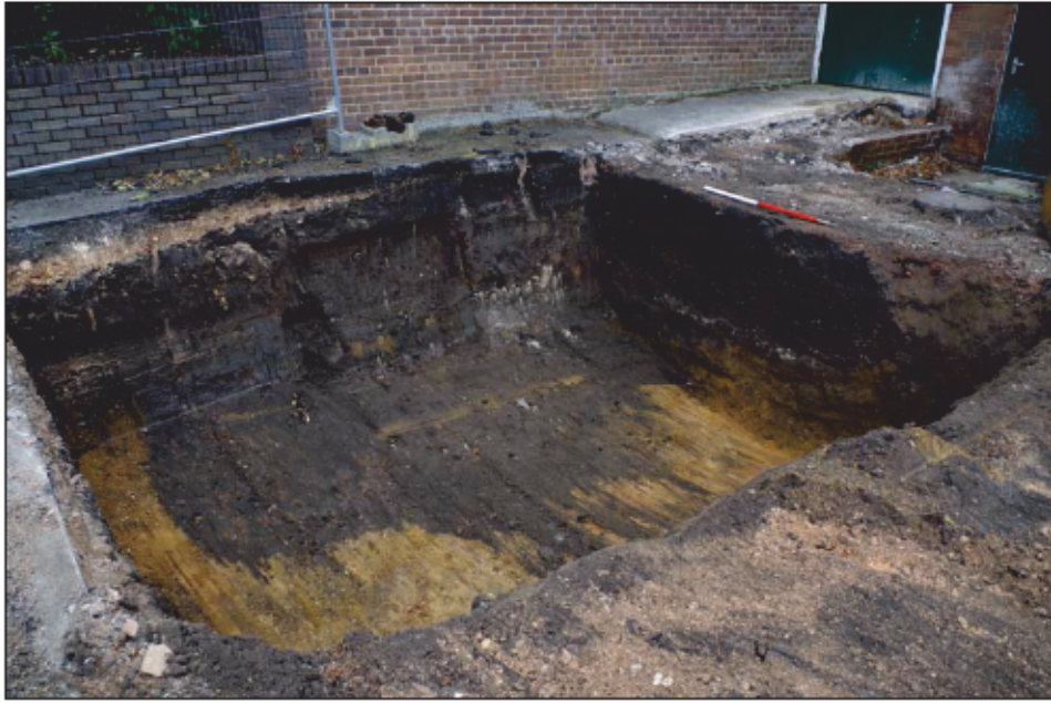
Plate 3: General shot of SMR 1: Area 1 following excavation. Photograph facing east
