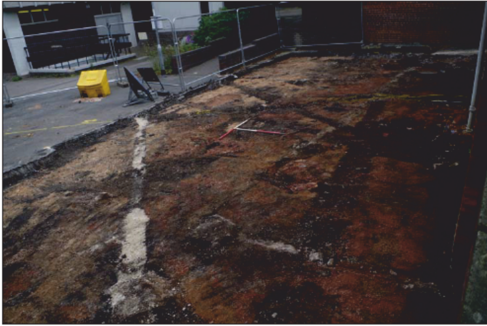
Plate 1: General shot of SMR 1 following machine strip, showing extent of services
