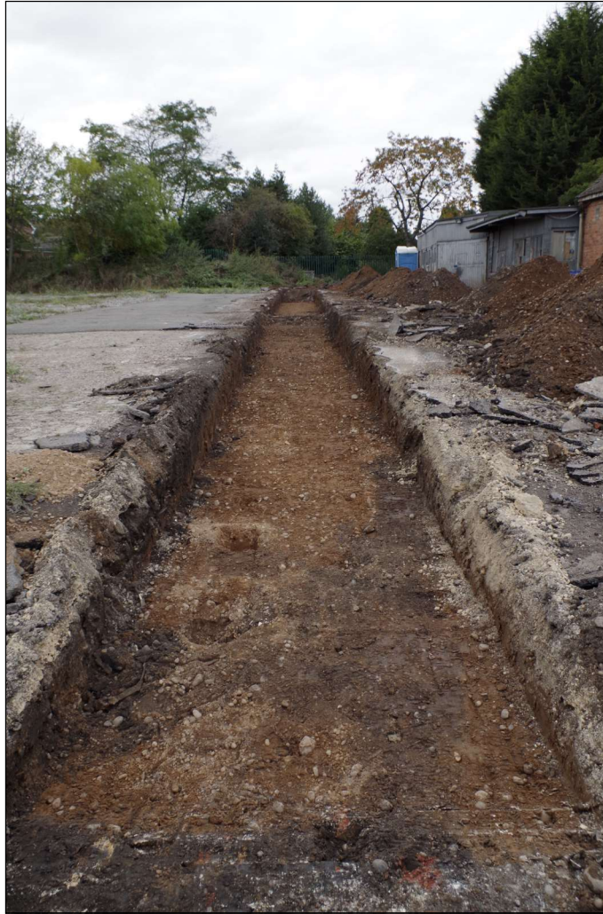
Plate 5: Trench 3, general shot looking west
