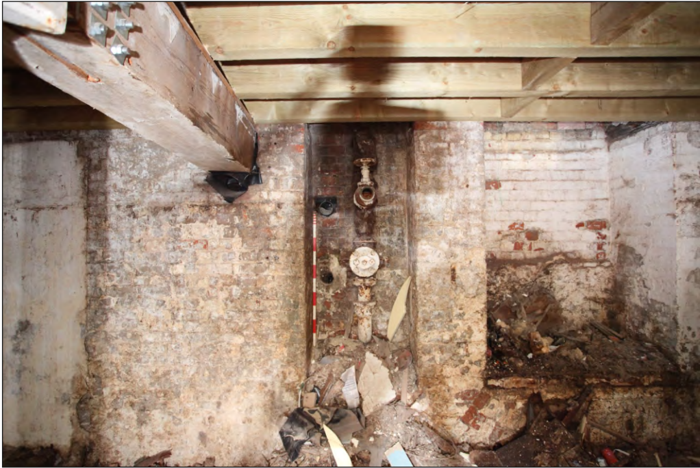
Plate 7: Basement of Huller House, old pipework against eastern elevation, 1m scale
