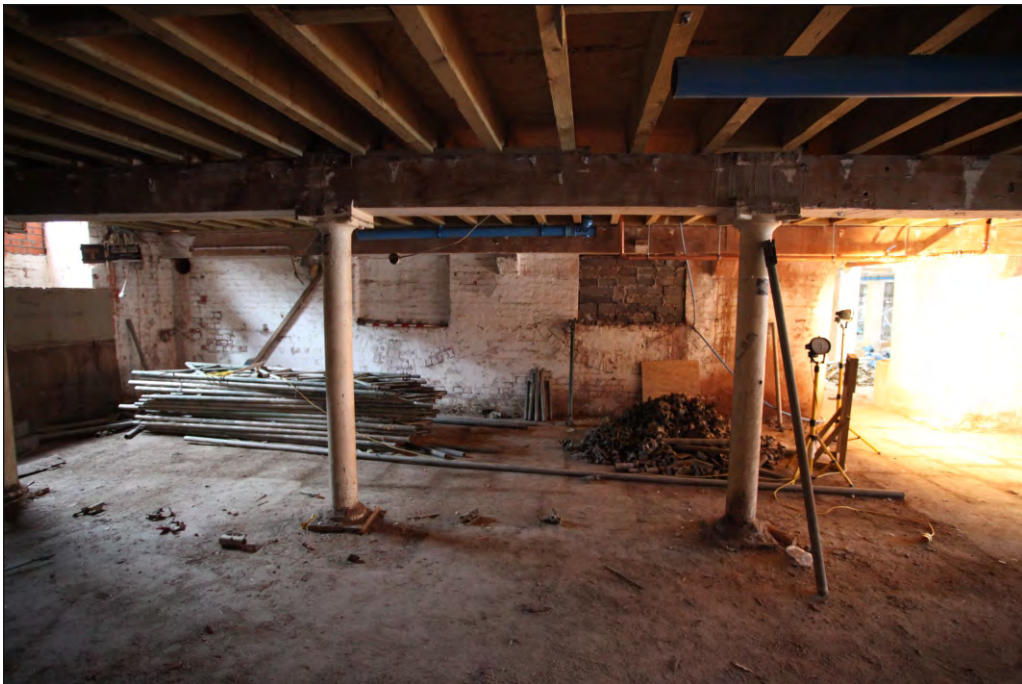
Plate 6: Basement of Huller House, relieving arches in southern elevation, 1m scale
