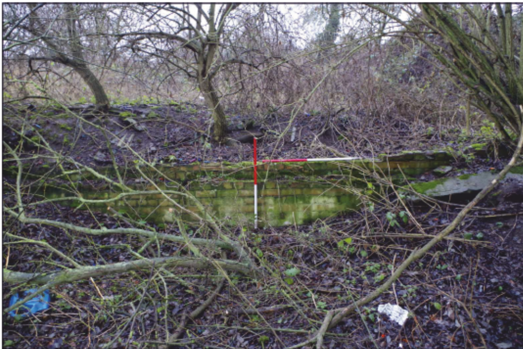
Plate 6: Surviving wall in Field 31, looking east
