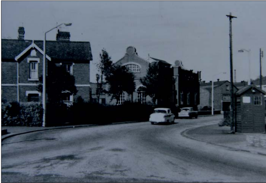
Plate 1: General view of the Site from the south-east of Green Street, c. 1960s, showing the former engineer's house and extant pumping station
