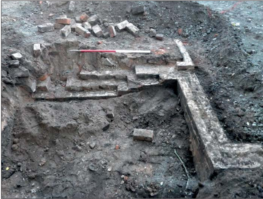
Plate 3: Brick foundation walls 104, 105, 106 and 107 at the western end of the trench, looking north-east
