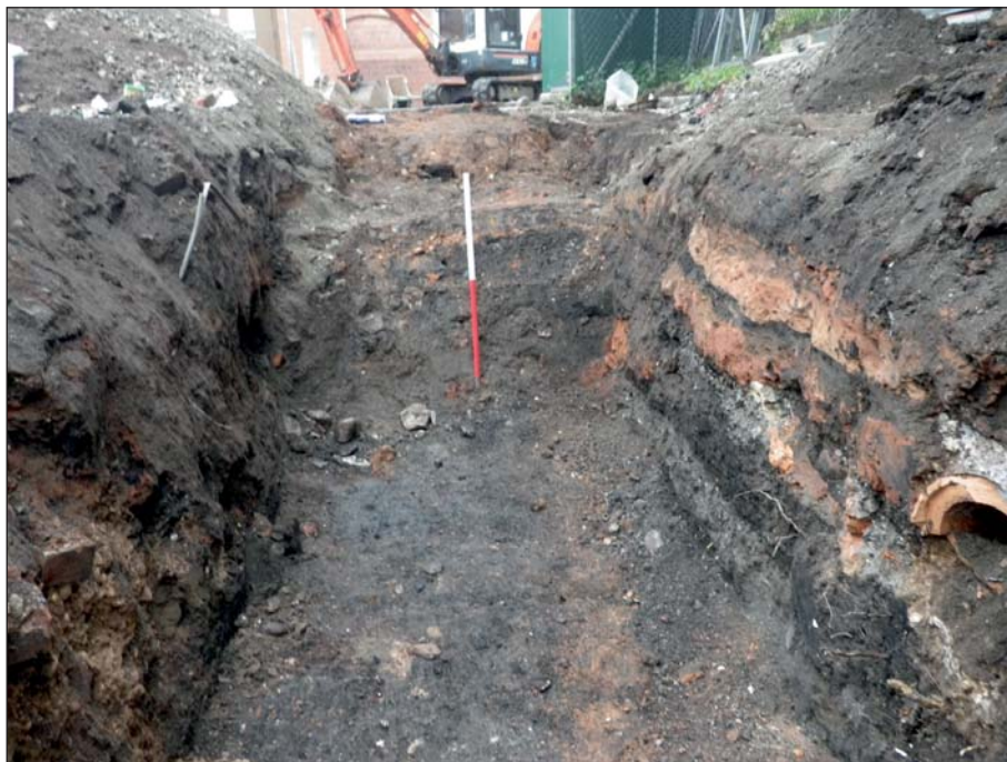
Plate 6: Representative section at the centre of the trench, looking east
