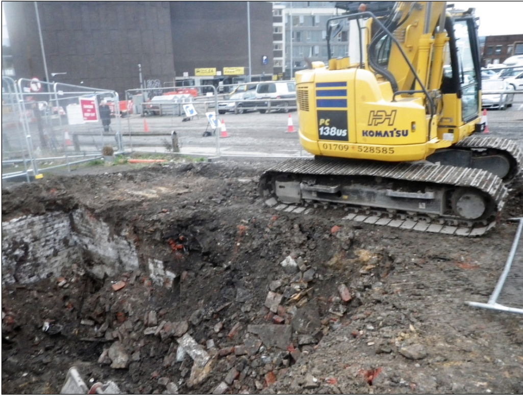
Plate 11: Cellar 2080, looking south-west
