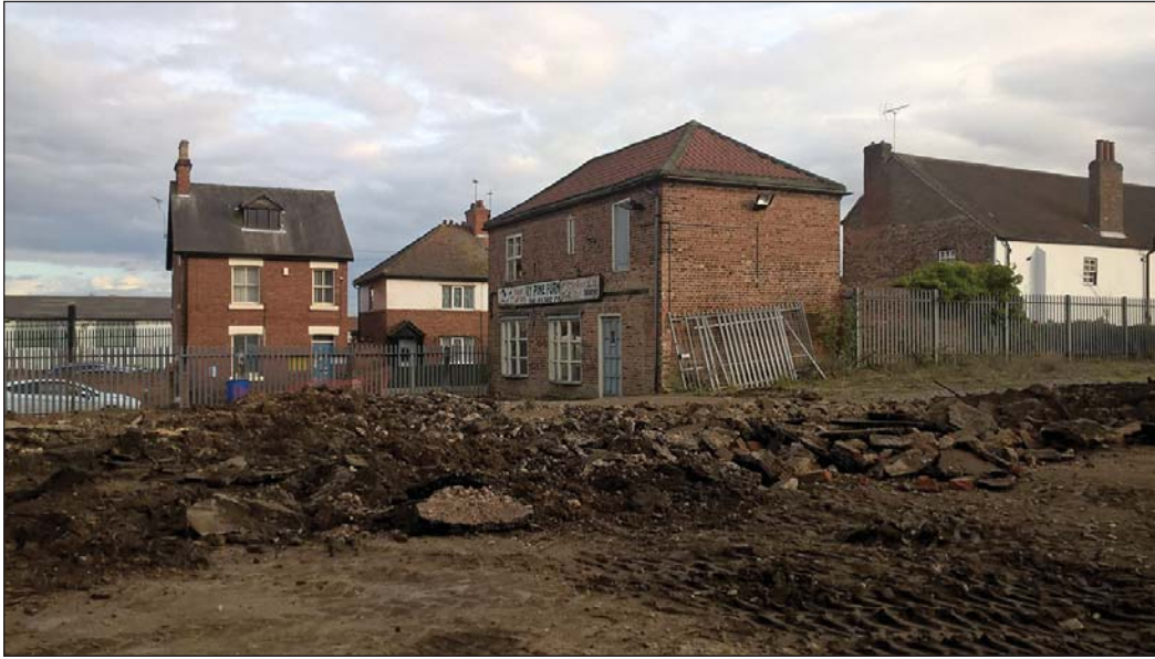
Plate 1: General shot of site during the machine strip. Shot facing east
