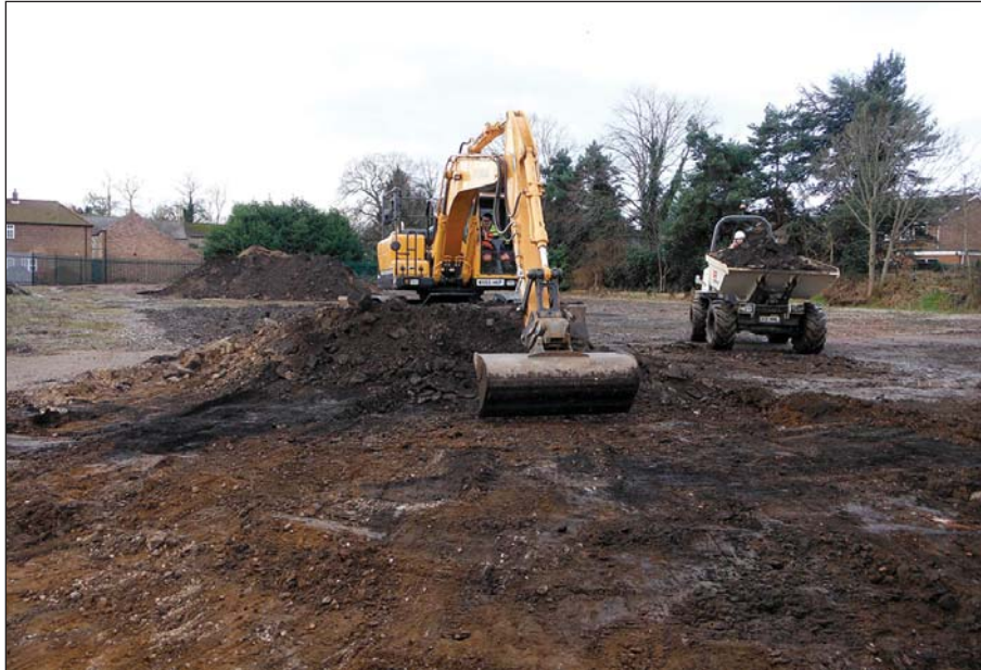
Plate 3: Detail shot of twentieth century disturbance being stripped
