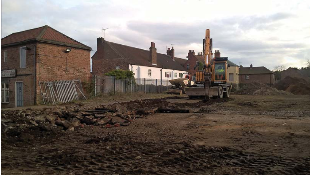
Plate 2: General shot of site during the machine strip. Shot facing southeast
