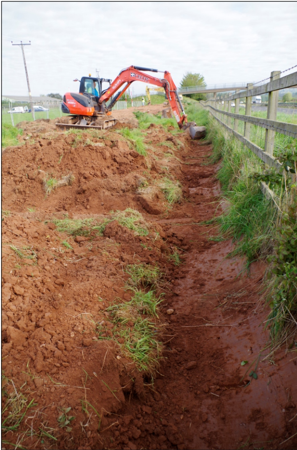
Plate 1: Excavation of north-south drainage ditch viewed from the south
