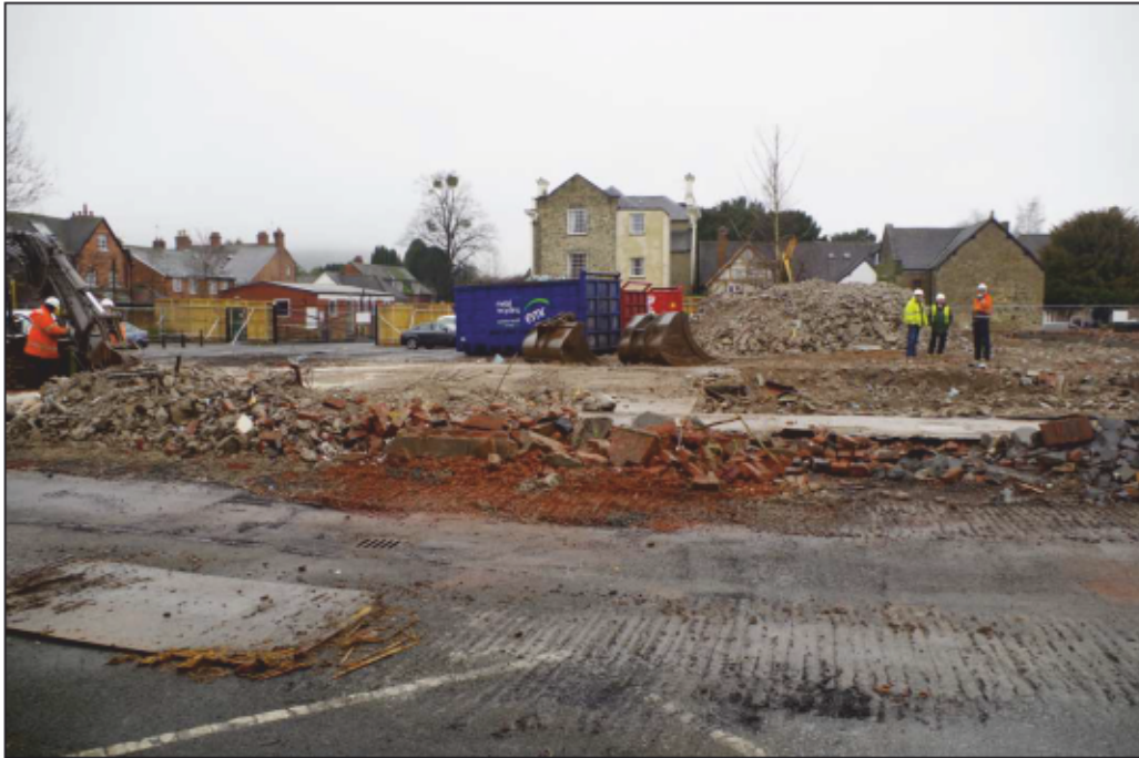
Plate 1: General shot of site following demolition of the twentieth century buildings
