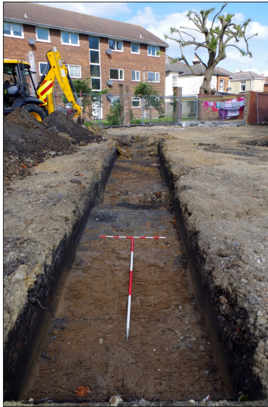
Plate 7: Trench 2, viewed from the South. Scales at 1 m and 2 m
