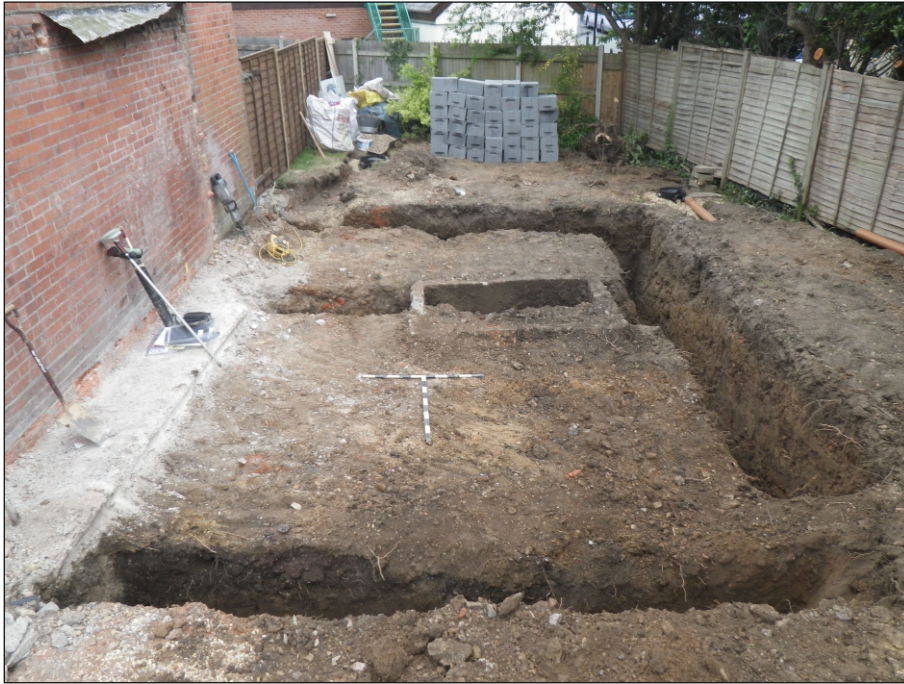
Plate 1: Site looking west
