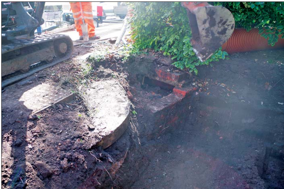
Plate 6: Inspection chambers 14003 (far, brick) and 14004 (near, concrete)
