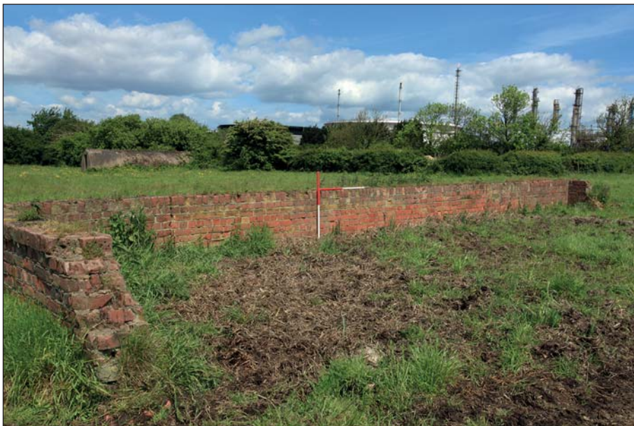
Plate 2: View of northern wall of Fuel Compound
