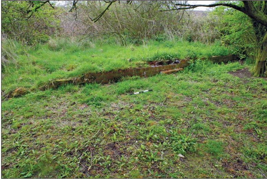
Plate 21: View of red-brick foundations of western wall of B3
