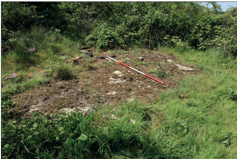
Plate 10: View of the concrete base of A2
