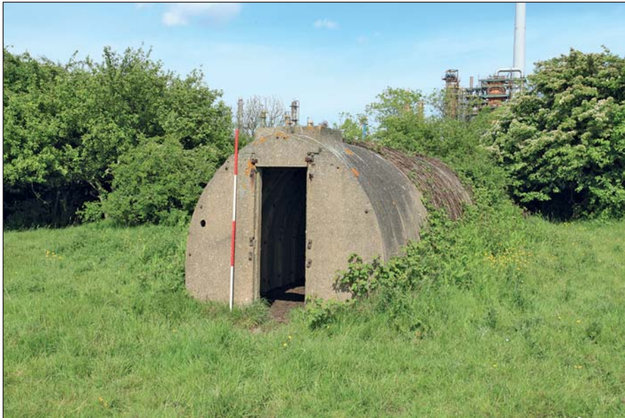
Plate 36: View of Air Raid Shelter 3, with truncated escape hatch projecting from the roof
