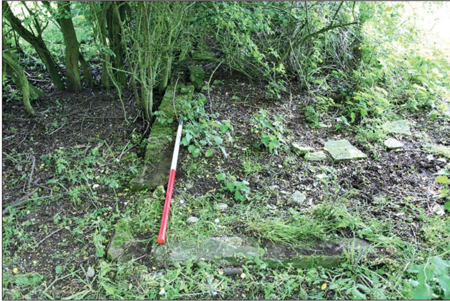
Plate 25: View of the south-eastern corner of foundations of C1
