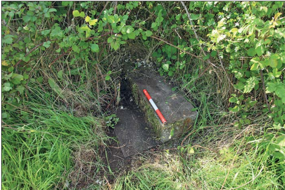
Plate 20: View of concrete step entrance to B2
