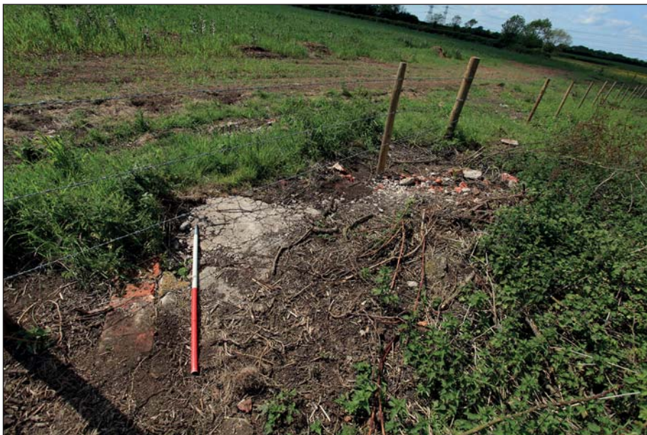
Plate 16: View of red-brick foundations of south-western corner and fragmented concrete base of B1
