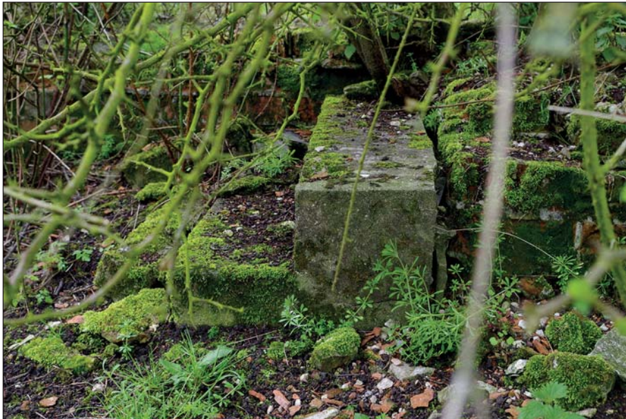
Plate 22: Concrete step abutting the northern elevation of B3
