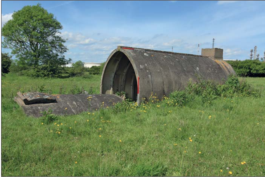
Plate 33: View of Air Raid Shelter 2 showing the collapsed western section
