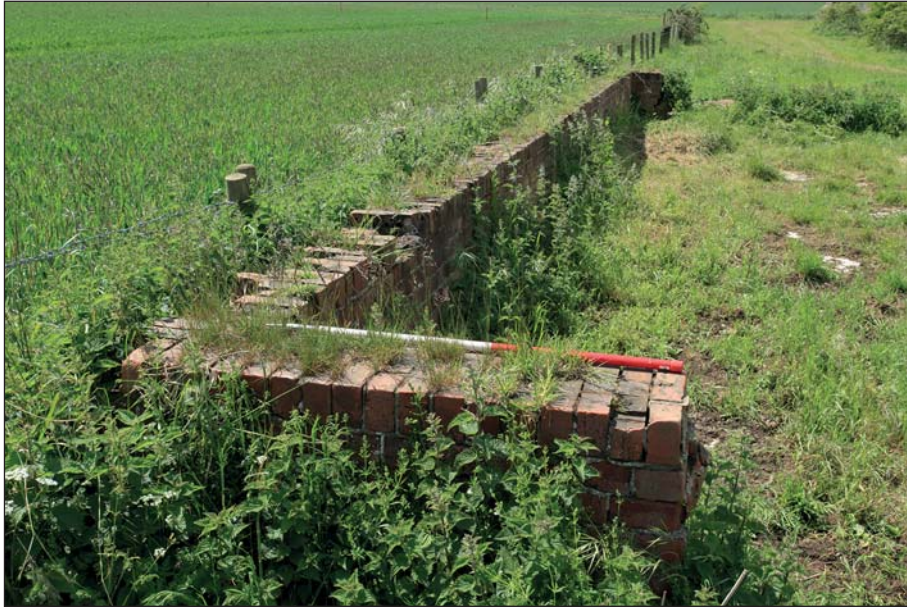
Plate 3: View of south-eastern corner of Fuel Compound
