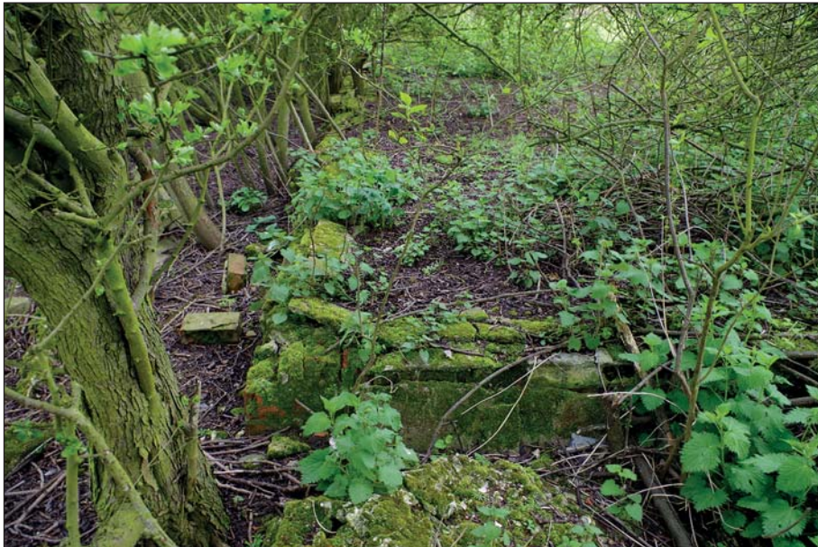
Plate 28: View of foundations of northern elevation of C2
