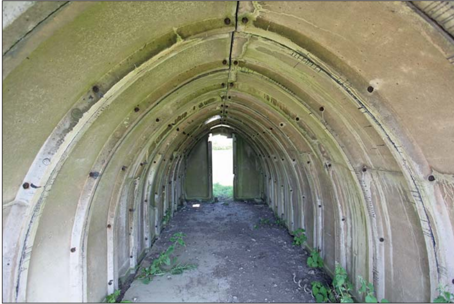
Plate 35: View of interior of Air Raid Shelter 2
