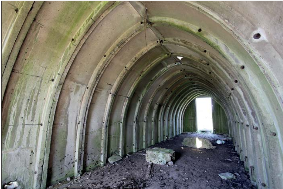
Plate 32: View of interior of Air Raid Shelter 1, showing the joins of the pre-cast concrete arches, with the north-eastern doorway beyond
