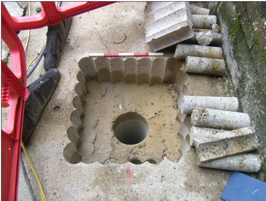
Plate 4: Test Pit 6 from the north (scale 0.50 m)
