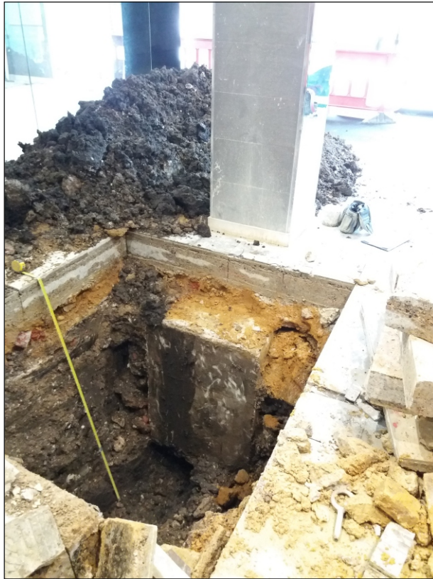
Plate 3: 1960s concrete pillar base impacting buried remains in Test Pit 3 (photo from south-east)
