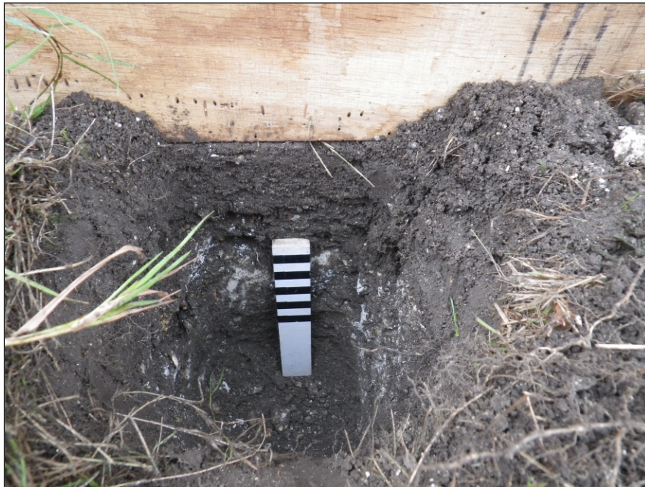
Plate 5: Typical example of the shallow holes excavated next to the replacement fence panels for supporting posts
