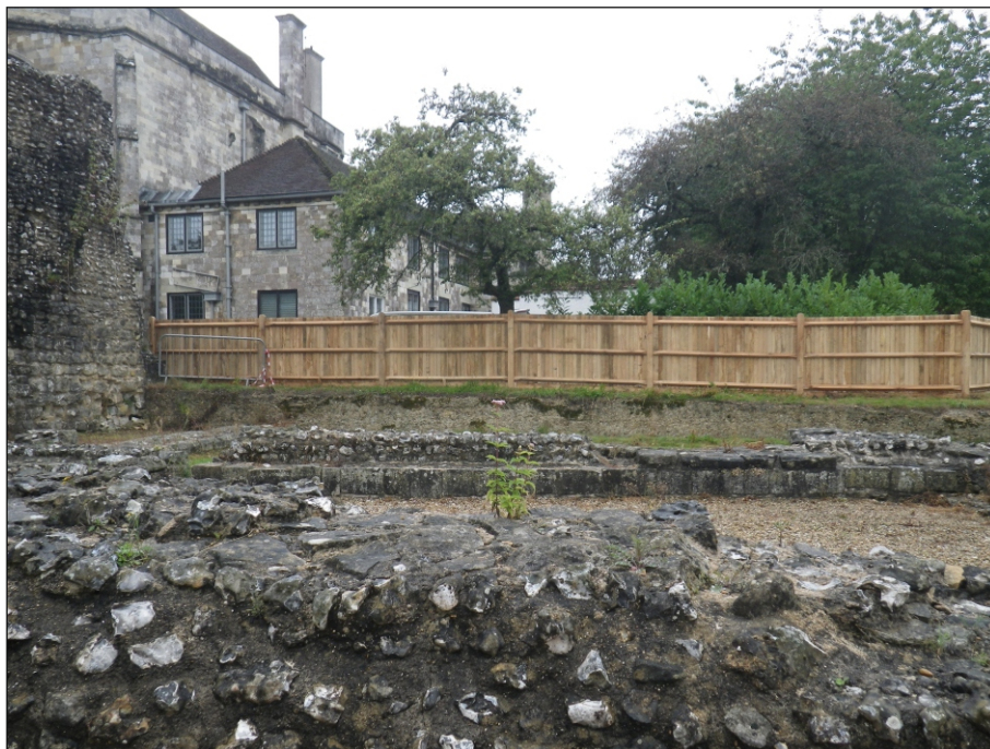
Plate 6: The replacement fence completed, viewed from the east
