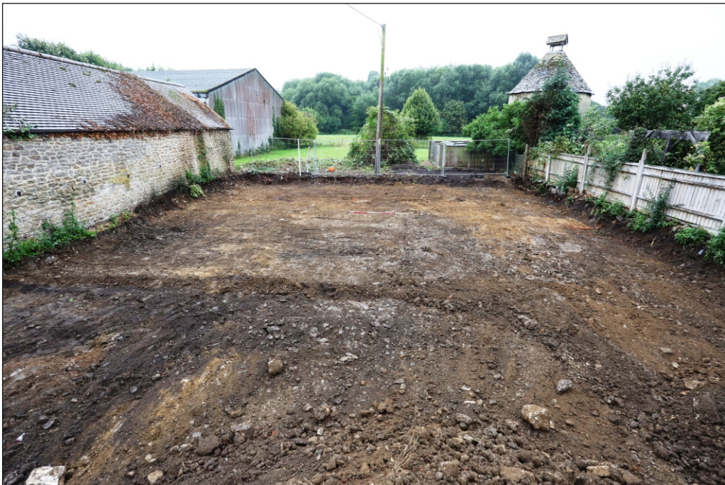
Plate 4: Area 1b after site stripping looking west
