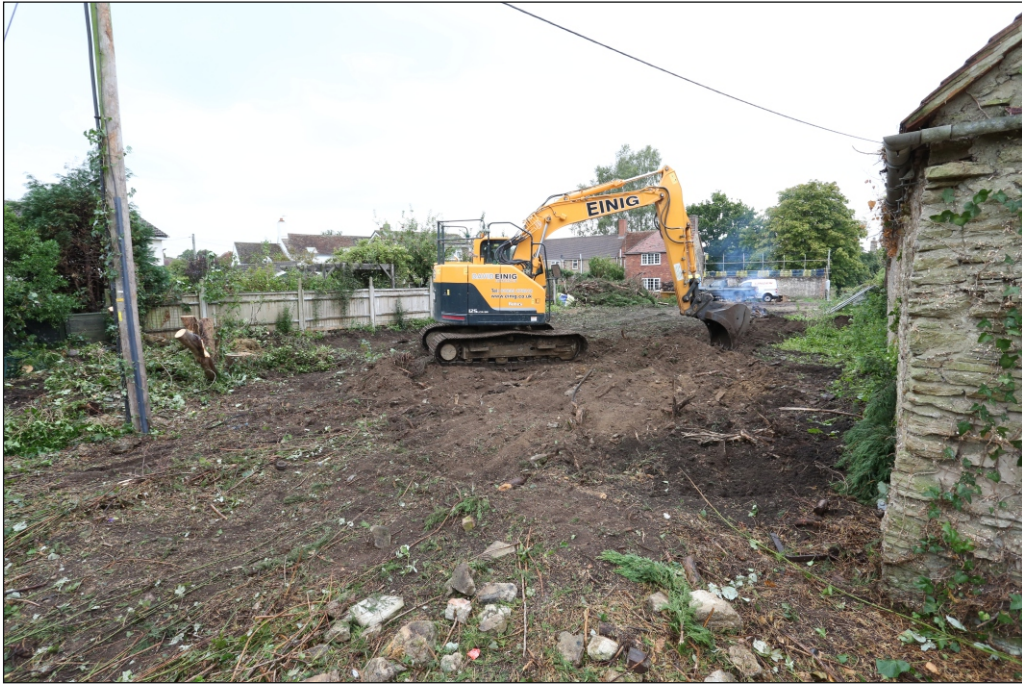
Plate 3: Area 1b removal of west tree boundary looking east
