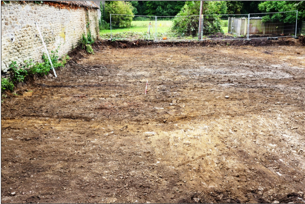
Plate 5: Area 1b remains of possible stone wall looking west
