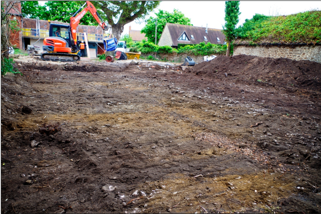
Plate 1: Area 1a topsoil stripping looking south-east
