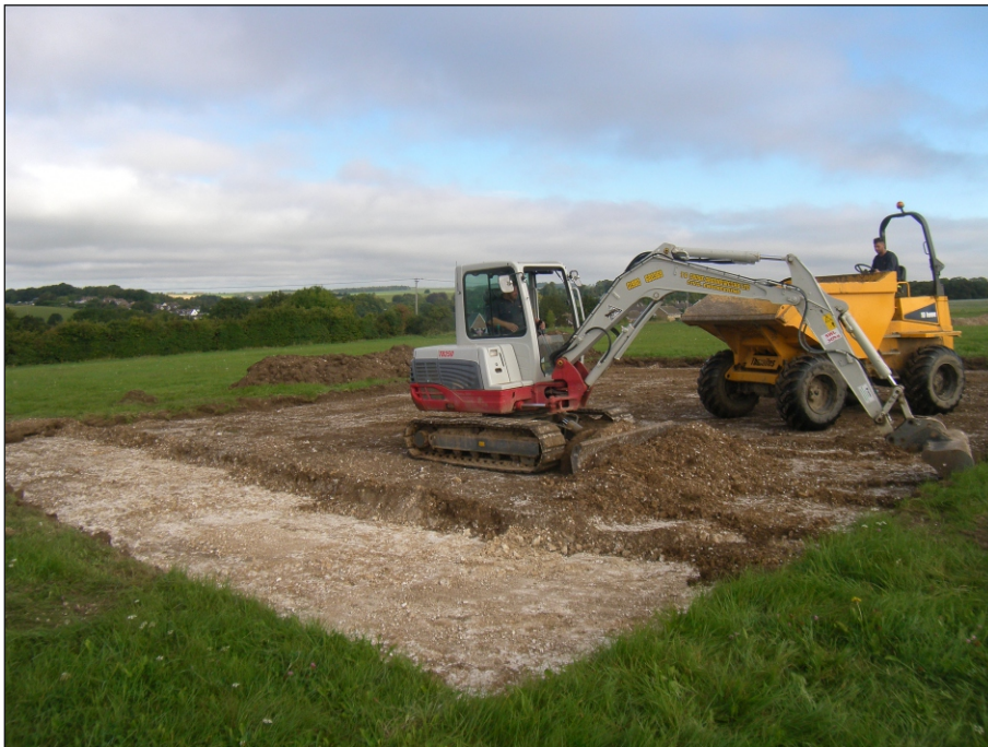
Plate 8: Topsoil stripping of Trench 13
