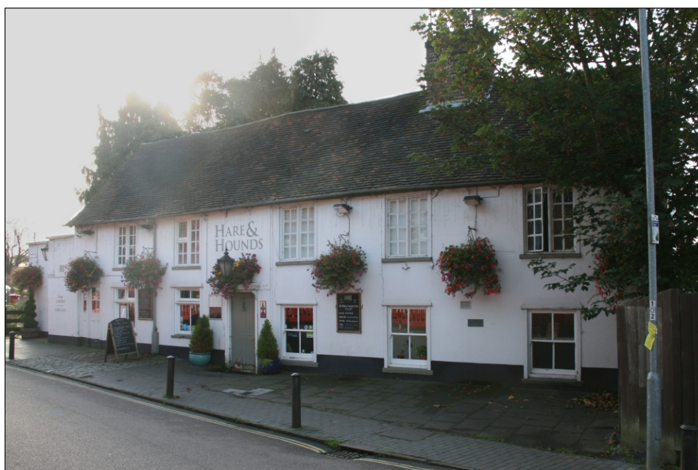
Plate 2: North face of the building, looking south-east
