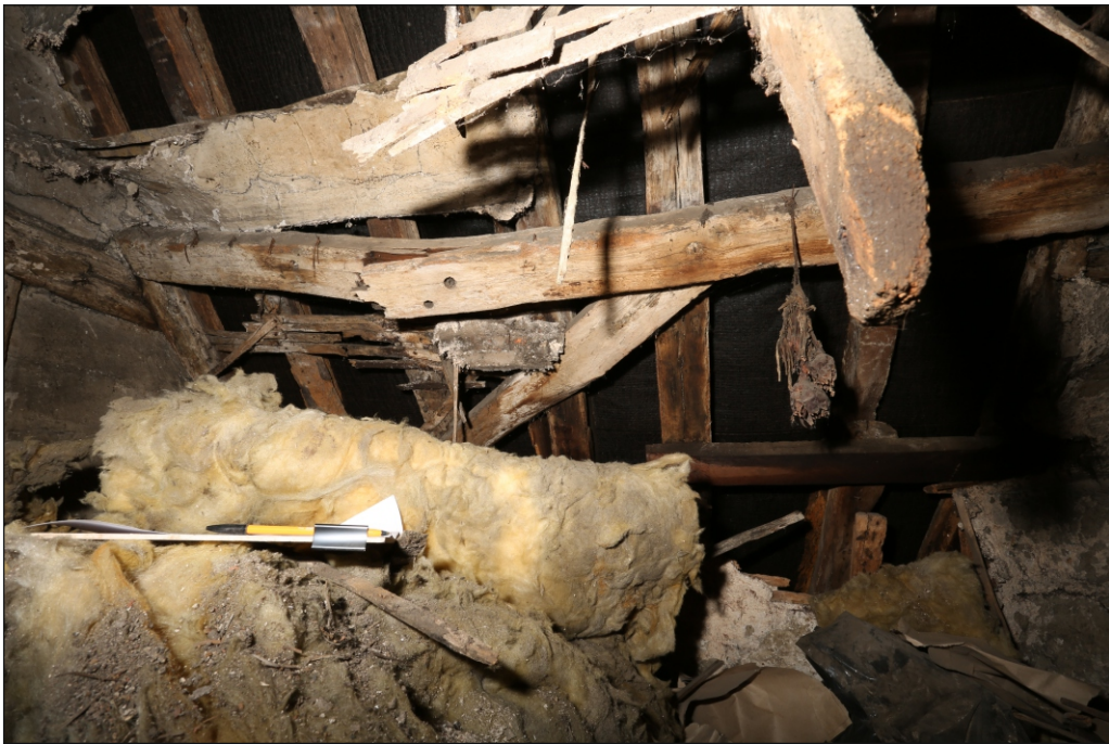
Plate 8: North side of Bay 1 roof, looking north-west
