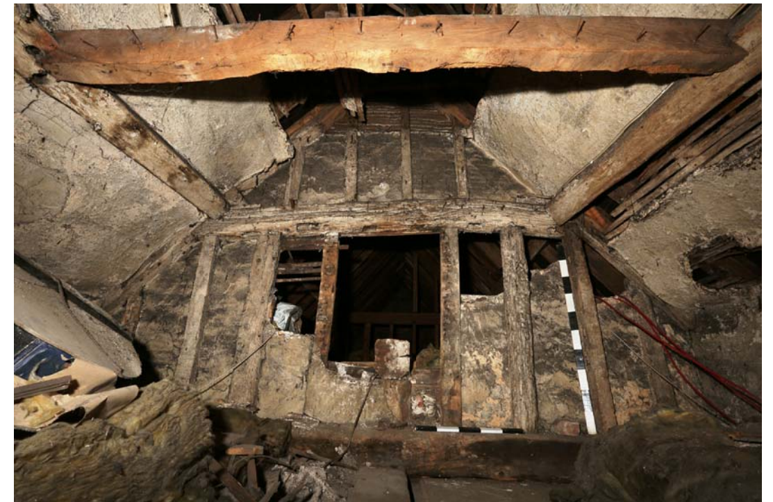
Photograph of Truss 4, viewed from the west.
