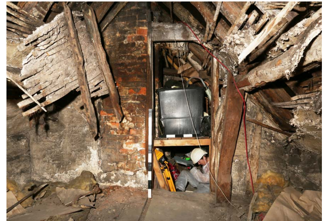
Photograph of Truss 2, viewed from the west, showing iron bracket on purlin and inserted post.
