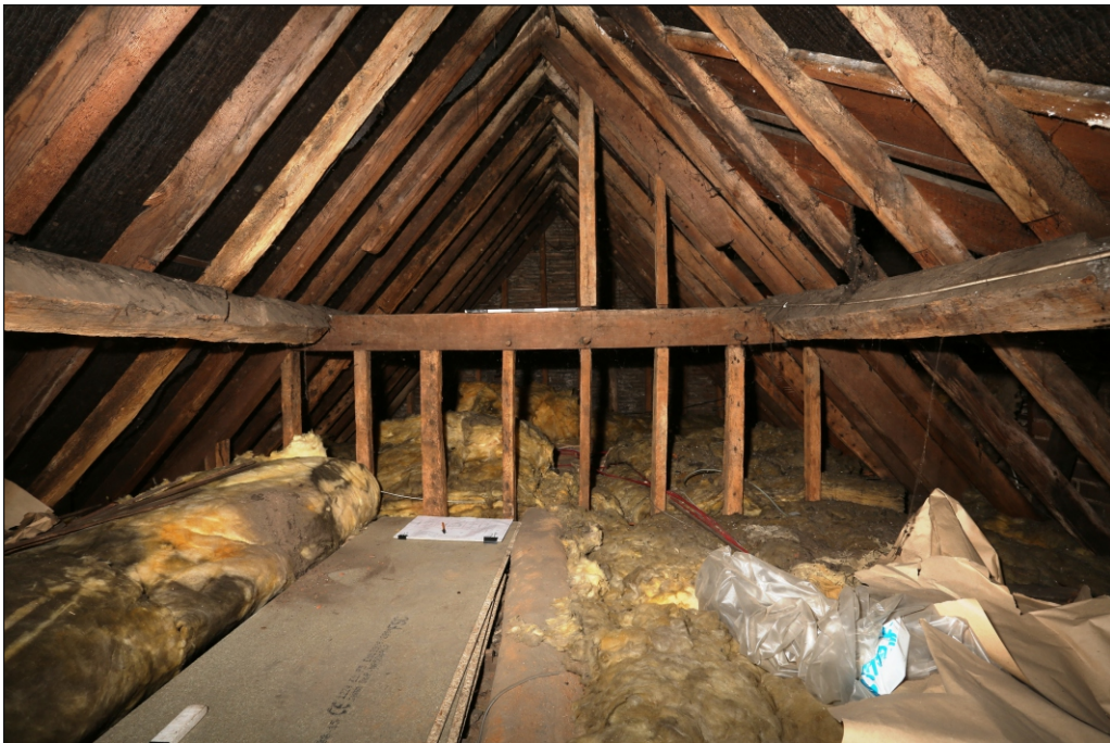
Plate 14: Truss 5 between bays 4 and 5, looking east
