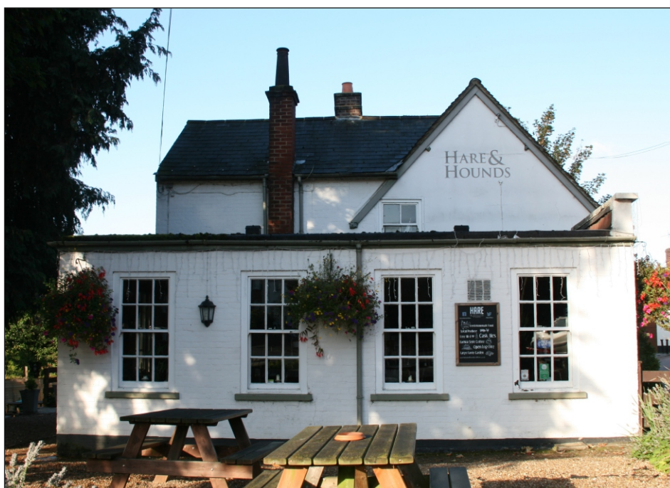
Plate 1: East face of the building, looking west
