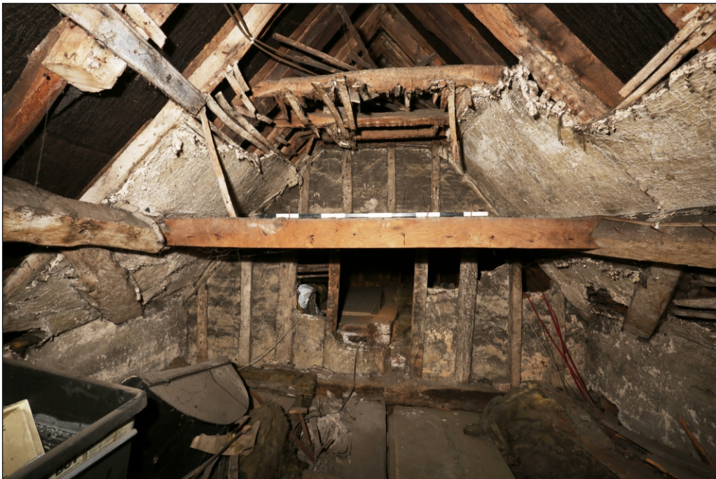
Plate 10: West face of Truss 4 in Bay 3, looking east
