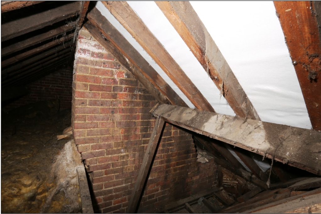
Plate 17: 19th century chimney between bays 5 and 6, looking south-west
