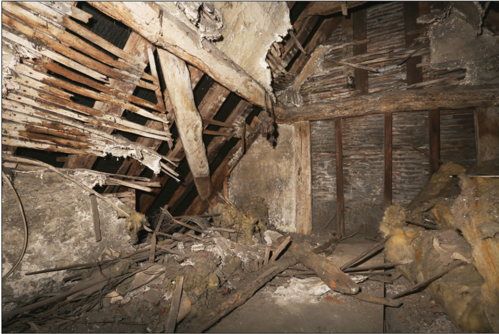
Plate 7: Truss 1 in Bay 1, looking west
