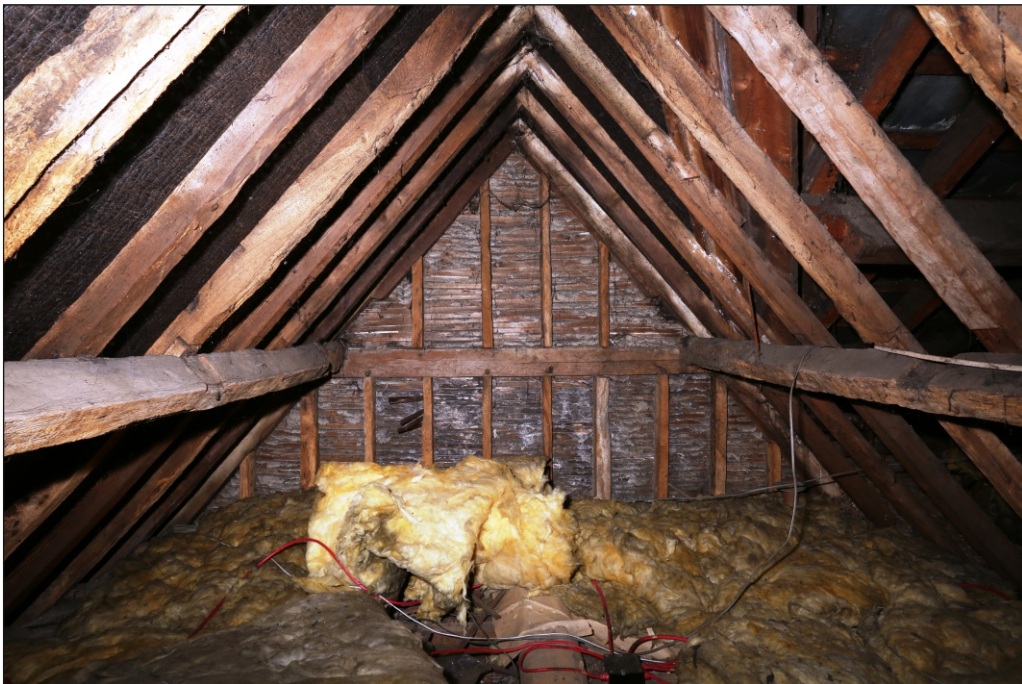
Plate 16: East gable end of building in Bay 5, looking east
