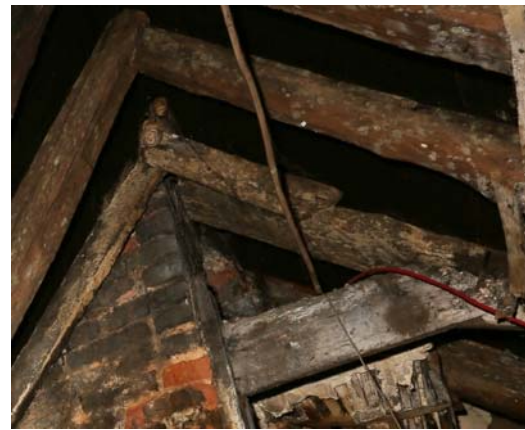
Photograph of detail of junction of principal rafters at roof apex
