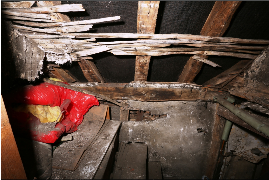
Plate 3: Staircase and south wall of Bay 2, looking south
