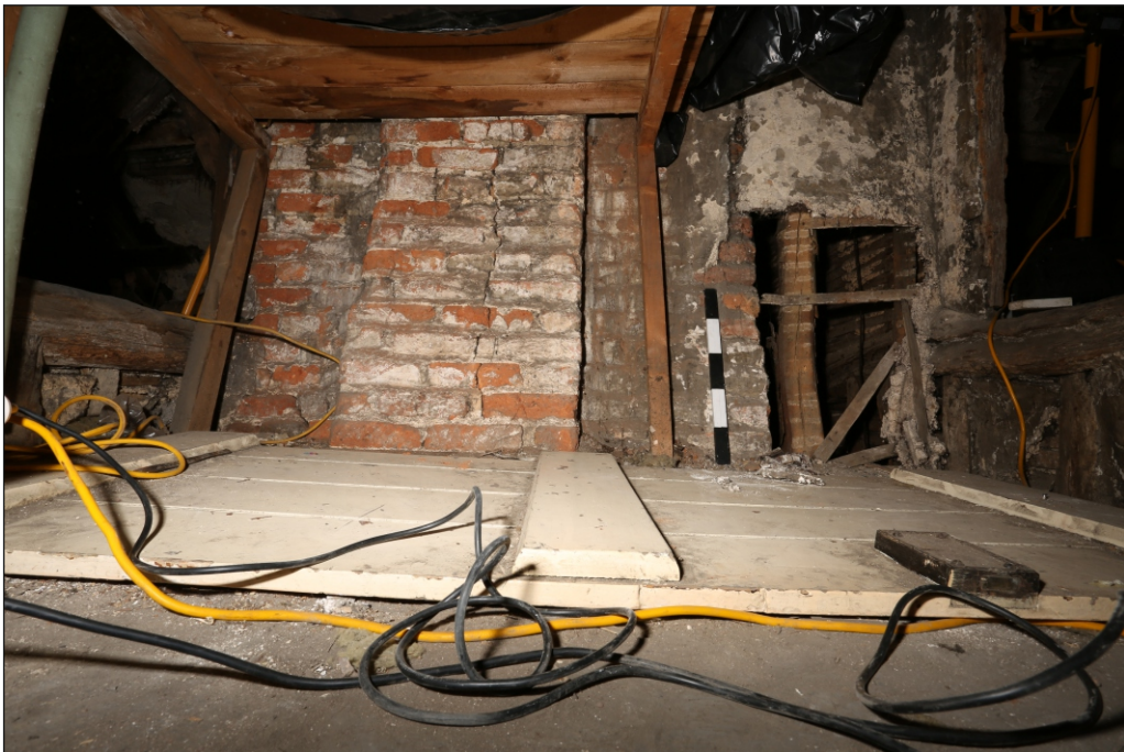
Plate 4: Chimney and void to the east side in Bay 2, looking north
