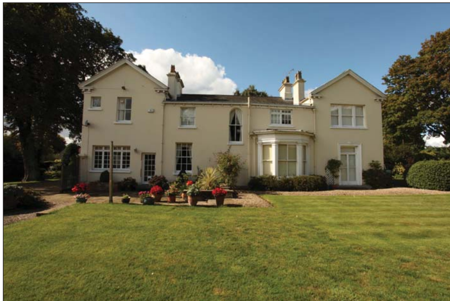
Plate 10: East elevation facing onto the rear garden
