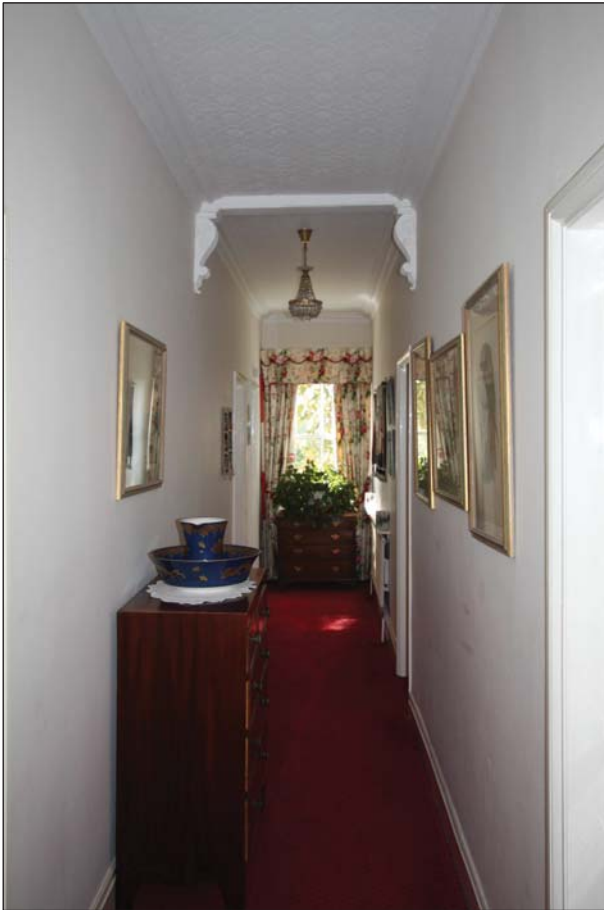
Plate 47: Corridor F1 looking south with consoles supporting a lintel
