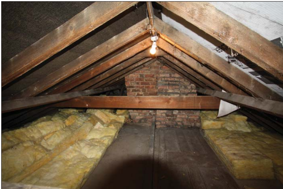
Plate 68: Loft area showing brick chimney stack
