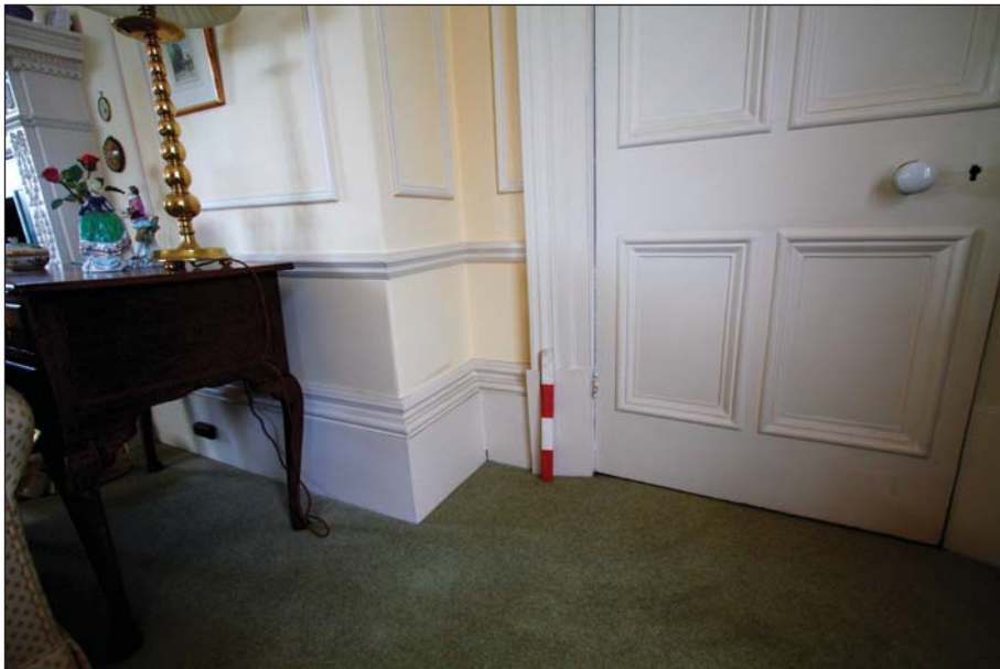
Plate 30: Detail of skirting board, dado rail and panelled door within G3
