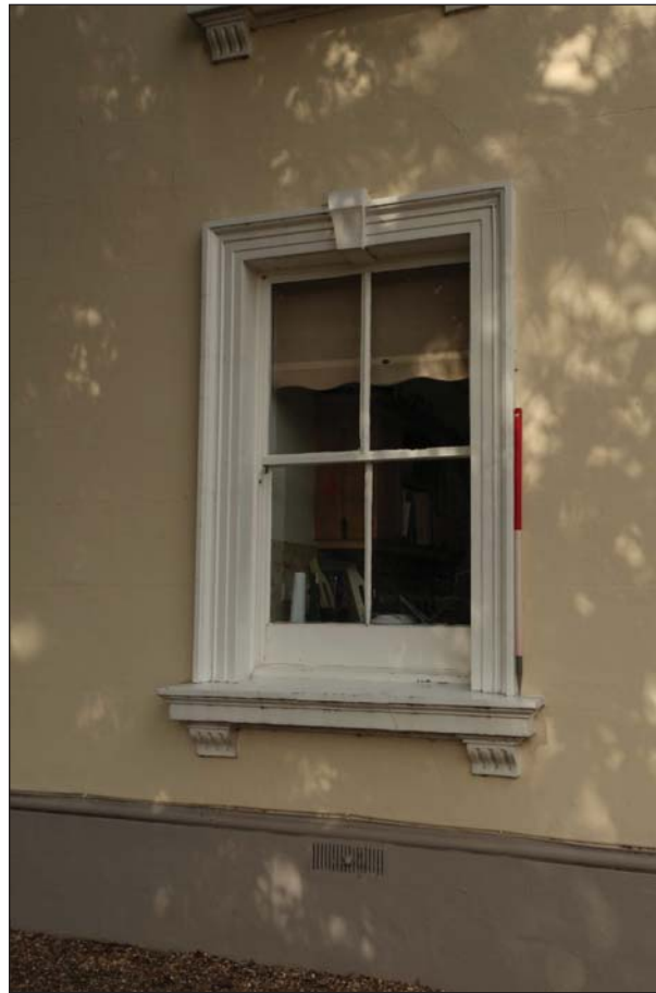
Plate 17: Detail of window opening within the south elevation
