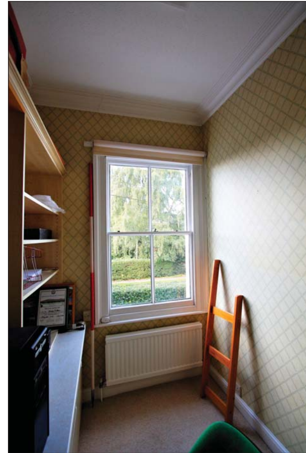
Plate 54: Detail of sash window within F6
