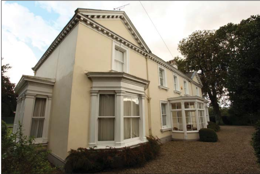
Plate 3: Northernmost bay of the west elevation viewed from the north-west
