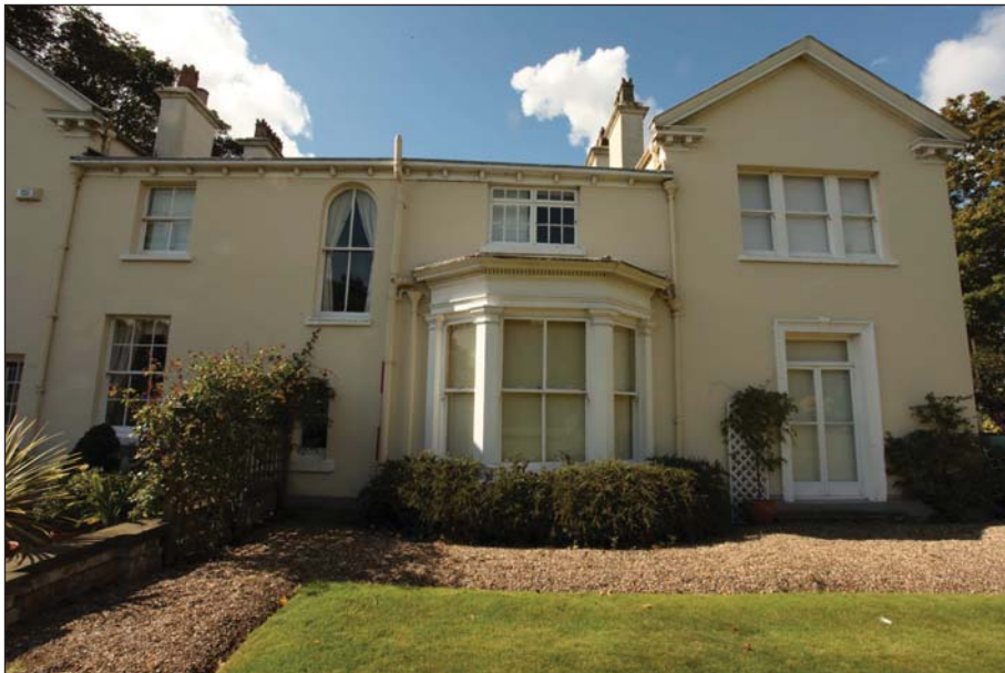
Plate 12: Central area and northernmost bay of the east elevation
