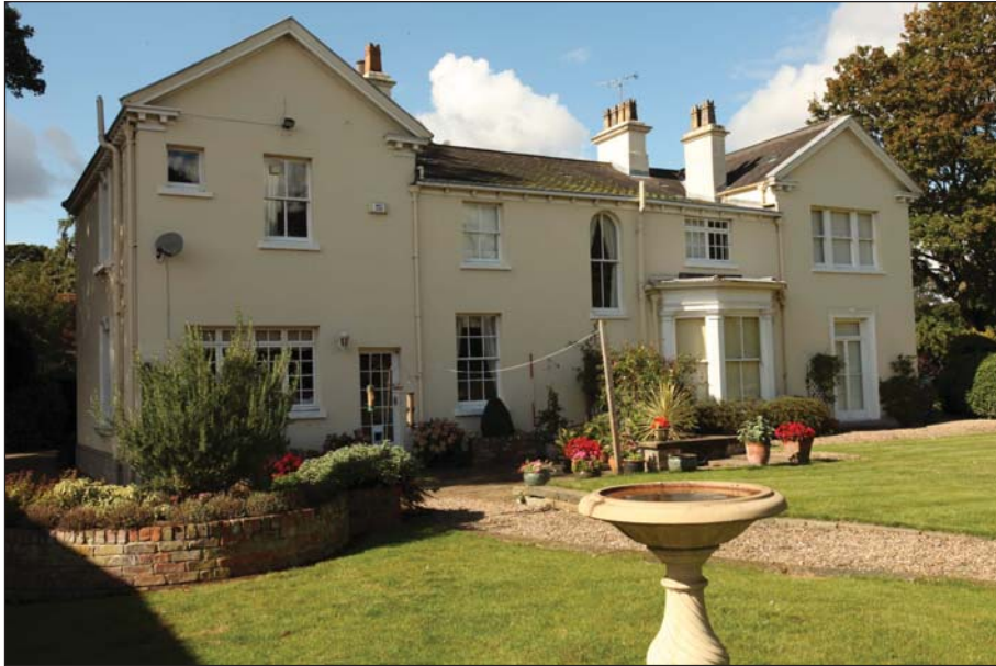
Plate 11: East elevation viewed from the south-east
