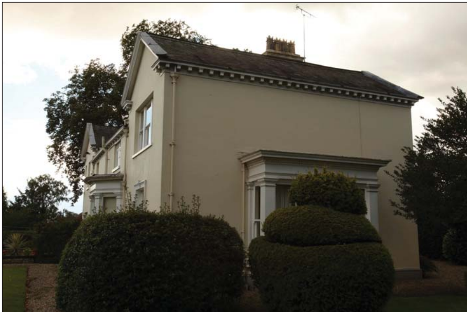
Plate 14: General view of the north elevation
