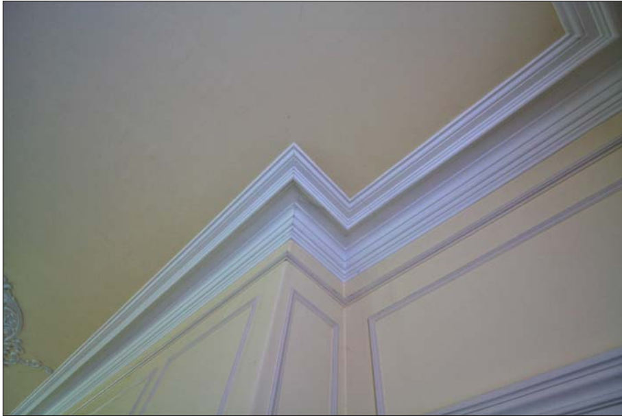
Plate 29: Detail of moulded cornice along the south wall and chimney breast of G3
