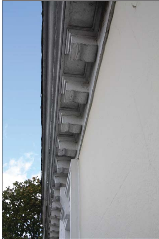
Plate 9: Detail of modillions along the cornice of the west elevation
