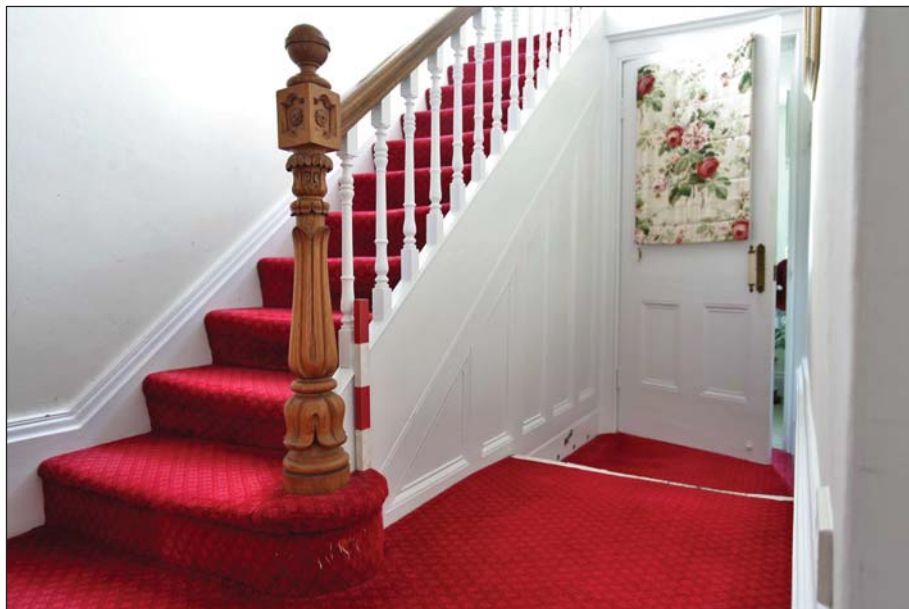
Plate 22: G1, detail of newel post of the staircase
