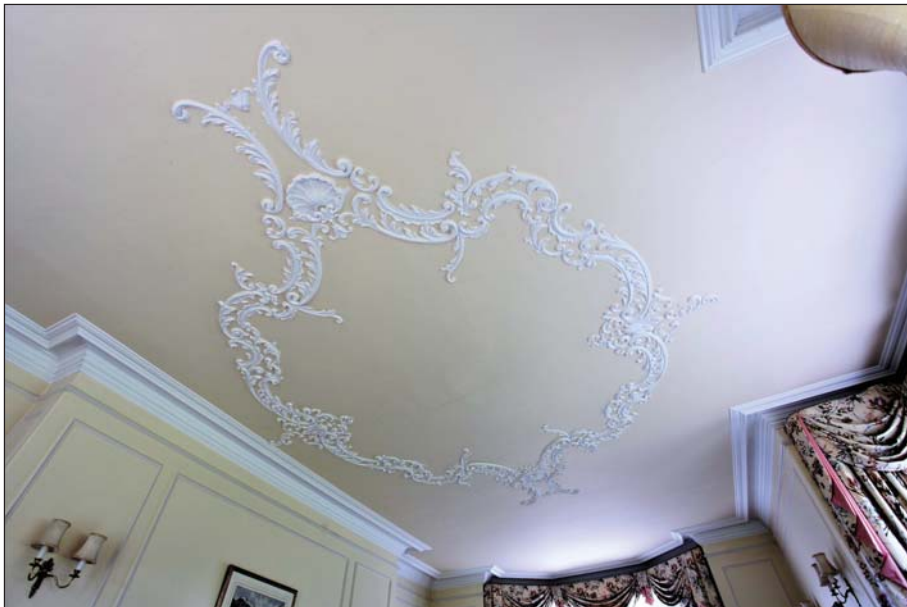
Plate 28: Detail of decorative plaster ceiling
