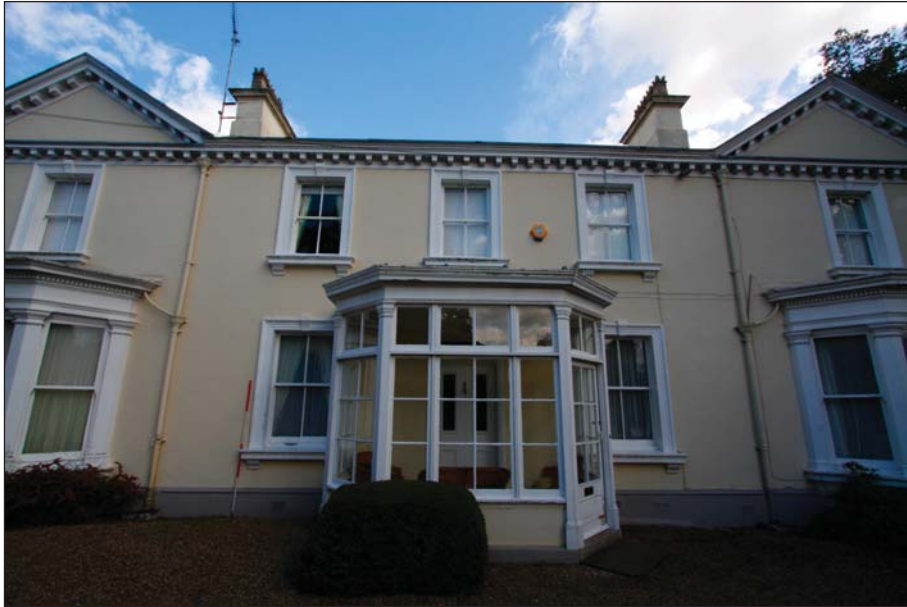
Plate 5: Central area of the west elevation with projecting porch
