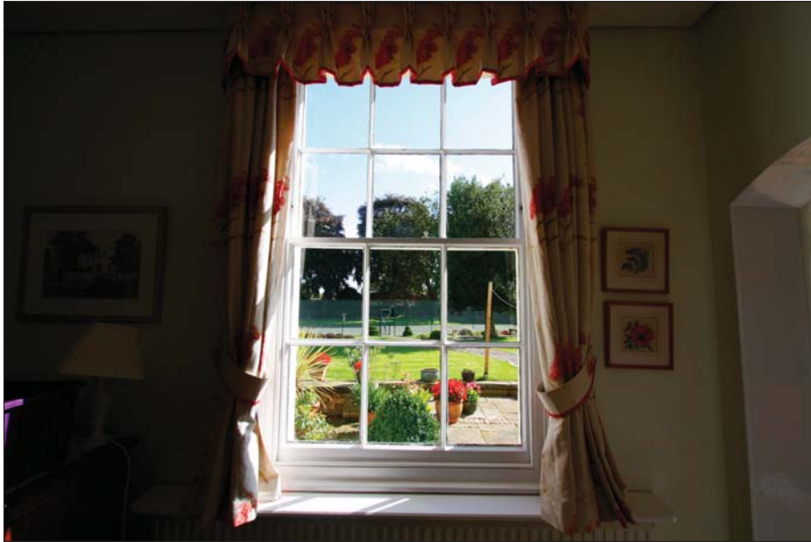
Plate 41: Detail of inserted sash window within the east wall of G9
