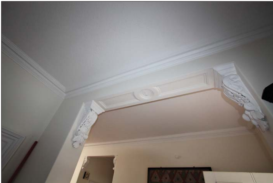
Plate 24: Detail of decorative plaster consoles of doorway opening between G1 and G2
