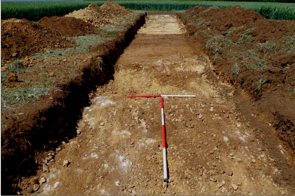
Plate 25: Ditches 906 and 904, pre-ex, view from the south-west
