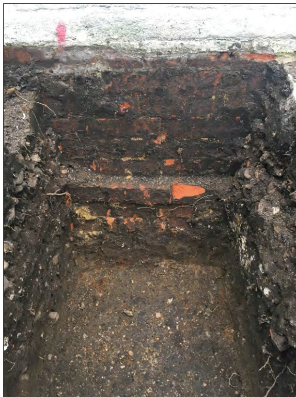
Plate 4: View of foundations of existing building with natural gravel geology, view from west
