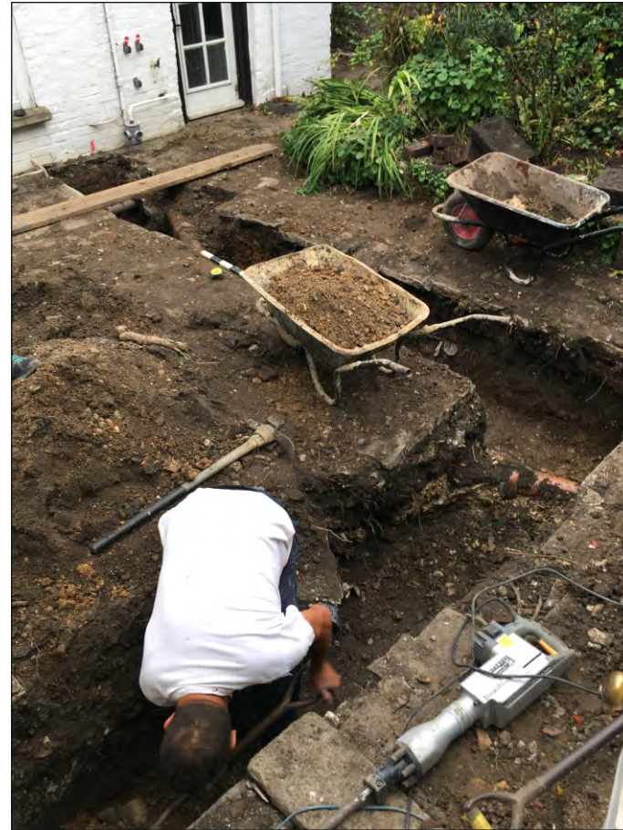
Plate 2: Working shot during excavation of footings, view from north-east
