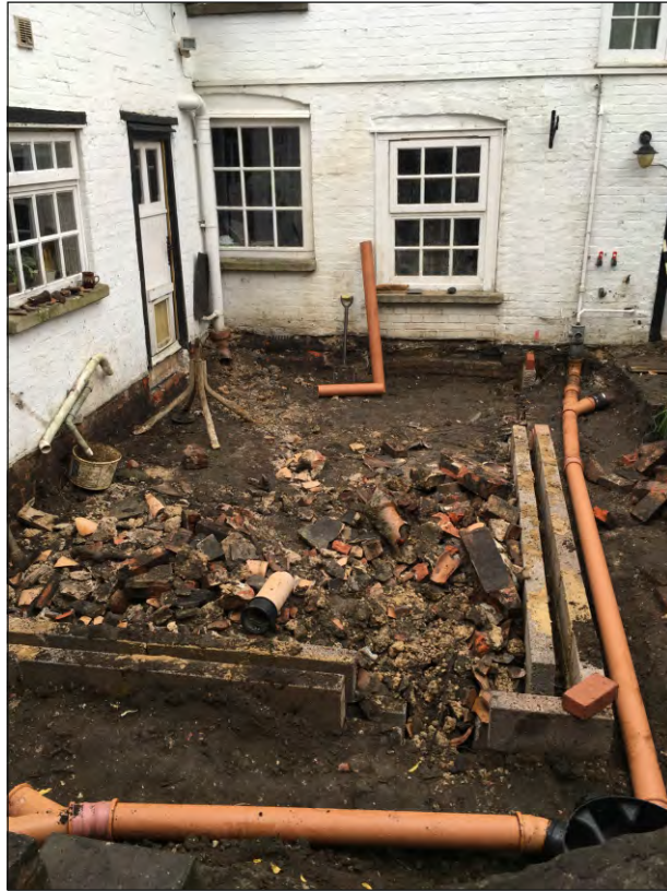
Plate 5: Working shot of final reduced levels, view from north
