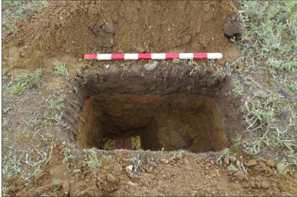
Plate 7: Water pipe test pit, viewed from the west
