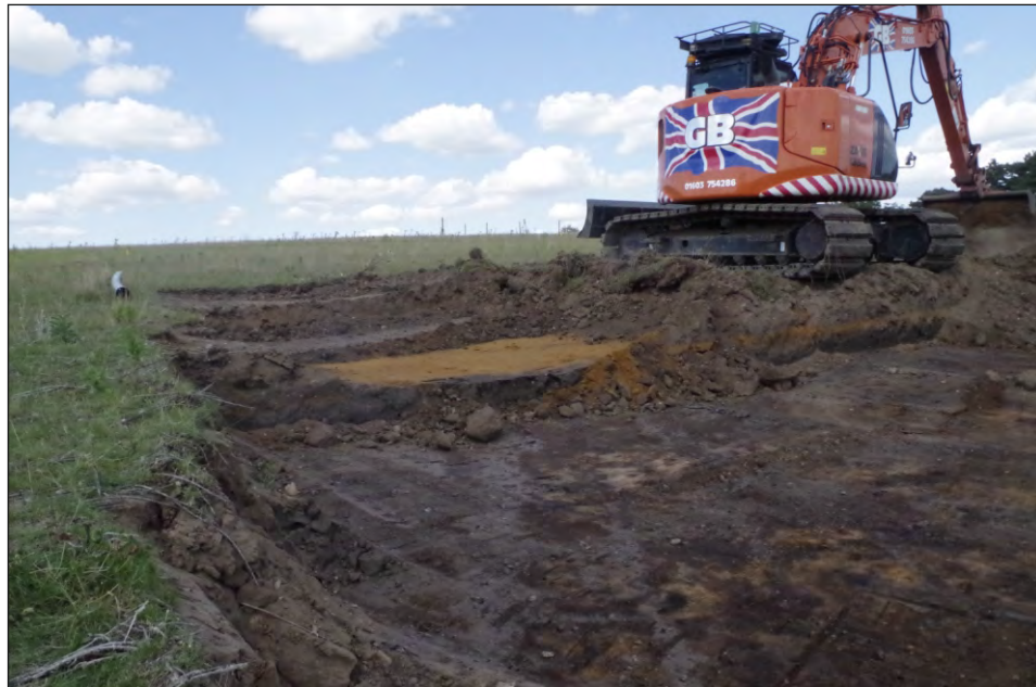
Plate 18: Ground reduction of berm in northern field, viewed from the southwest
