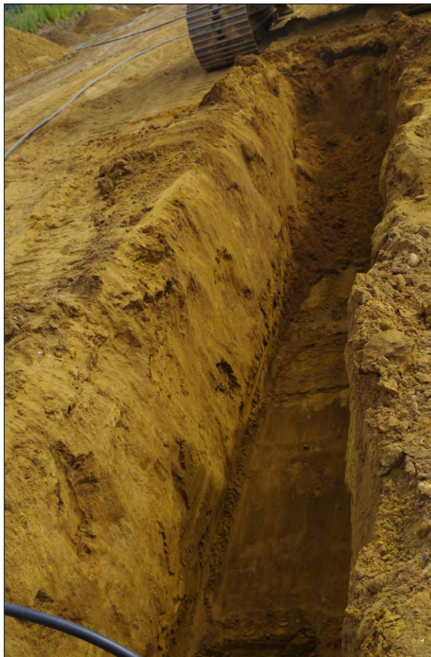
Plate 12: Cable trenches in western field, viewed from the west
