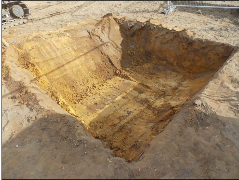
Plate 3: HDD receiver pit in eastern field/compound area, viewed from the south
