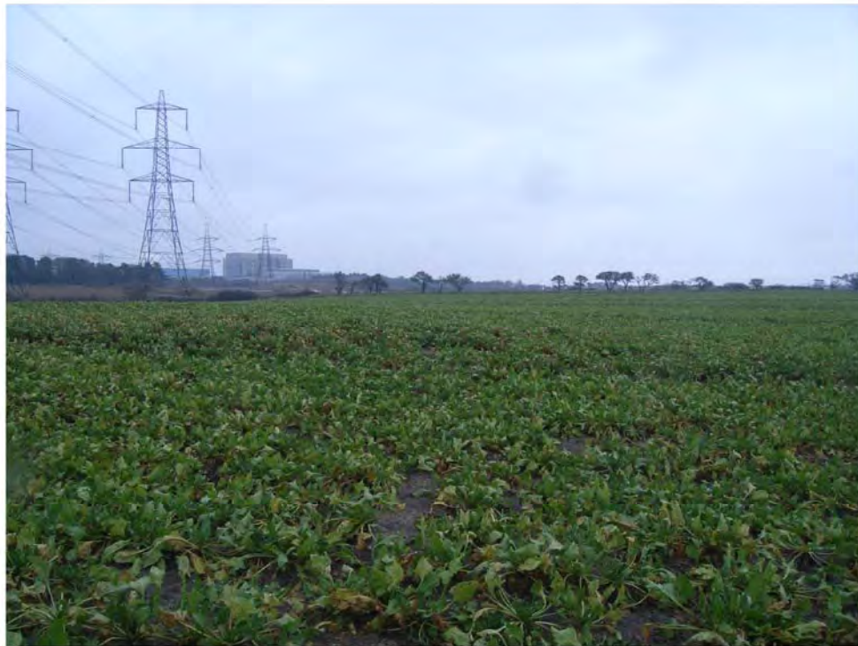
Plate 4 Location of substation 2
