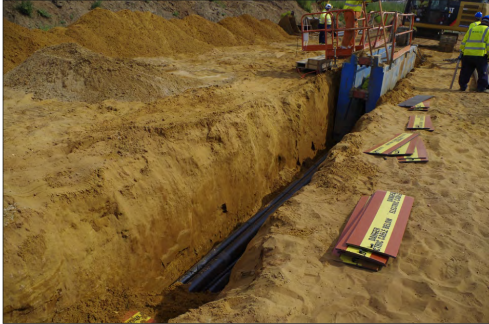
Plate 13: Cable trenching in western field, viewed from the southwest
