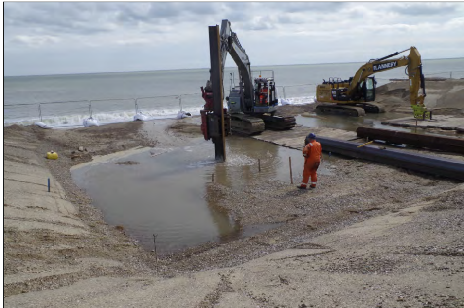
Plate 22: Working shot of piling for the cofferdam, viewed from the northwest
