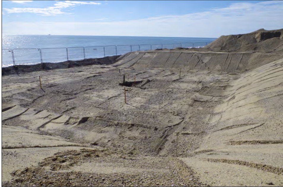
Plate 21: Stripping of beach area, viewed from the northwest
