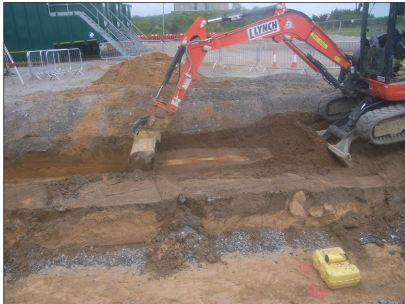
Plate 2: Cable trenches in eastern field/compound area, viewed from the south
