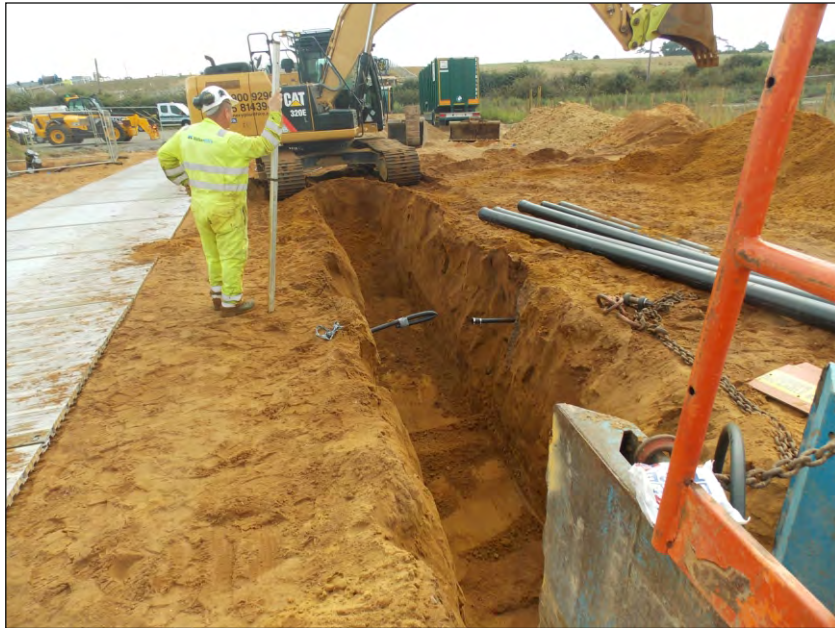
Plate 4: Cable trenching in eastern field/compound area, viewed from the west
