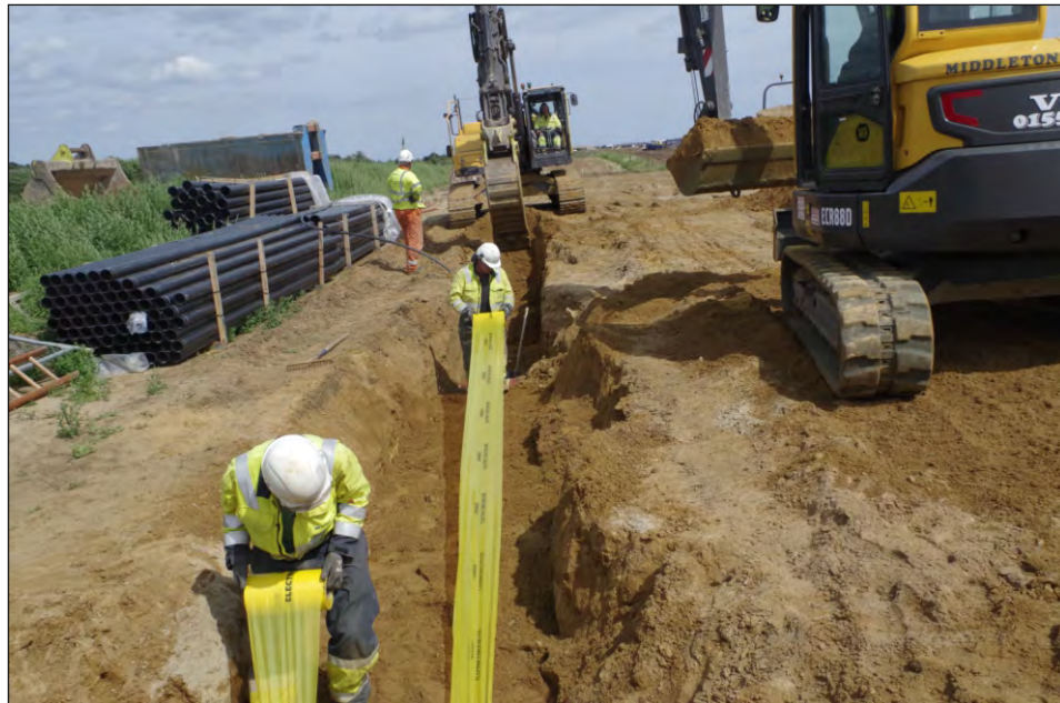
Plate 14: Cable trenching in western field, viewed from the west
