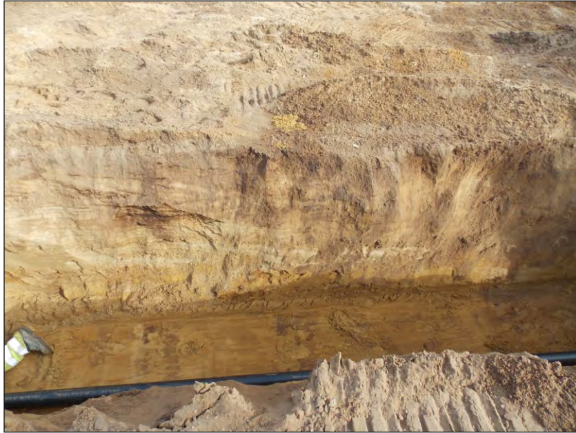
Plate 15: Cable trench in northern field, viewed from the west
