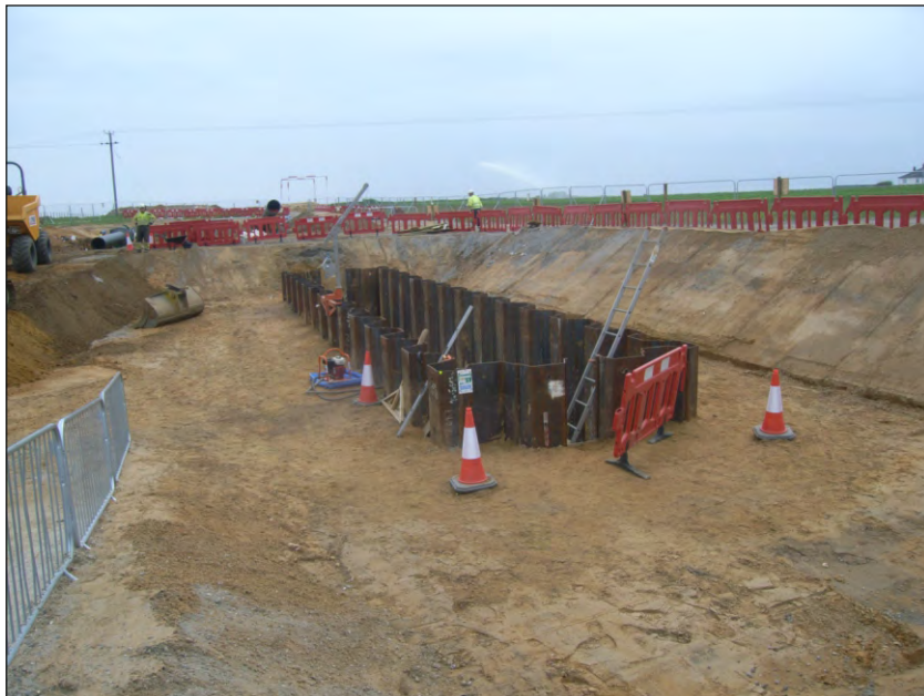
Plate 6: Transition joint bay in eastern field/compound area, viewed from the northwest
