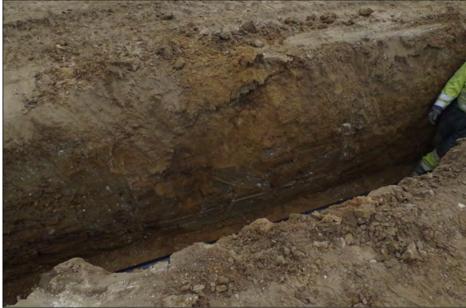
Plate 17: Cable trench in northern field, viewed from the northwest
