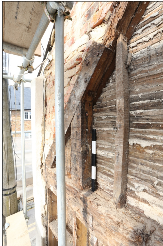
Plate 22: The north-east side of the south-west elevation at tie-beam level showing some modern repairs
