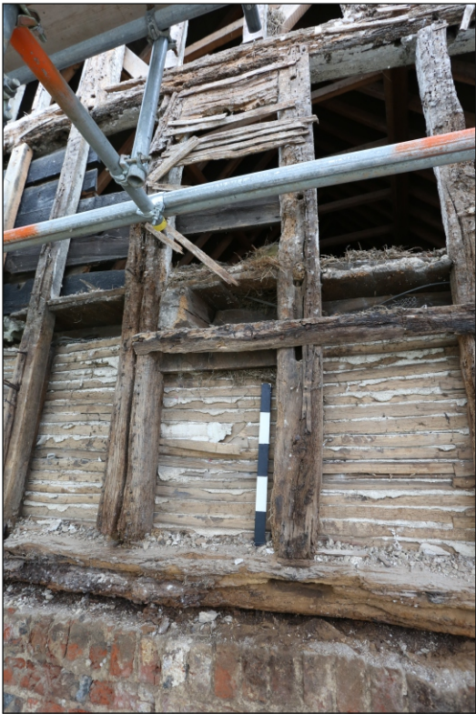
Plate 36: Reused timber stud and remnant lath and plaster located towards the centre of the south-east elevation beneath the tie-beam
