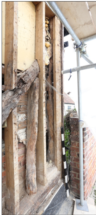
Plate 24: The earlier and modern south-east posts in the south-west elevation. Note the empty mortices
