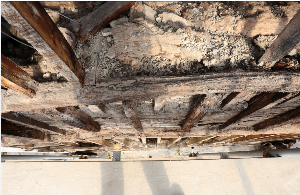
Plate 29: The groove in the top of the collar in the south-west elevation
