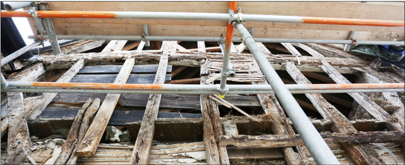
Plate 35: Soffit of the tie-beam in the south-east elevation showing stave holes and empty mortice
