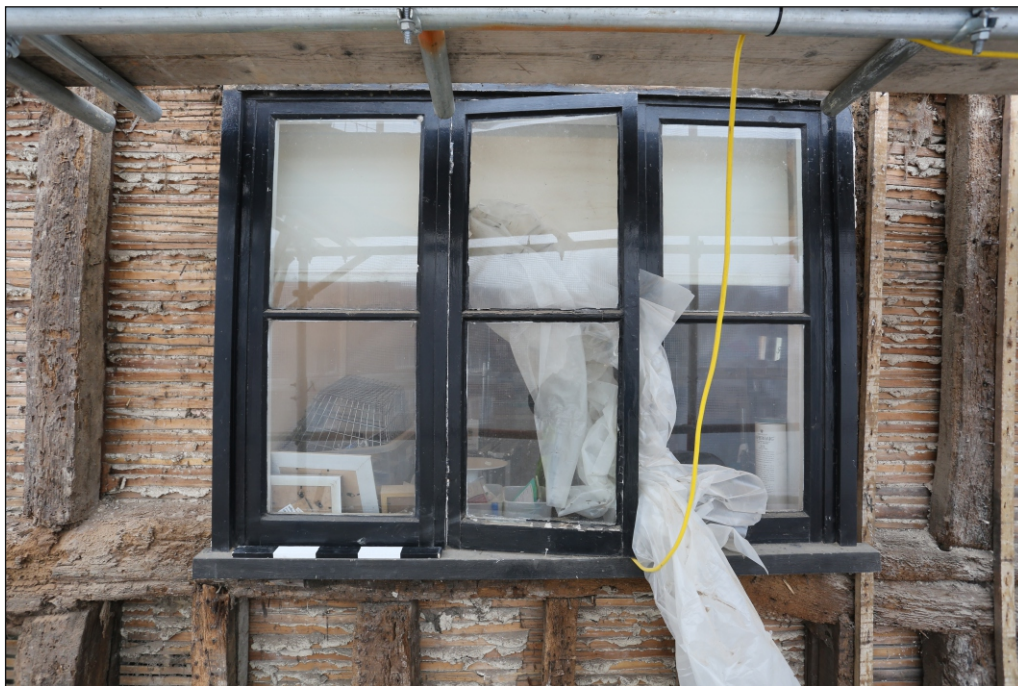
Plate 10: The north-east elevation first floor window
