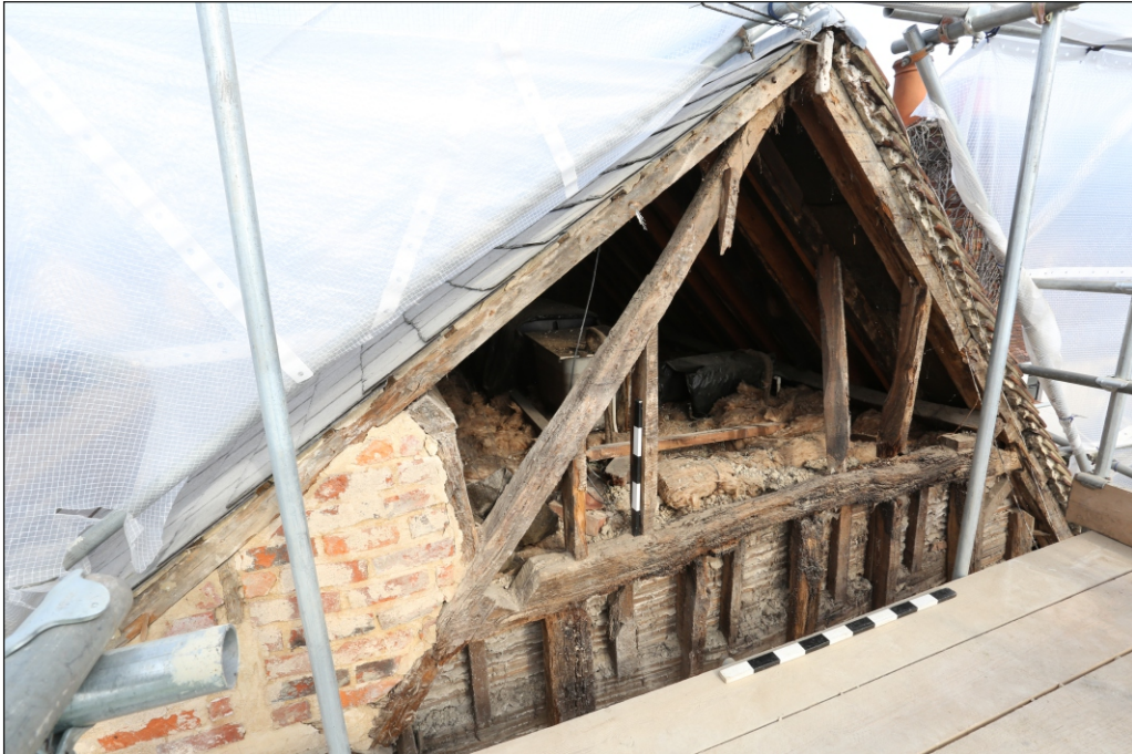
Plate 23: The south-west elevation at collar/roofspace level, viewed from the west
