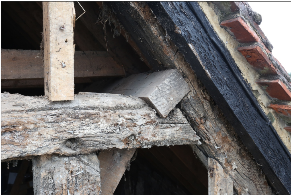
Plate 38: North-east end of the collar, the clasped purlin and reduced principal rafter in the south-east elevation
