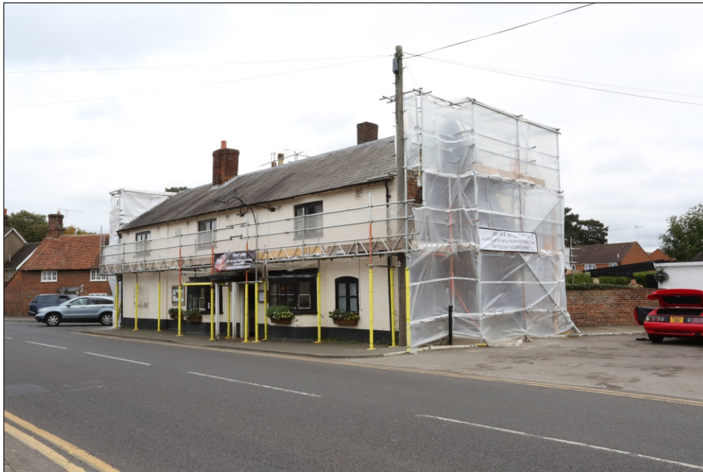
Plate 3: The Rose & Crown public house when scaffolded, viewed from the south-west
