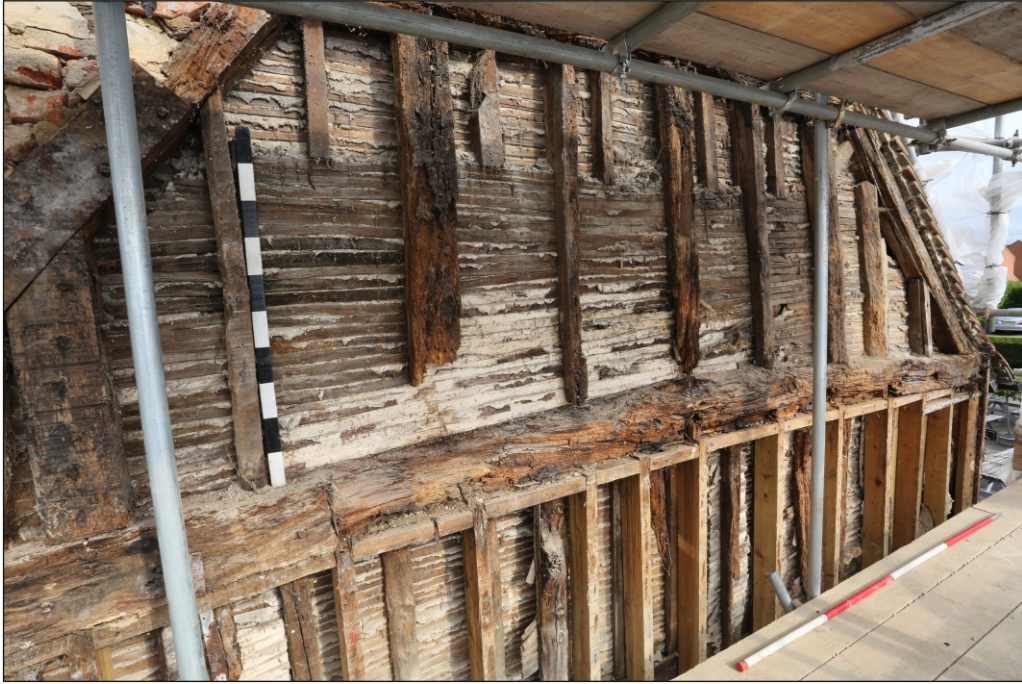
Plate 21: The south-west elevation at tie-beam level, viewed from the west
