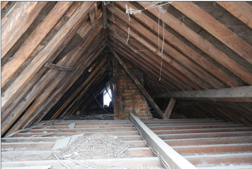
Plate 18: The roofspace of the main range viewed from the north-east
