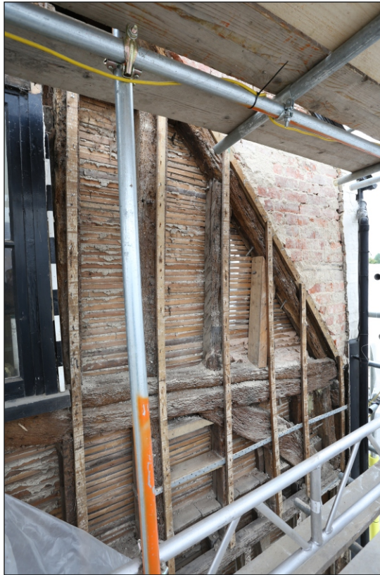
Plate 11: The north-west side of the north-east elevation at tie-beam/first floor level
