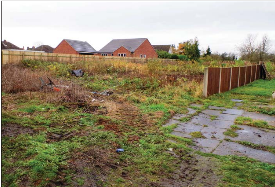
Plate 1: Entrance and general view of the Site, looking south-west
