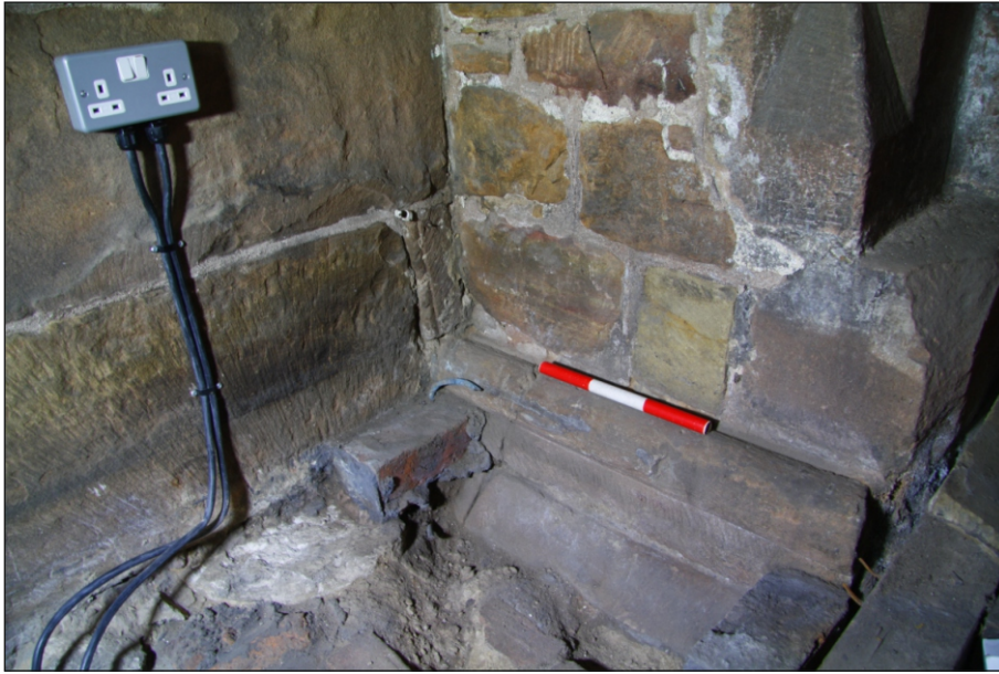
Plate 15: External Norman plinth (104) on the south side of the Chancel and architectural fragment (105) reused as foundation of the pier under the wall of Jesus Chapel/South Chapel
