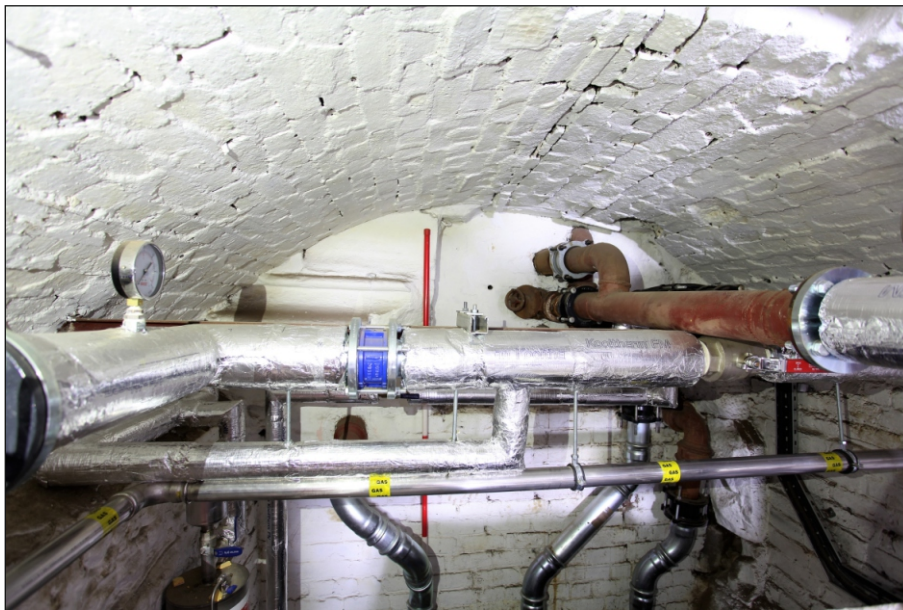
Plate 2: Vaulted Boiler House with inserted wall to the west
