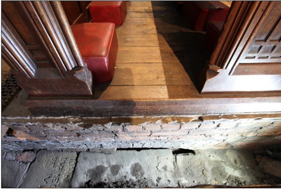
Plate 19: Burial vaulted chamber (108) adjacent to ledger stone (107) incorporated into the brick-lined duct
