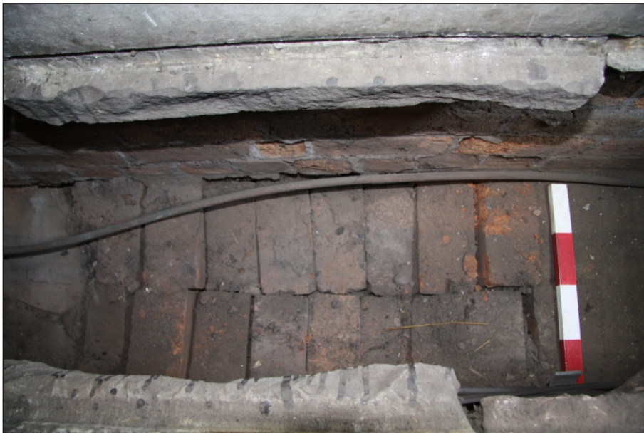
Plate 12: Brick paving with void beneath the floor within the duct across the Chancel
