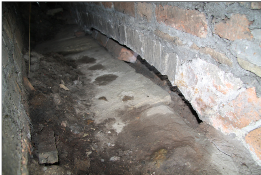
Plate 20: Arched head of the vaulted chamber (108) with later brickwork above
