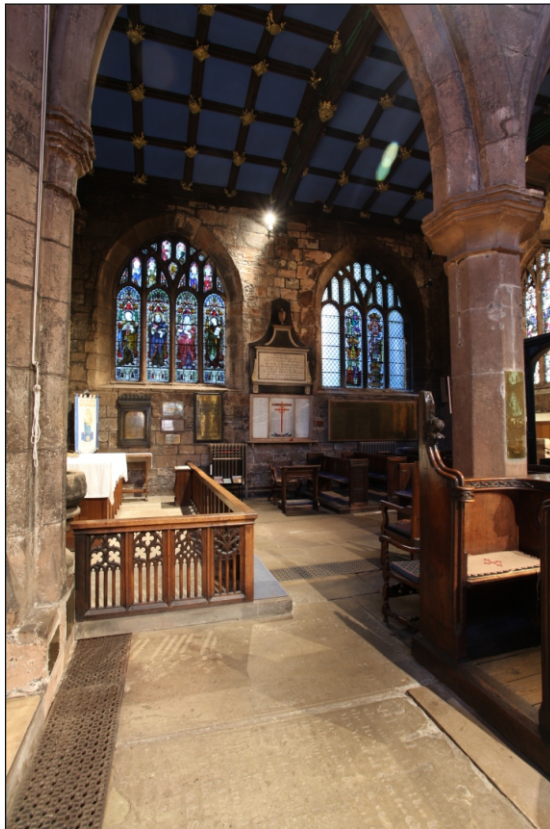
Plate 1: General internal view of Rotherham Minster showing the floor with ducts covered with cast-iron grilles
