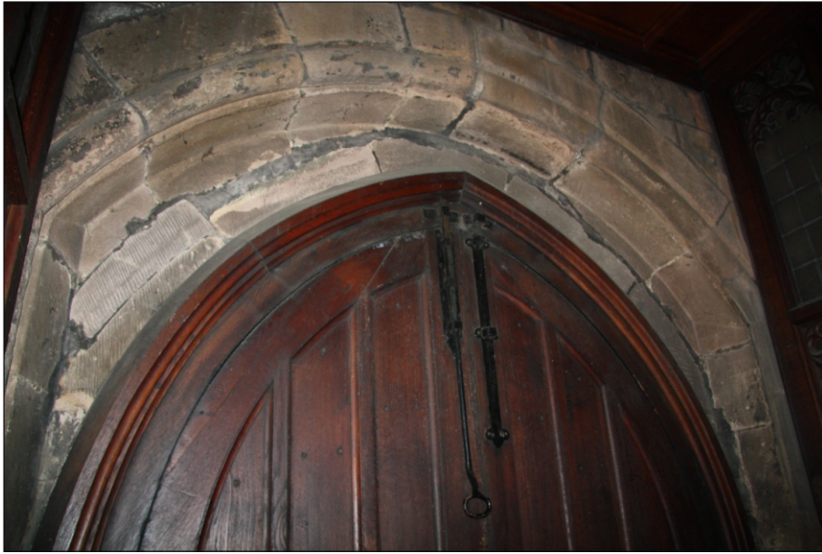
Plate 9: Internal face of the West Porch's doorway with round arch decorated with roll moulding edge
