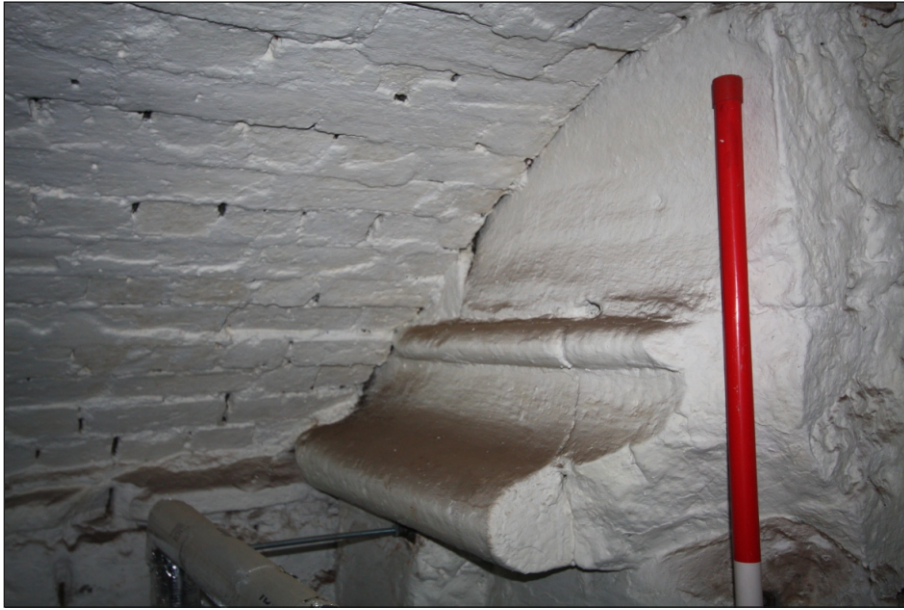
Plate 3: Detail of truncated 15th century external wall with moulded string course
