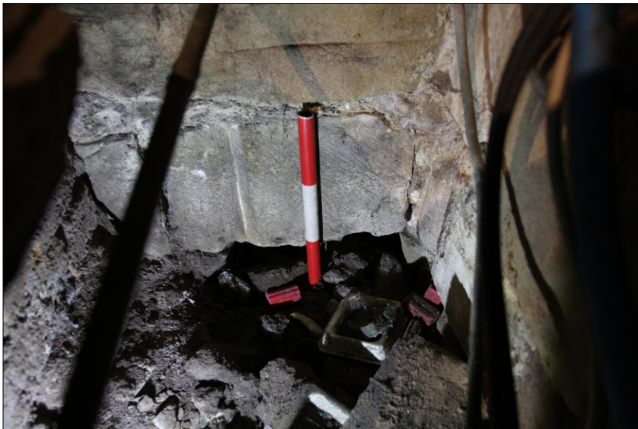
Plate 8: Architectural fragment (102) adjacent to (101) acting as foundation of the north-east corner of the north chapel/organ chamber
