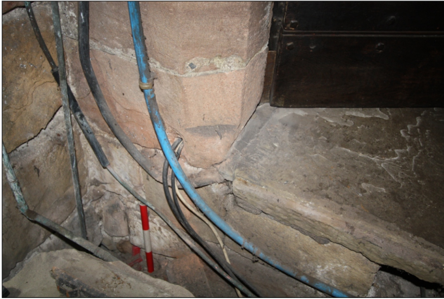
Plate 7: Architectural fragment (101) beneath the doorway of the Clergy Vestry
