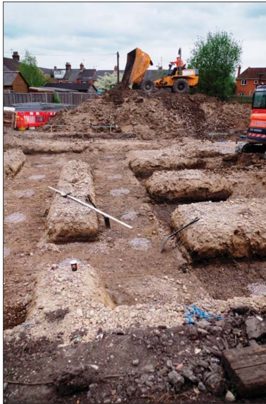
Plate 9: Trench 9 showing foundation trenches and underlying general mixed alluvial deposits and round stone filled piling columns
