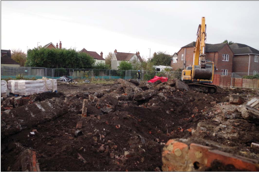
Plate 1: Removal of shallow foundations of demolished almshouses
