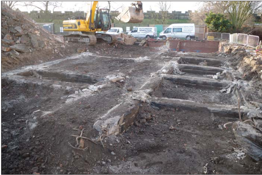
Plate 1: Concrete foundations of Oliver House within areas 1, 3 and 6 and cellar walls 401
