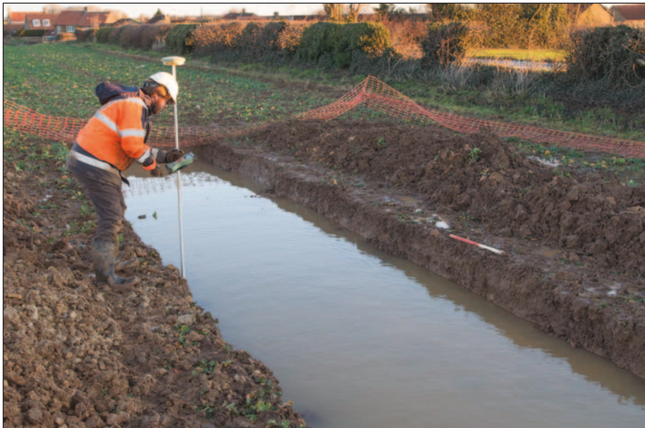
Plate 16: Ground water in Trench 9
