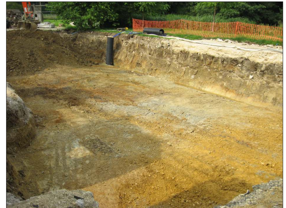
Plate 4: Post-excitation shot of trench, north-west end
