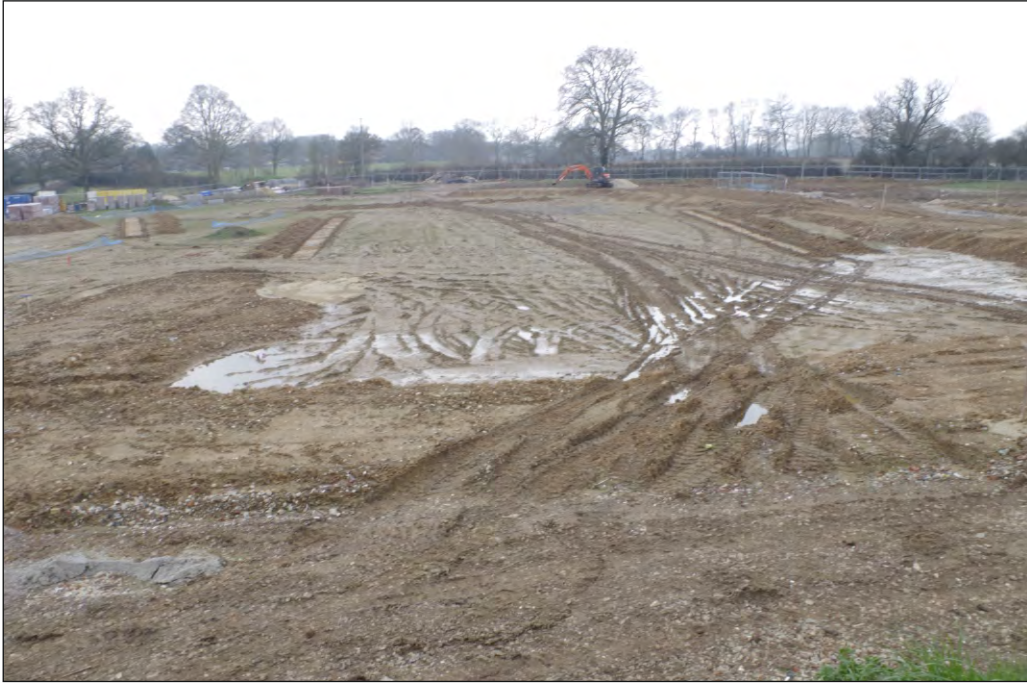
Plate 1: Overview of the Site from the north
