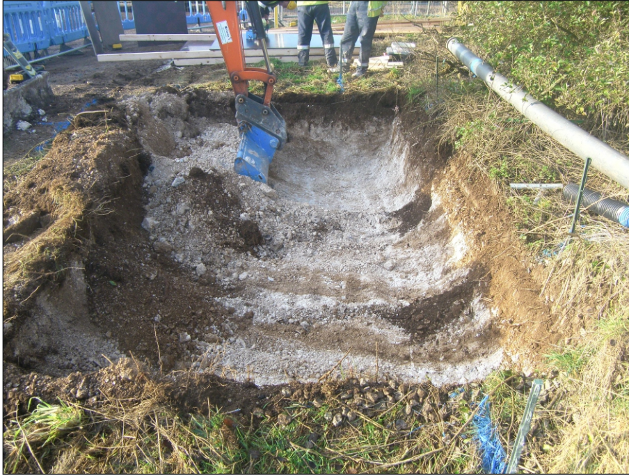
Plate 1: Footprint of substation, view from the north
