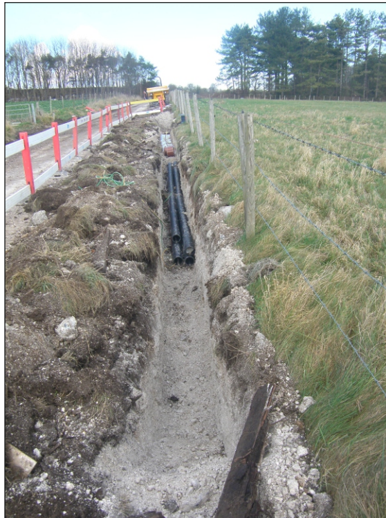
Plate 2: Cable route, view from the south
