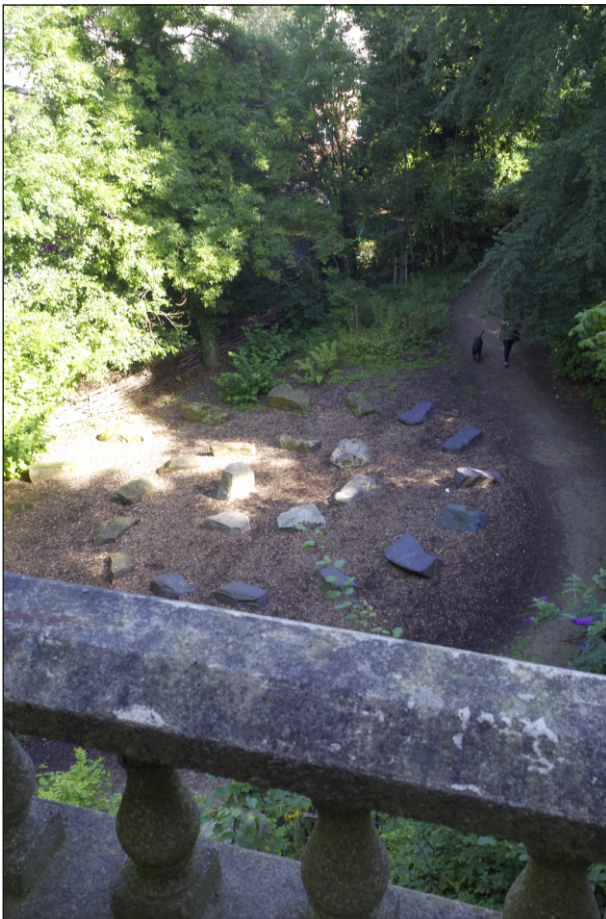
Plate 30: View from the top of the Grade II listed catacombs down towards Porter Brook, from the south-west
