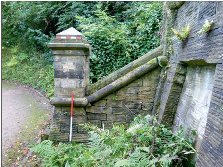
Plate 2: General shot of staircase CC1, view from west
