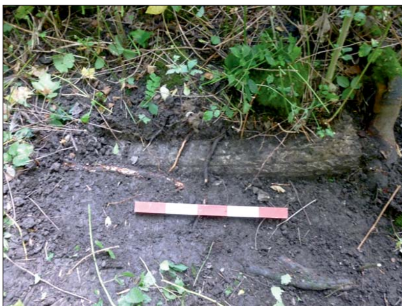
Plate 14: Detail shot of stone capping on top of vault wall NCC1
