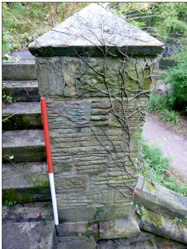
Plate 6: Detail shot of interior stone wall of staircase, central landing
