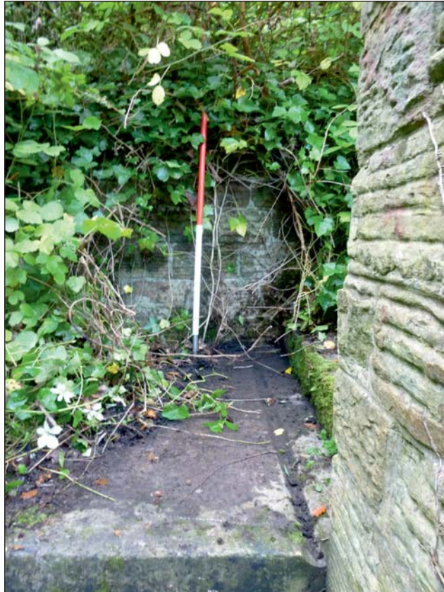
Plate 7: Detail shot of southern rear wall of staircase
