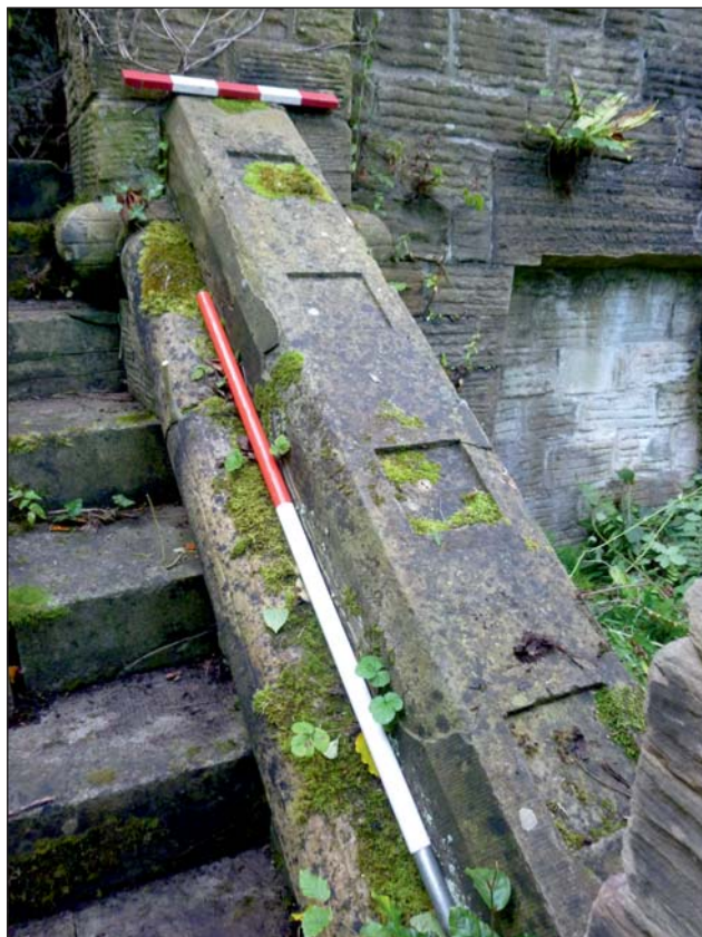
Plate 4: Detail shot of balustrade carving from interior of staircase
