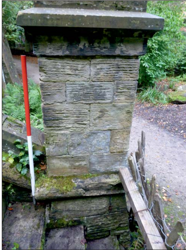
Plate 5: Detail shot of interior stone wall of staircase, lower level
