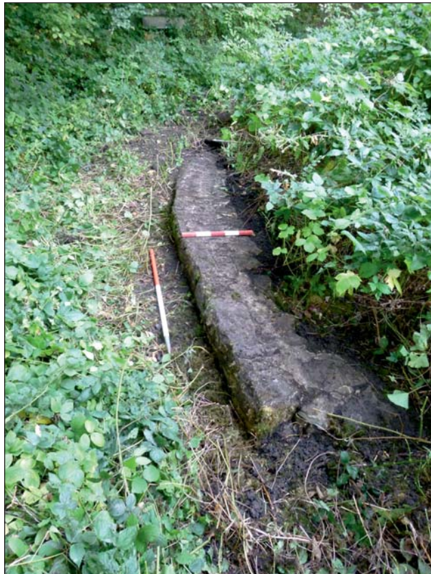
Plate 10: General shot of vault wall NCC1, view from north
