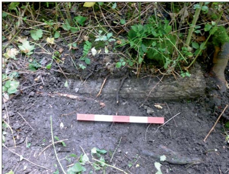
Plate 45: Detail shot of stone capping on top of vault wall
