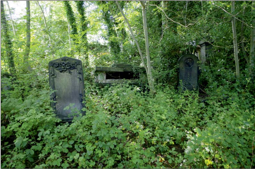
Plate 9: A damaged monument with its end open
