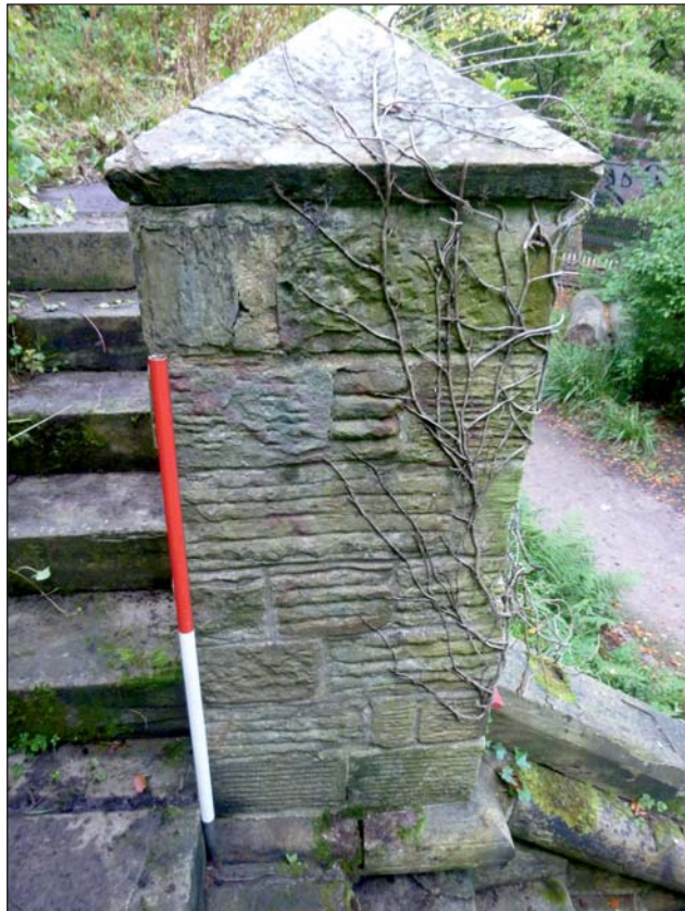
Plate 37: Detail shot of interior stone wall of staircase, central landing
