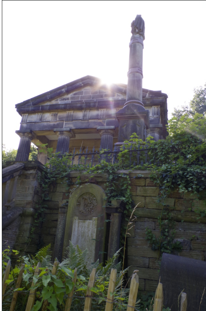
Plate 31: View towards the Grade II* listed Non Conformist Chapel, from the north-west
