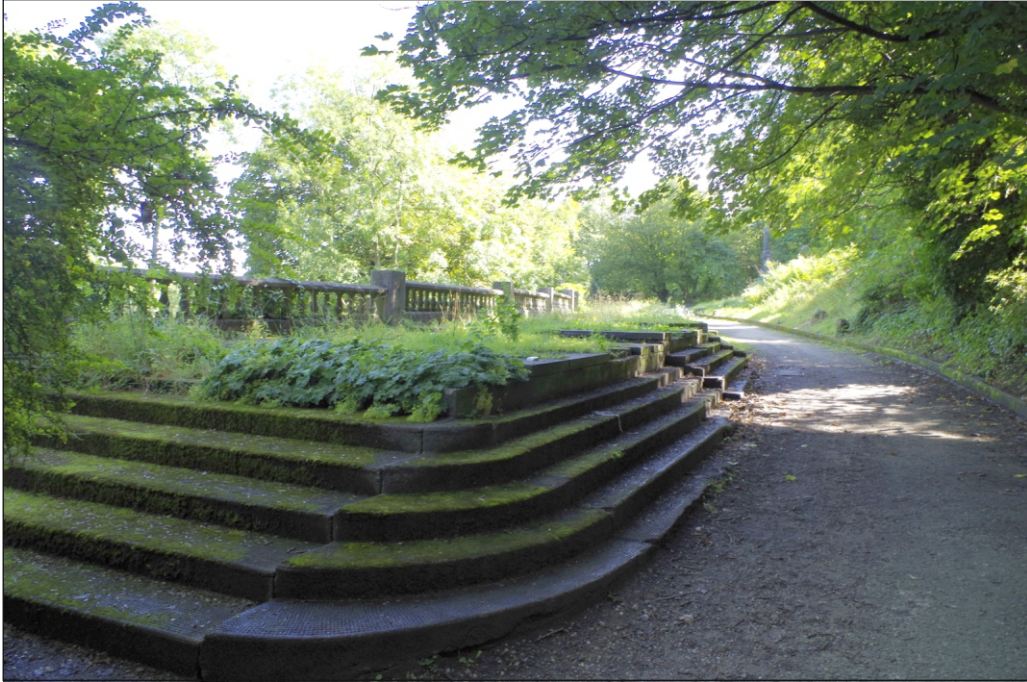
Plate 29: View across the top of the Grade II listed catacombs, from the south-south-west
