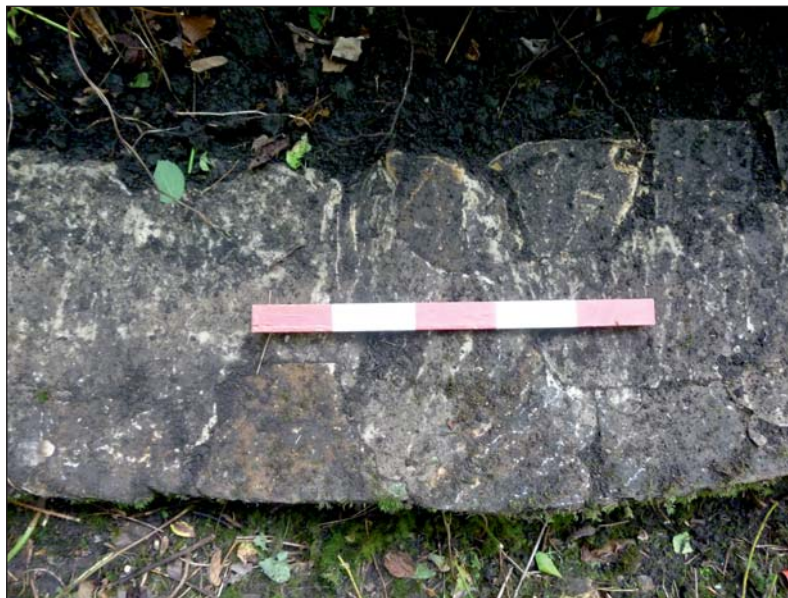
Plate 43: Overhead shot of vault wall, showing construction
