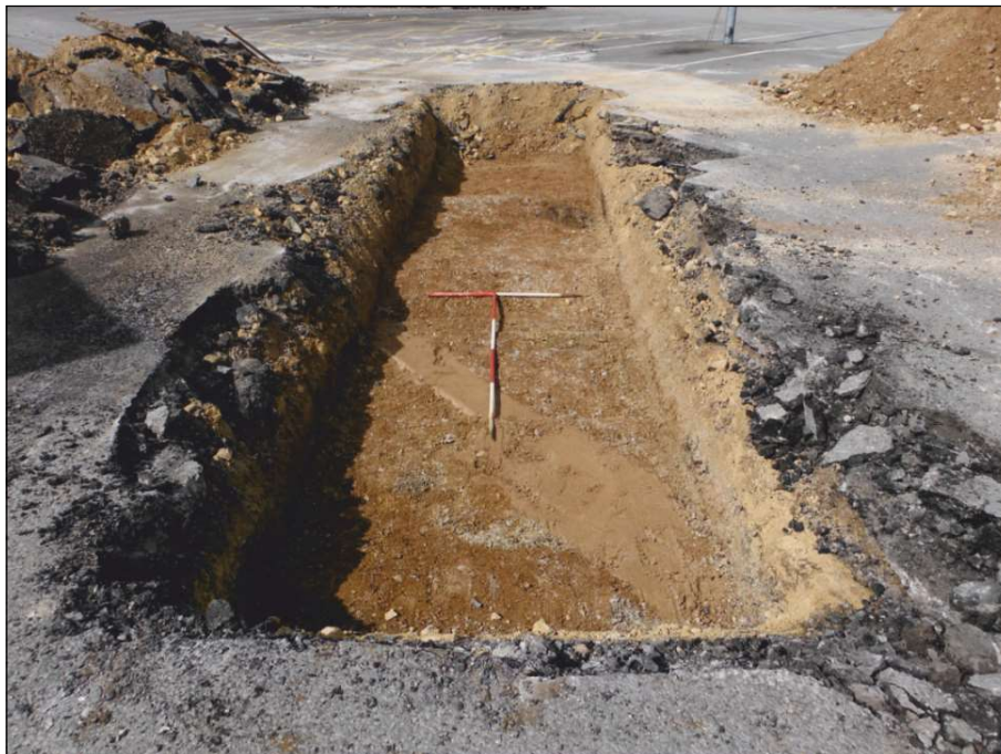
Plate 4: General shot of trench 2, facing northwest
