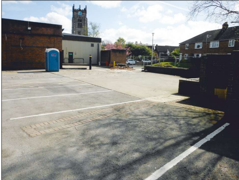
Plate 1: General shot of the car park pre-excitation
