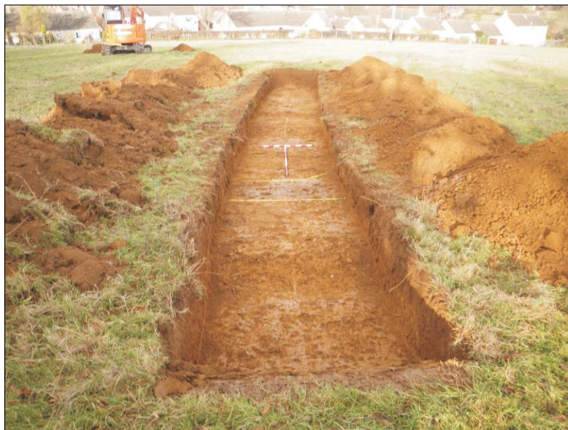
Plate 2: General view of Trench 1
