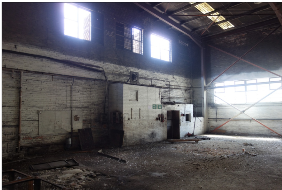
Plate 80: Internal view of Building 12, looking east
