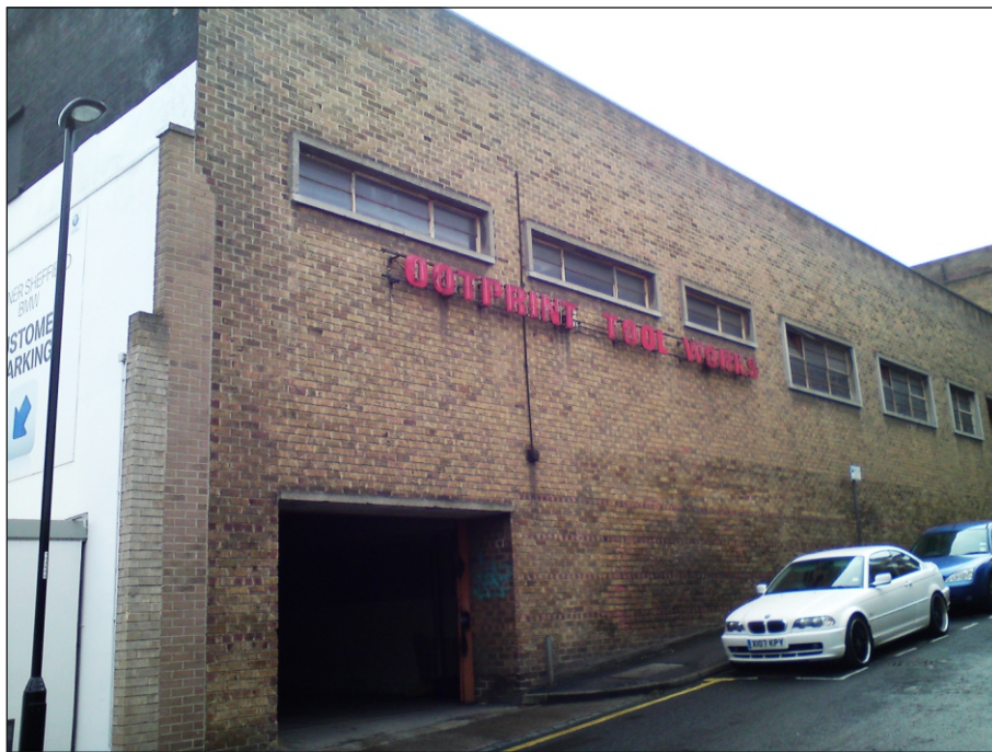
Plate 32: Easternmost end of the north elevation with evidence of earlier walls
