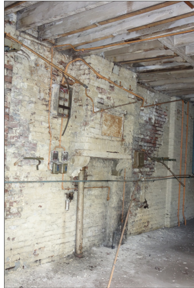
Plate 106: Chimney breast supported by sandstone corbels
