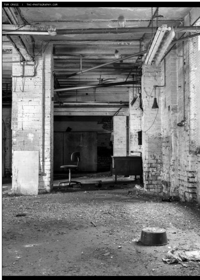
Plate 100: Ground floor of Building 16, looking south
