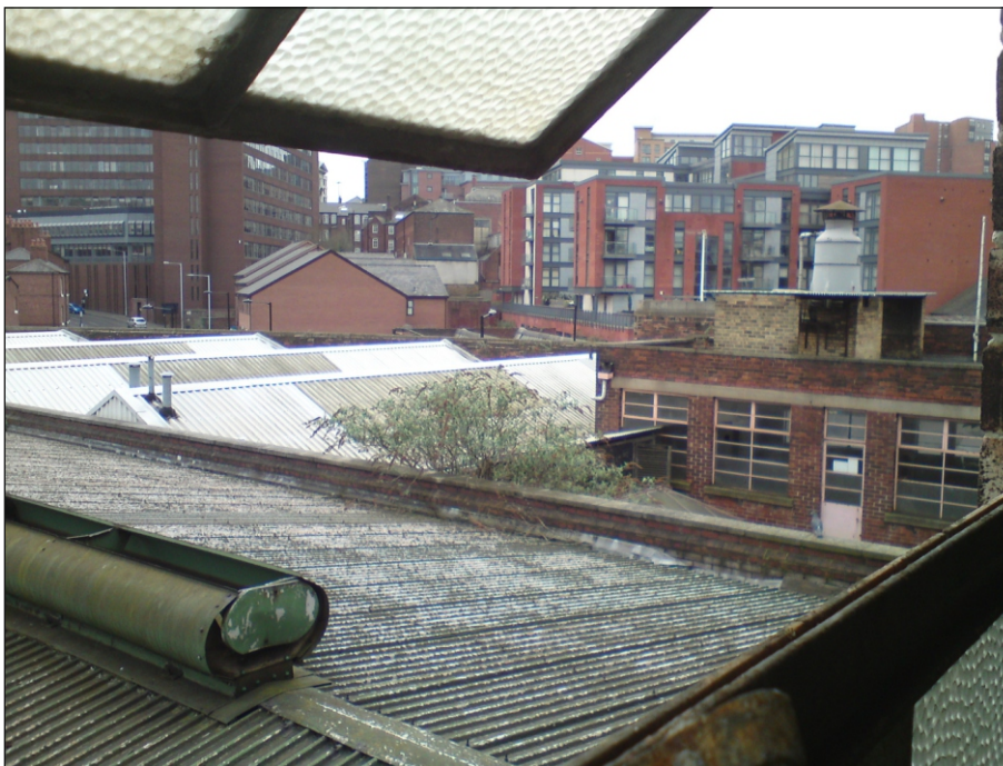
Plate 108: Court 1, viewed from the second floor of Building 14
