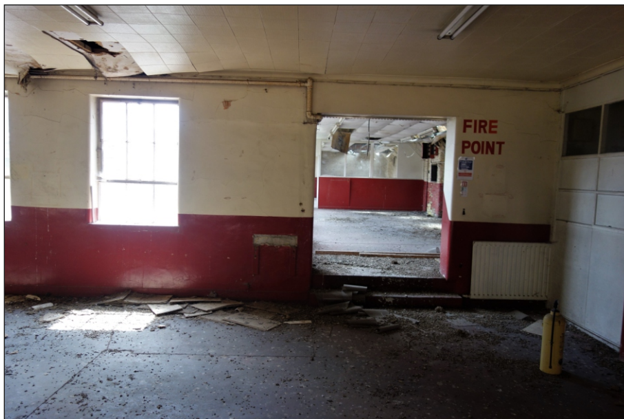
Plate 54: Internal view of the ground floor of Building 6
