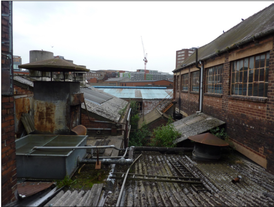
Plate 103: East elevation of Building 17 showing reduced window openings within the top storey
