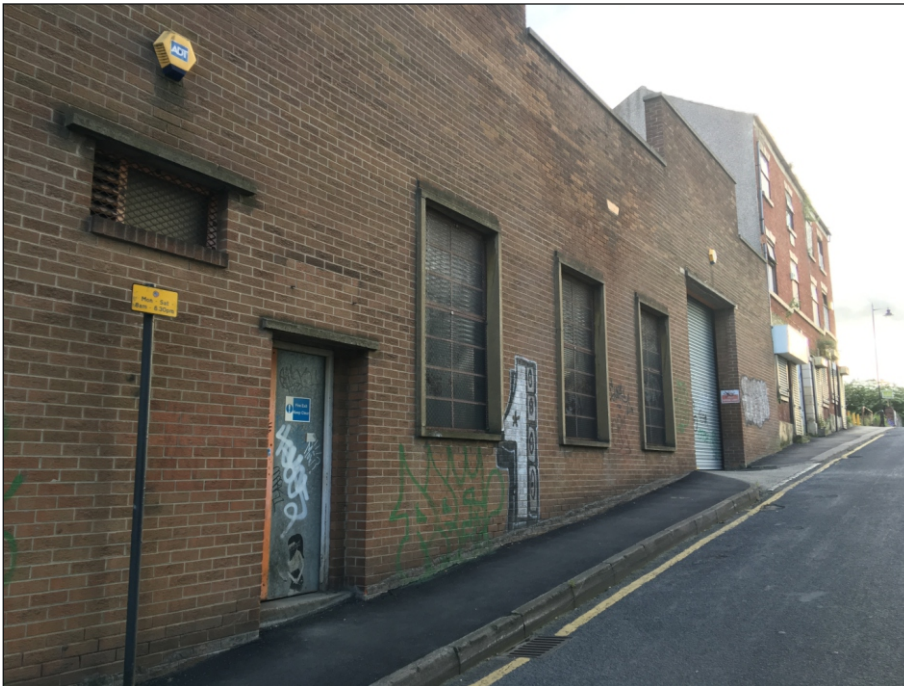
Plate 64: Front elevation of Building 10, looking north-west
