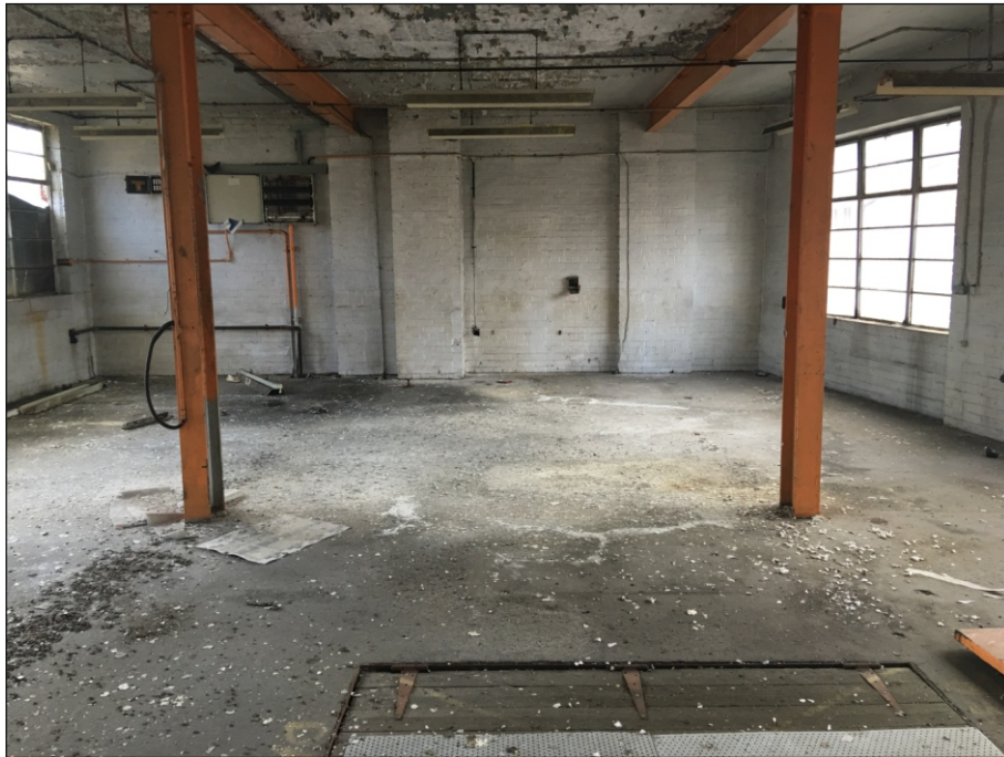
Plate 89: Eastern side of the first floor of Building 13
