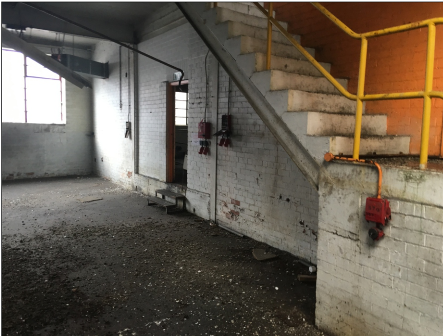
Plate 86: Eastern side of the ground floor of Building 13, looking south-west
