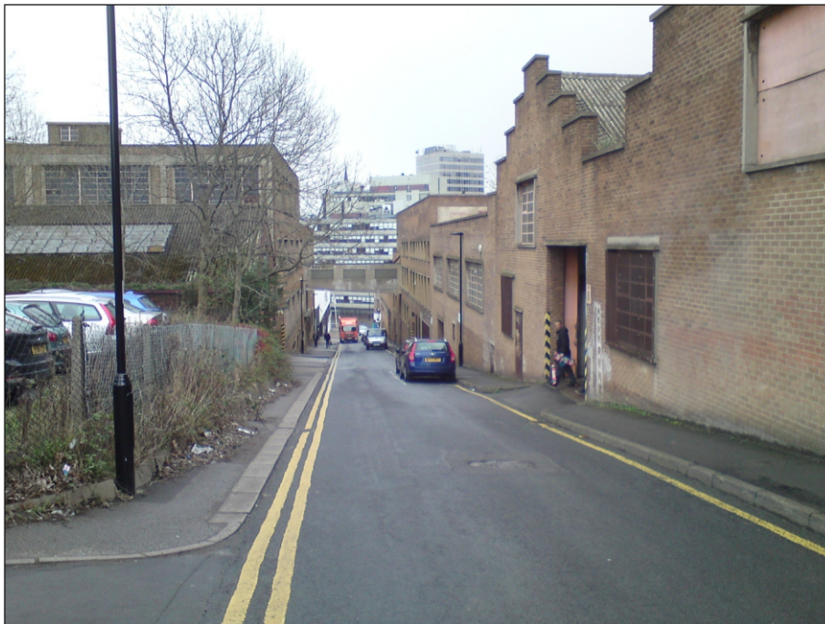
Plate 56: Front elevation of Building 8 facing onto Hollis Croft
