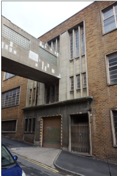
Plate 22: Principal doorway area with concrete panels and bridge across Hollis Croft
