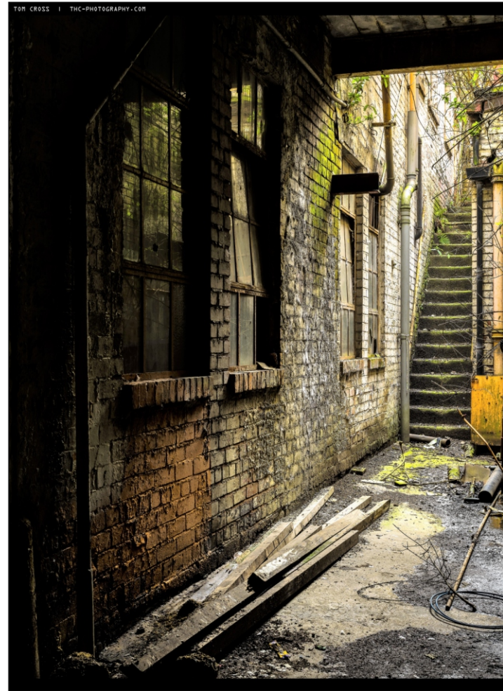
Plate 98: Window openings along the west elevation of Building 16
