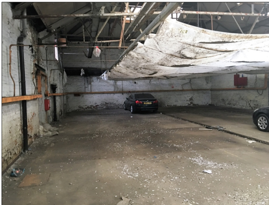
Plate 60: Internal view of Building 8
