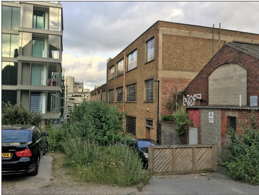
Plate 15: Rear elevation of Building 2 facing onto White Croft, viewed from the west
