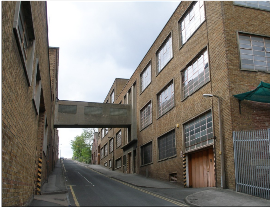
Plate 19: Building 3 along Hollis Croft (courtesy of Dinah Saich)
