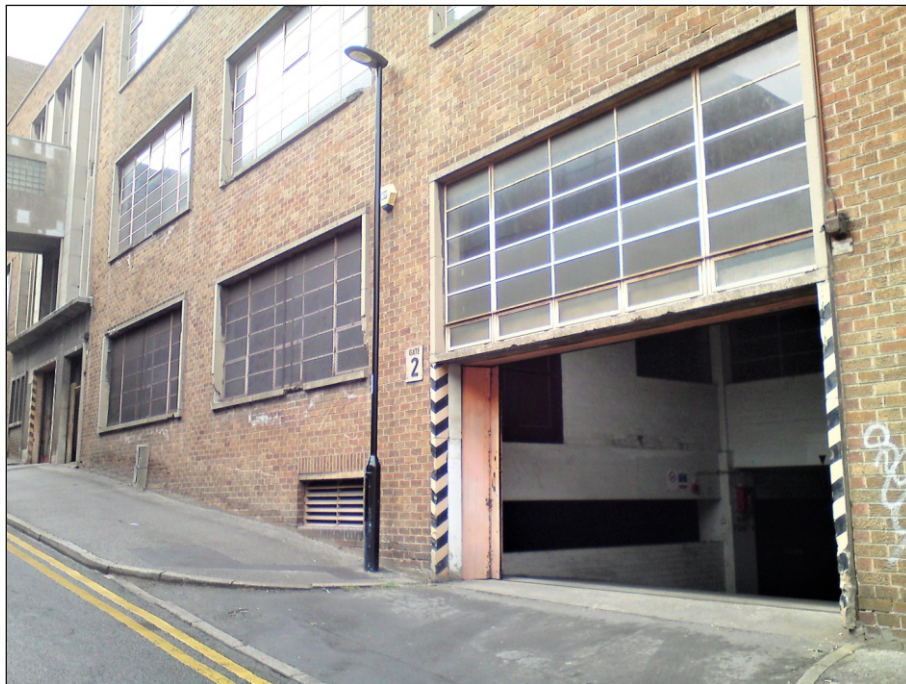
Plate 20: Eastern end of Building 3 with doorway to underground car park along Hollis Croft
