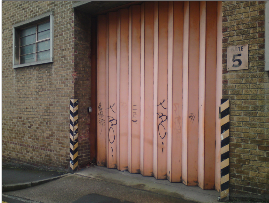
Plate 33: Concertina doorway - Gate 5 - along Hollis Croft
