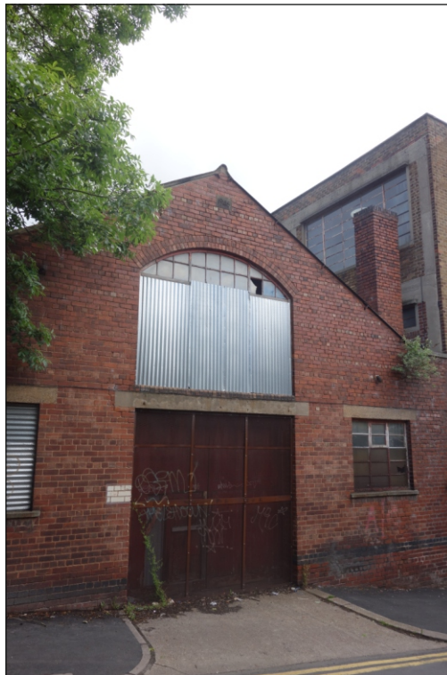
Plate 6: Front elevation of Building 1 showing its date plaque '1946' to the top of the gable
