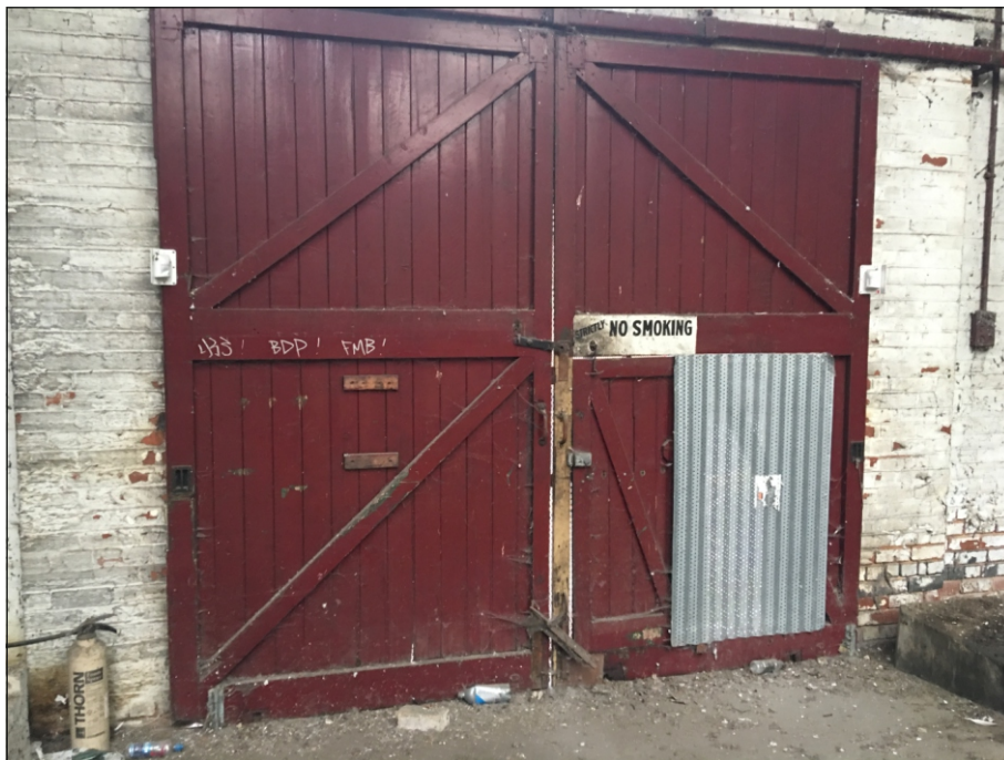
Plate 12: Detail of sliding ledged timber doors
