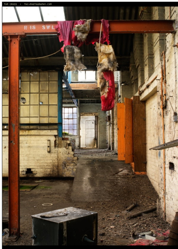
Plate 94: Southern end of the first floor with ramp to adjacent Building 15
