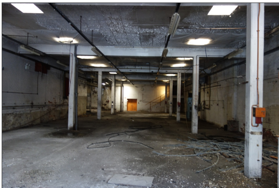
Plate 72: Internal view of Building 11
