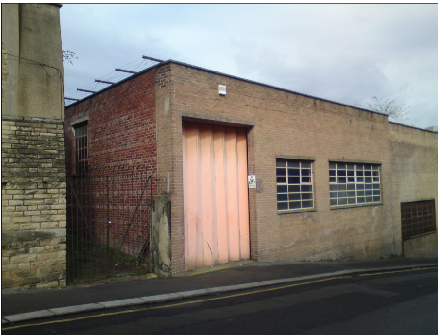
Plate 70: Front elevation of Building 11 facing onto Garden Street
