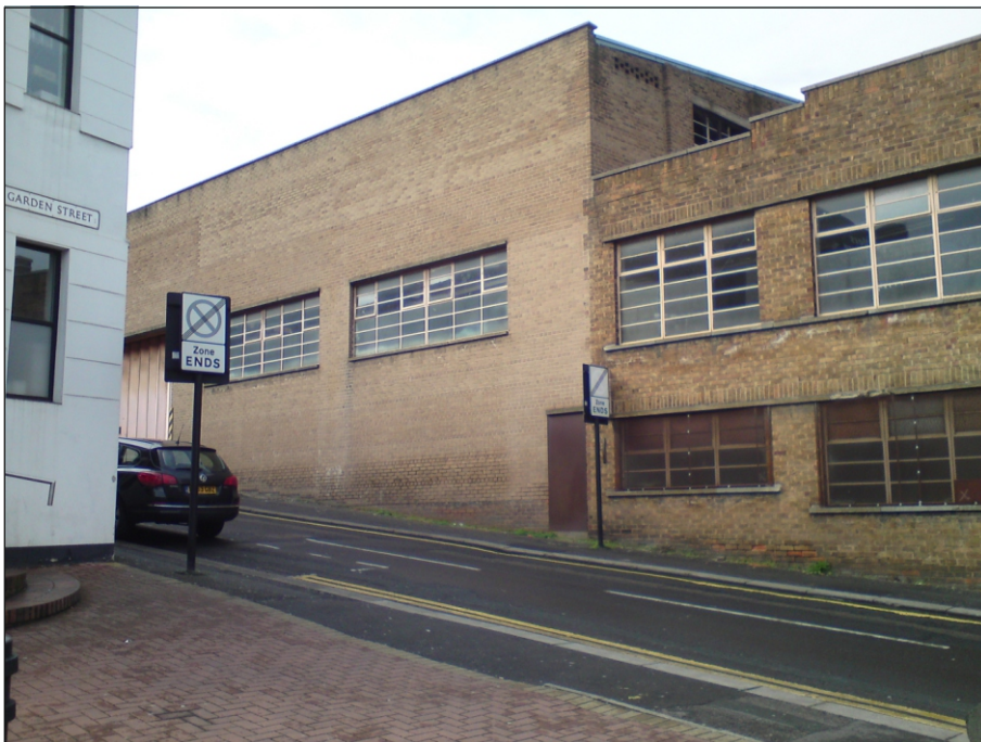
Plate 78: Eastern end of the front south elevation of Building 12
