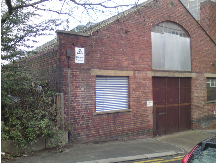
Plate 5: Front elevation of Building 1 facing onto Hollis Croft
