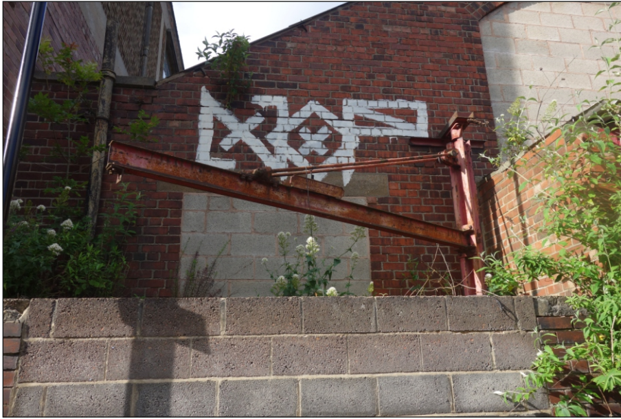
Plate 9: Detailed view of crane
