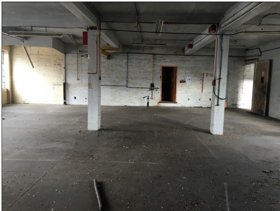
Plate 90: Western side of the first floor of Building 13
