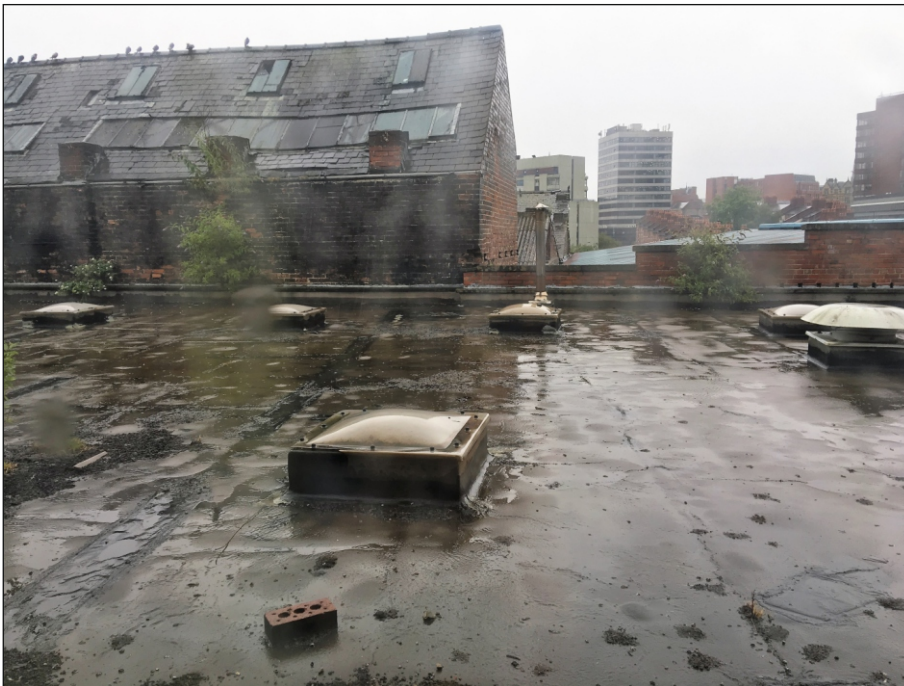
Plate 104: Upper section of the west elevation of Building 17 showing blocked-up chimney stacks
