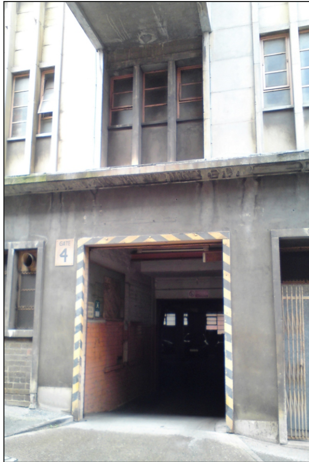
Plate 23: Doorway to underground car park beneath the bridge
