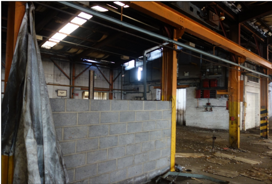
Plate 42: Building 4, looking south-west towards Building 14
