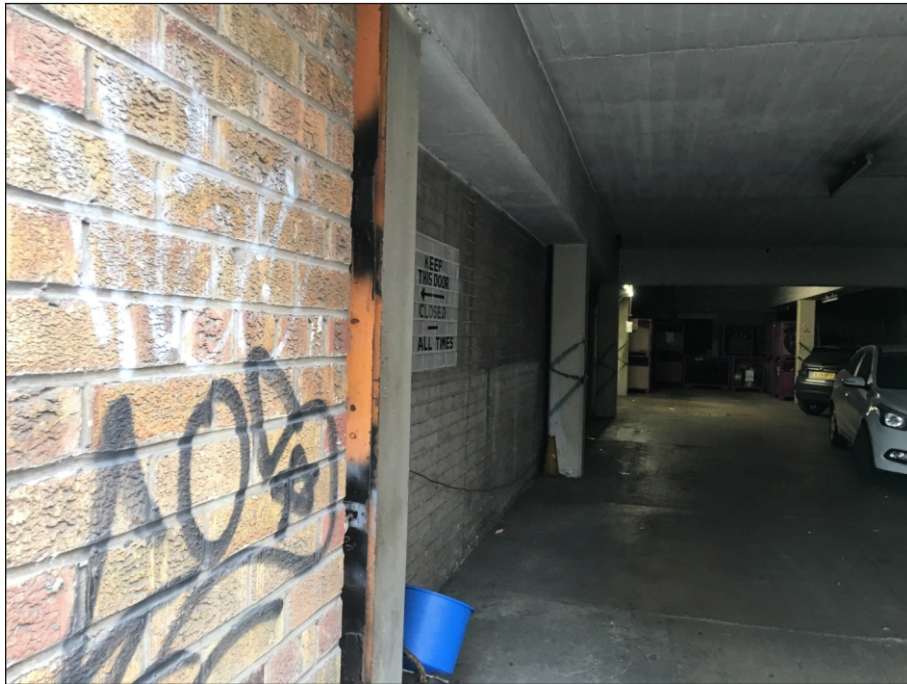
Plate 37: Easternmost doorway facing onto Hollis Croft leading to car park
