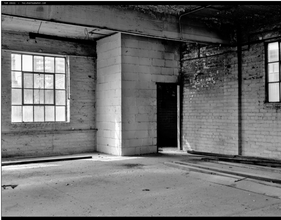
Plate 91: Internal view of Building 14, looking north-west
