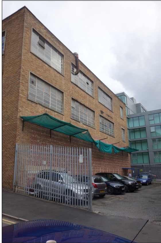
Plate 29: East elevation of Building 3 facing onto an external car park
