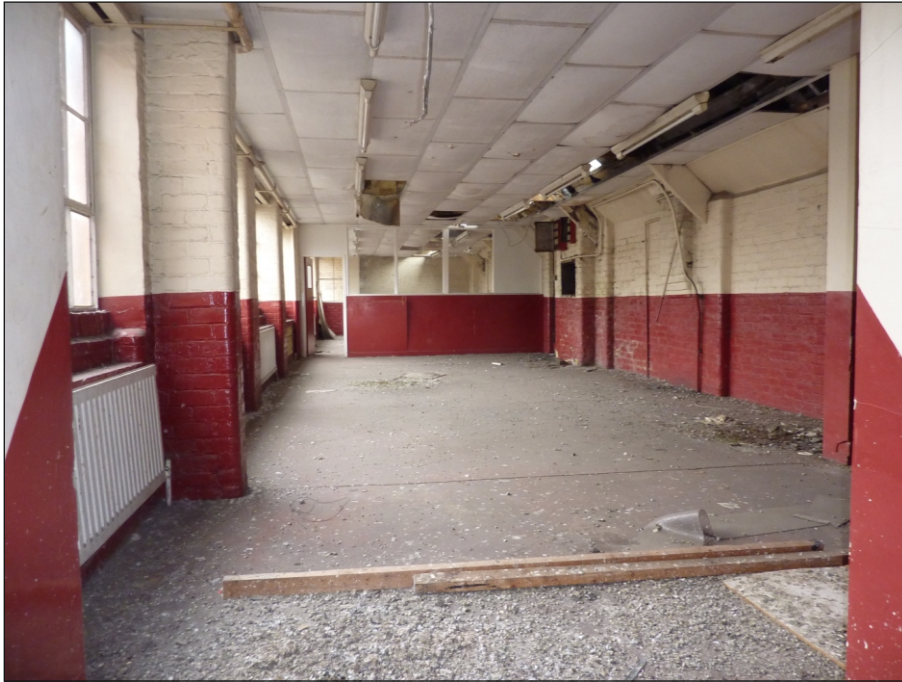
Plate 107: Uppermost floor of Building 17, looking south
