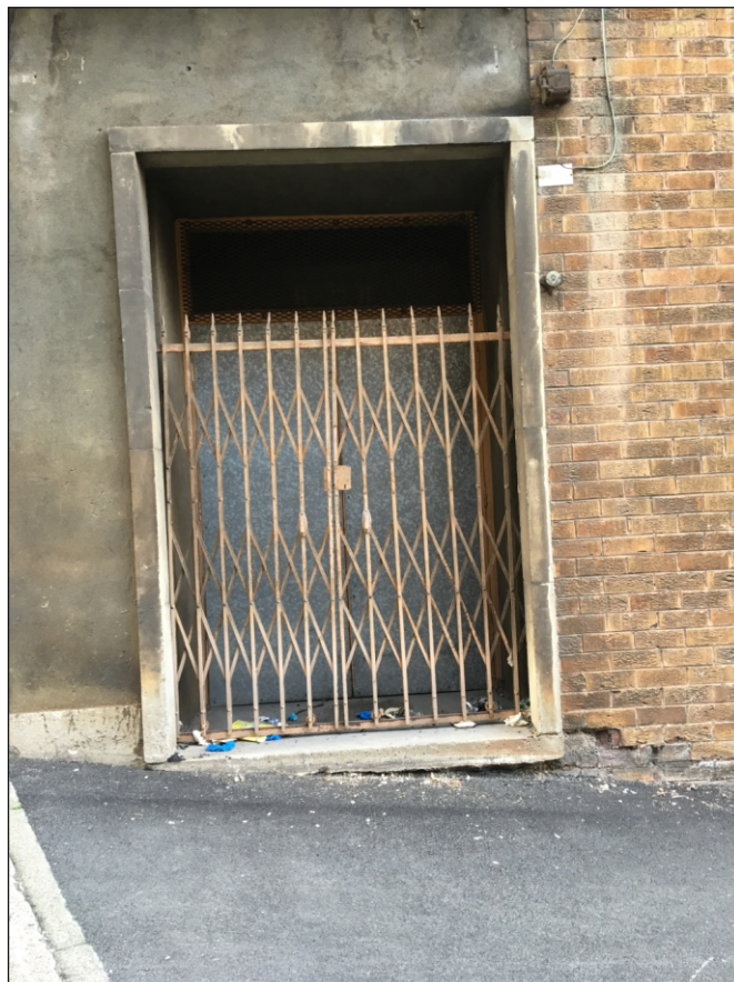
Plate 25: Metal sliding shutter to the east of Gate 4
