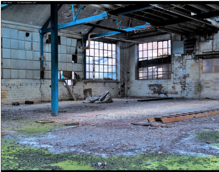
Plate 96: First floor of Building 15, looking north-west
