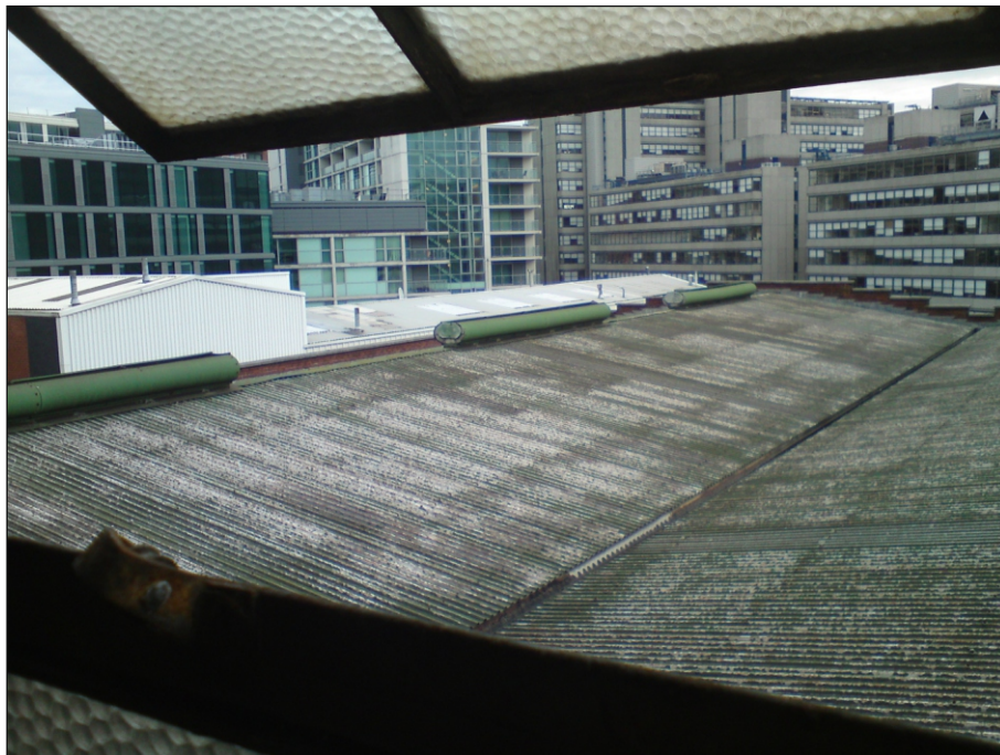
Plate 36: Detail of double shallow pitched roof with central valley of Building 4
