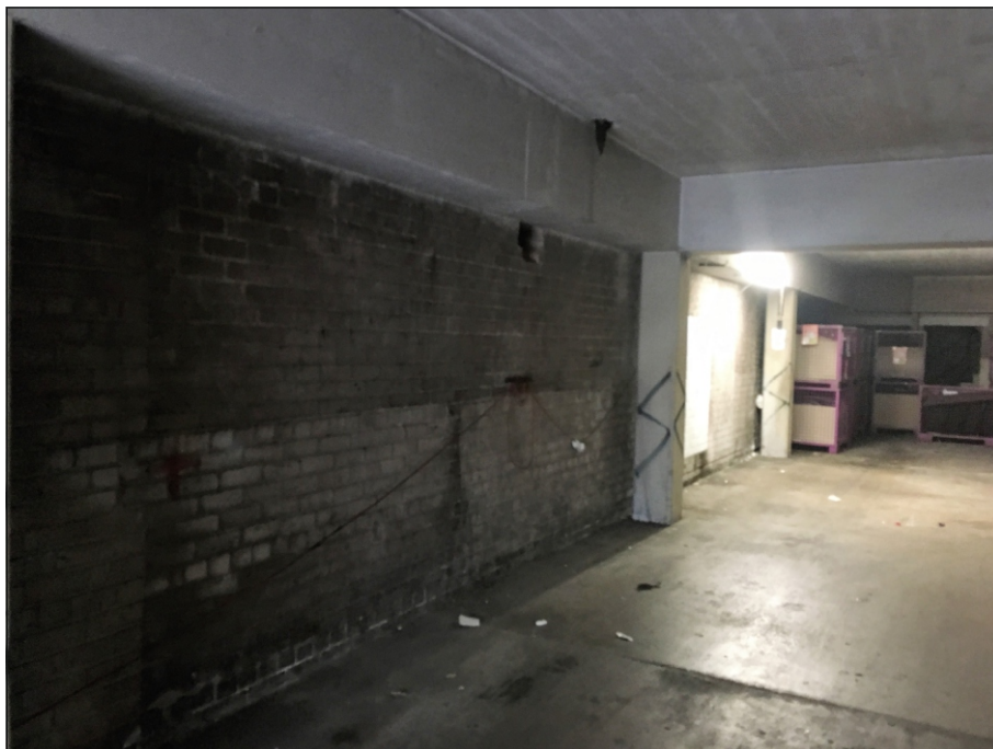
Plate 38: Car park area within Building 4
