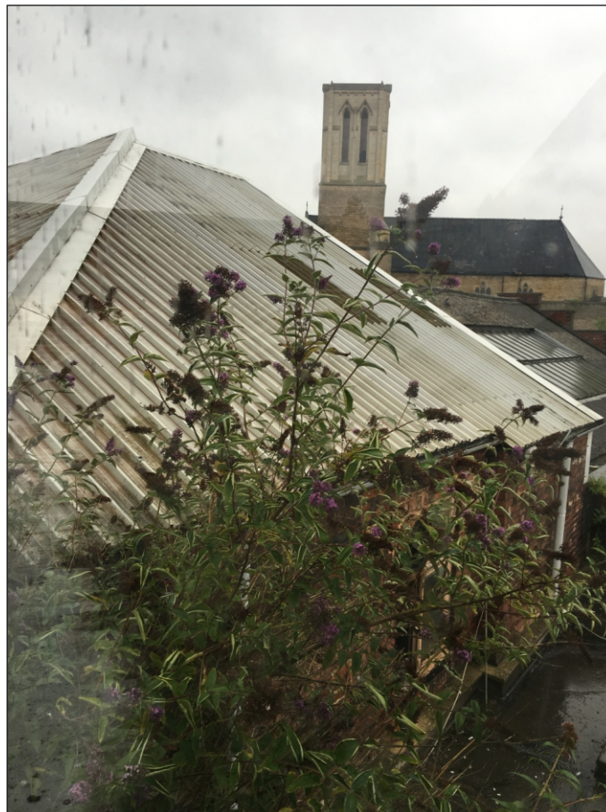
Plate 58: View of the southern hipped section of the roof, looking north
