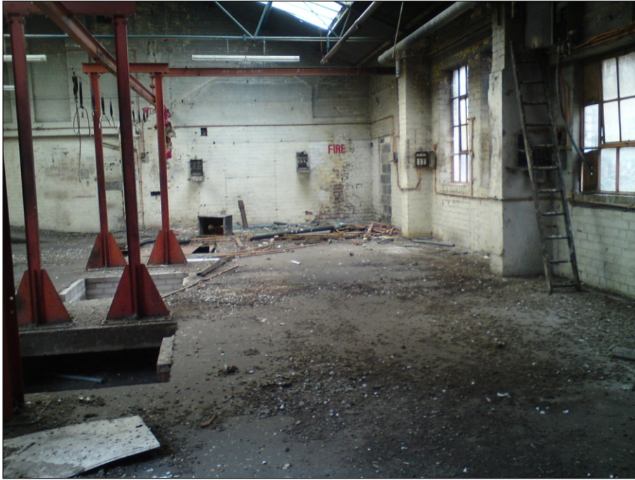
Plate 93: First floor of Building 16, looking south
