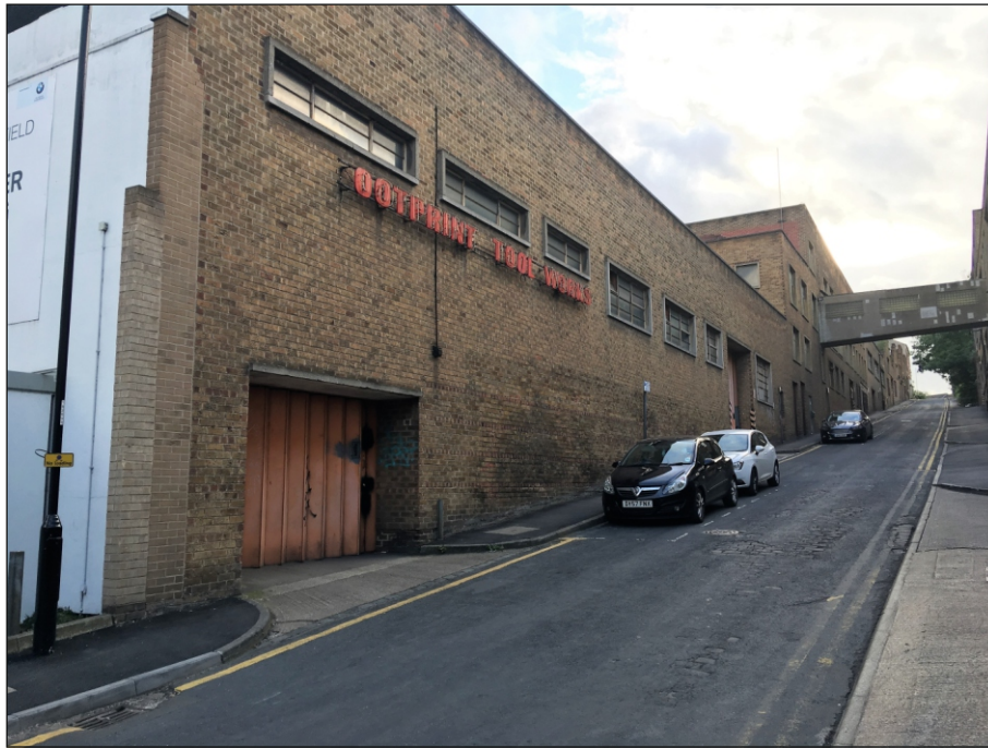
Plate 31: General view of Building 4 along Hollis Croft
