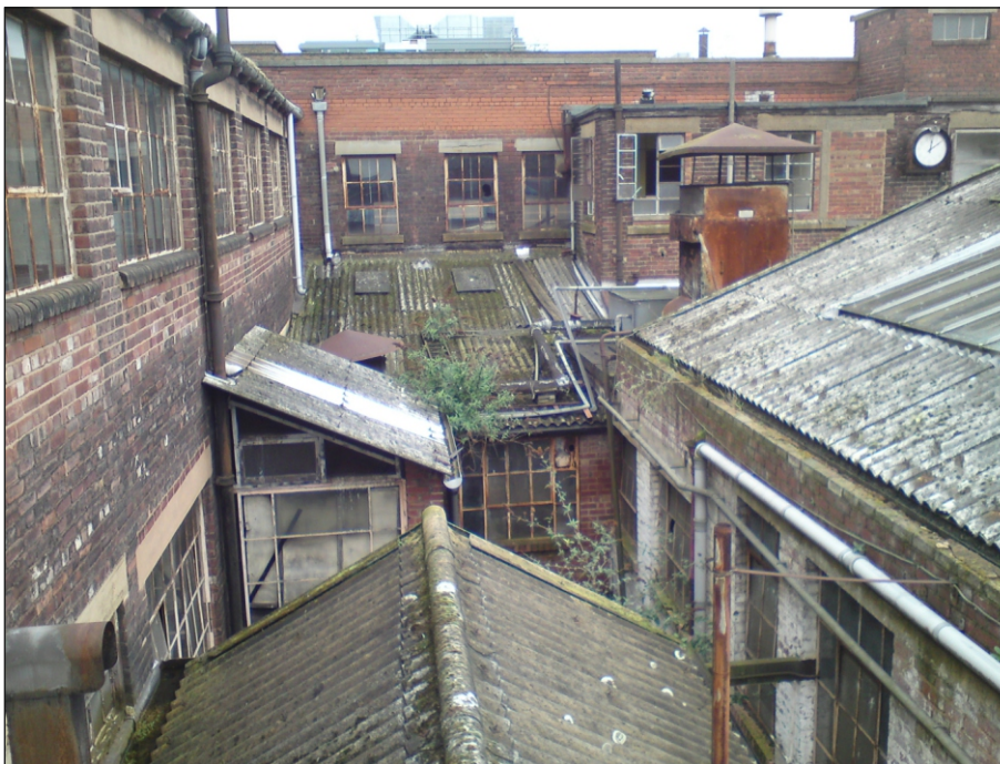
Plate 110: Court 2, looking north
