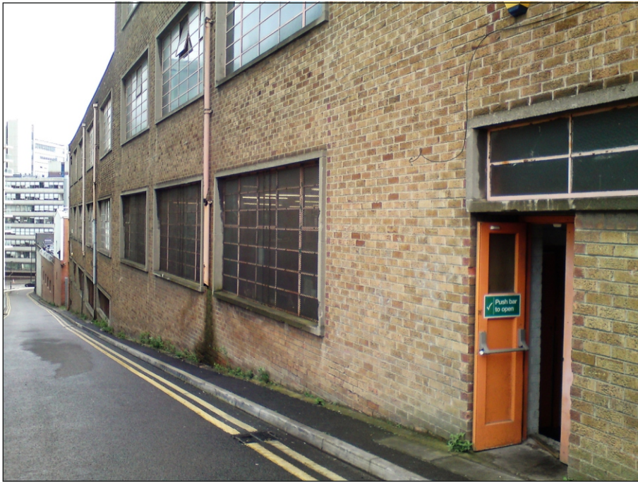
Plate 17: Detail of inserted fire exit doorway to the western end of Building 2
