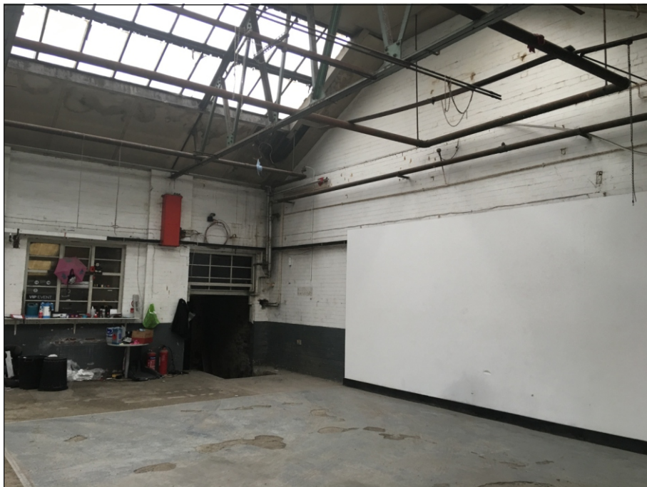
Plate 62: Internal view of Building 9
