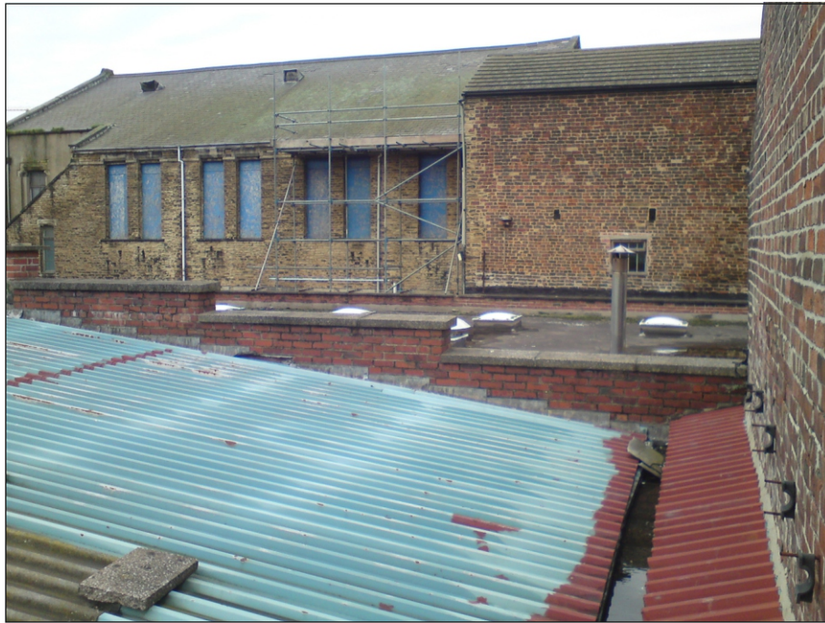
Plate 79: Stepped parapetted gable concealing the shallow pitched roof of Building 12
