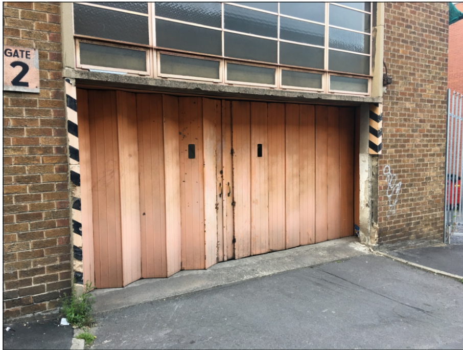
Plate 21: Detail of concertina doorway - Gate 2 - of Building 3
