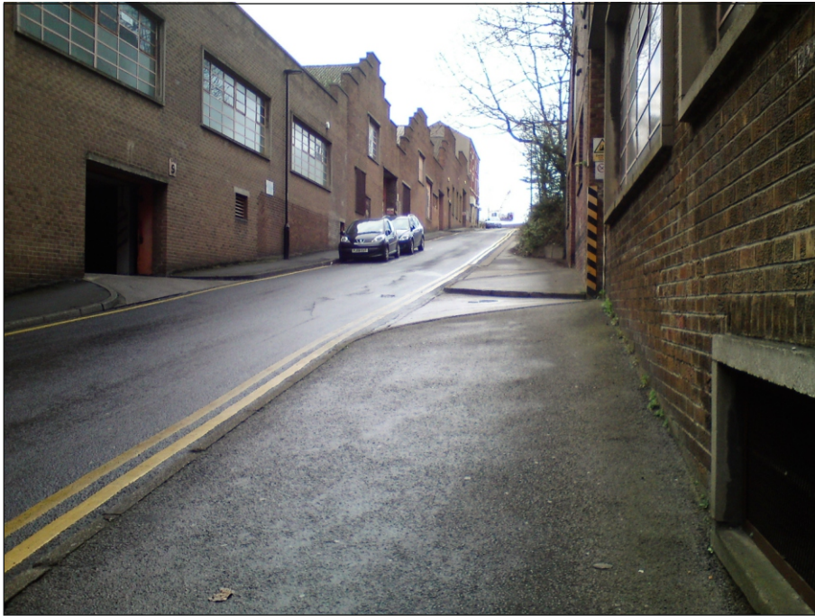
Plate 55: Front elevation of Building 7 facing onto Hollis Croft
