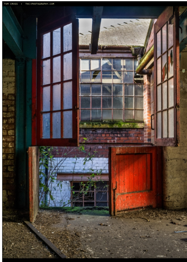
Plate 102: First floor of Building 16, looking east
