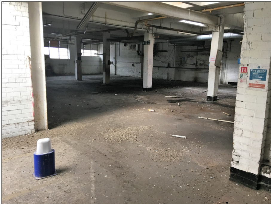
Plate 88: Western side of the ground floor of Building 13
