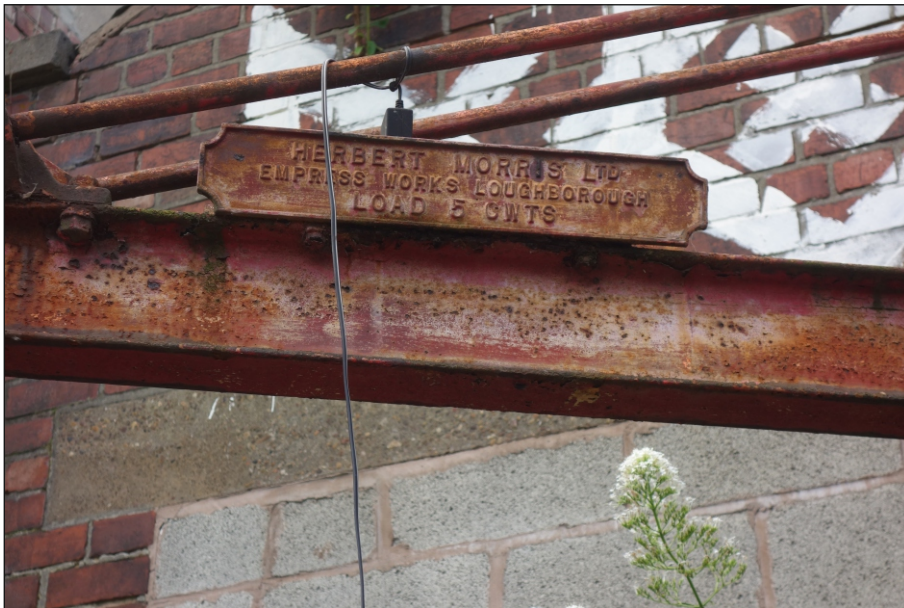
Plate 10: Crane maker's plate
