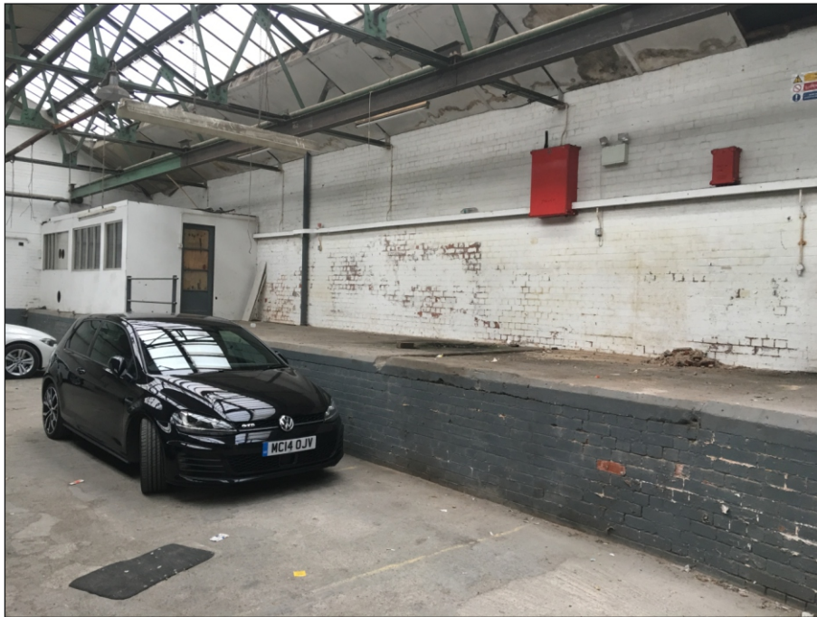
Plate 67: Internal view of Building 10, looking south-west
