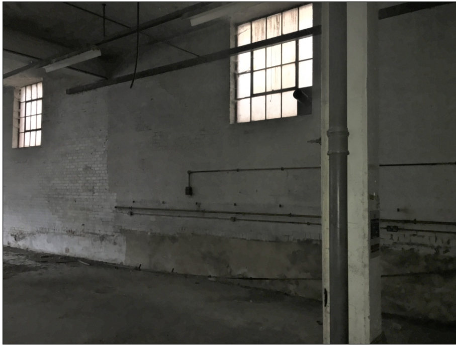
Plate 73: Inside Building 11, looking south-west
