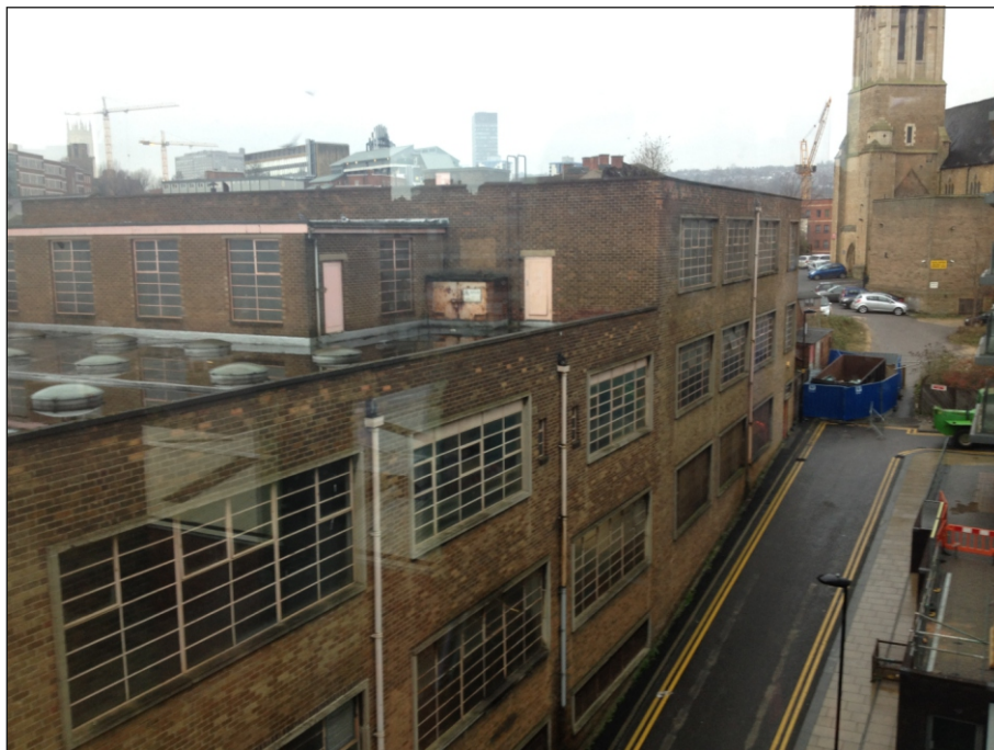
Plate 16: Rear elevation of Building 2, viewed from the east
