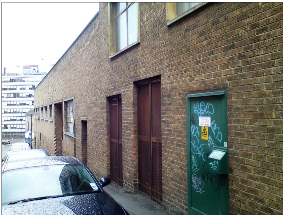
Plate 44: Inserted doorways within the north elevation of Building 5, looking east
