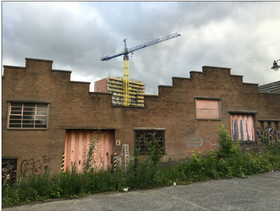
Plate 61: Front elevation of Building 9 (to the right) facing onto Hollis Croft
