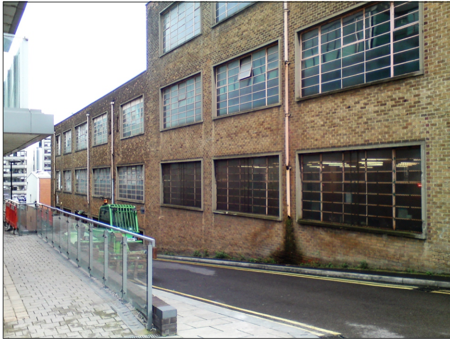
Plate 27: General view of the rear elevation of Building 3
