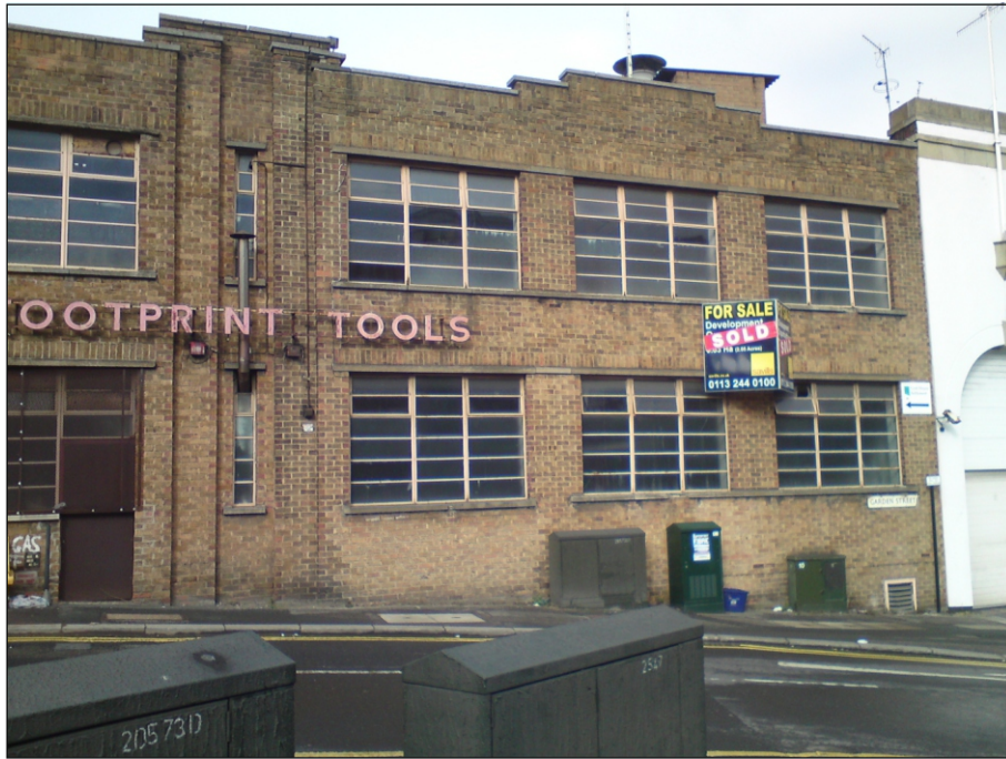
Plate 83: Eastern side of the front elevation of Building 13
