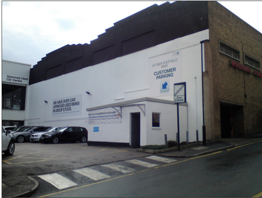
Plate 35: East elevation of Building 4
