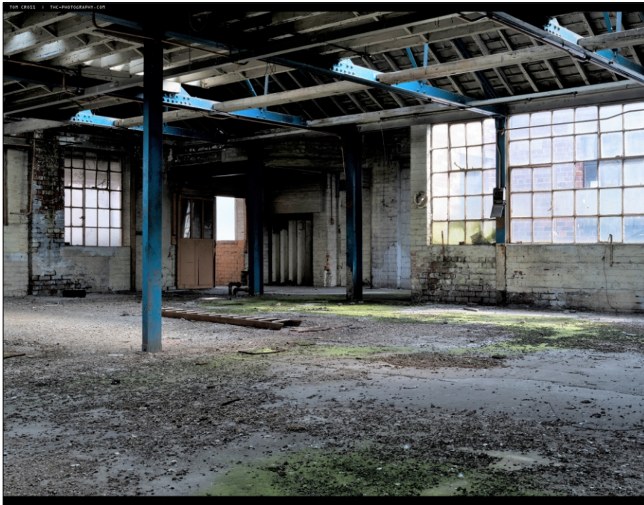
Plate 95: First floor of Building 15, looking north-east
