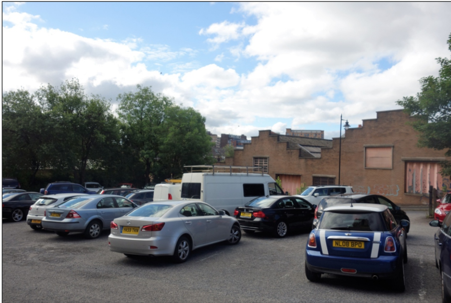
Plate 57: Front elevation of Building 8 viewed from a car park to the north
