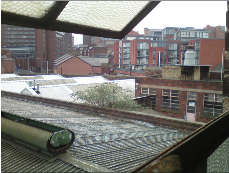
Plate 85: Rear elevation of Building 13 facing onto Court 1
