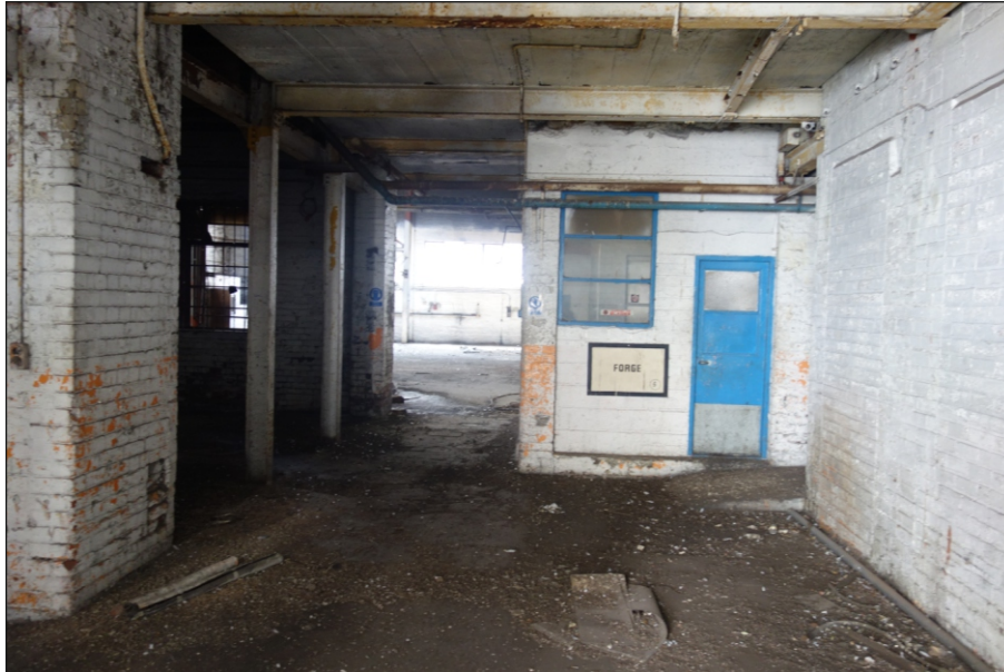
Plate 101: Ground floor of Building 16, looking west
