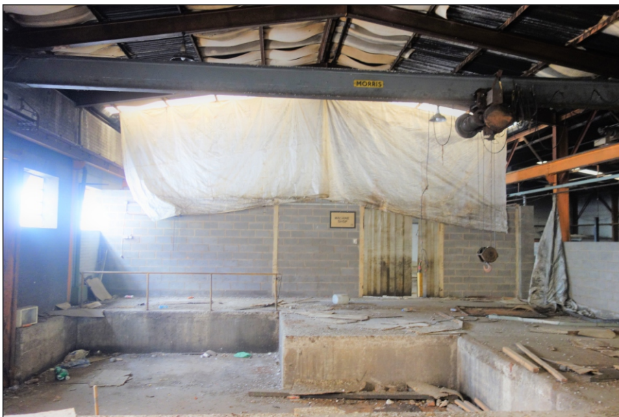
Plate 40: Workshop area within Building 4, looking east
