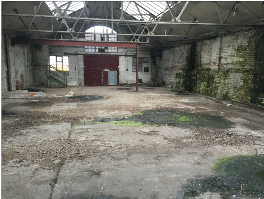
Plate 11: Internal view of Building 1, looking south
