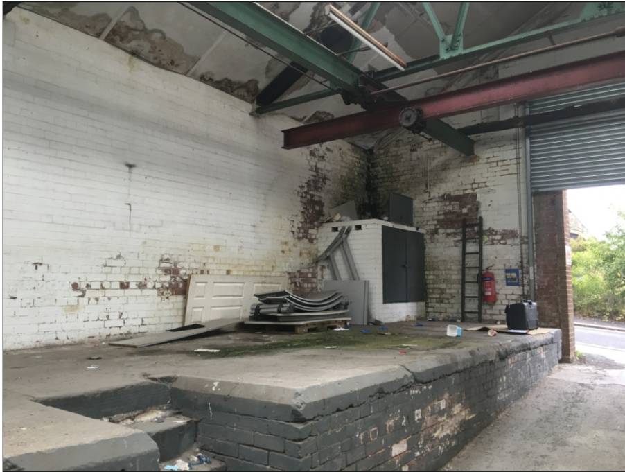
Plate 69: Internal view of Building 10 looking towards the doorway with roller shutter
