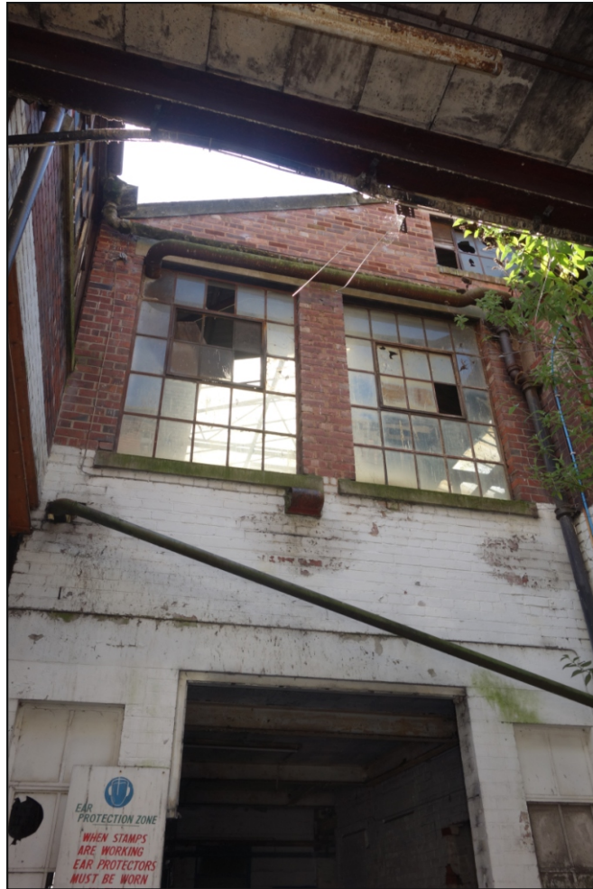
Plate 97: Gable wall of Building 16
