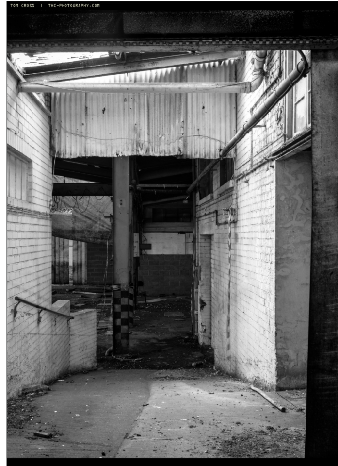
Plate 48: Building 5 extension to the left along a ramp down to Building 4
