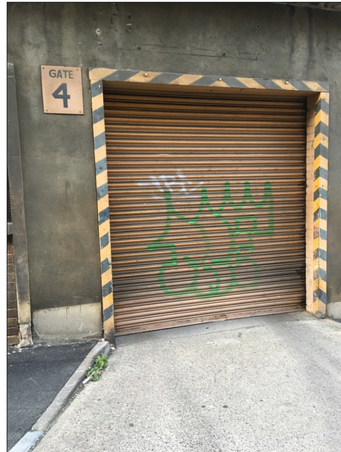
Plate 24: Detail of roller shutter - Gate 4 - along Hollis Croft
