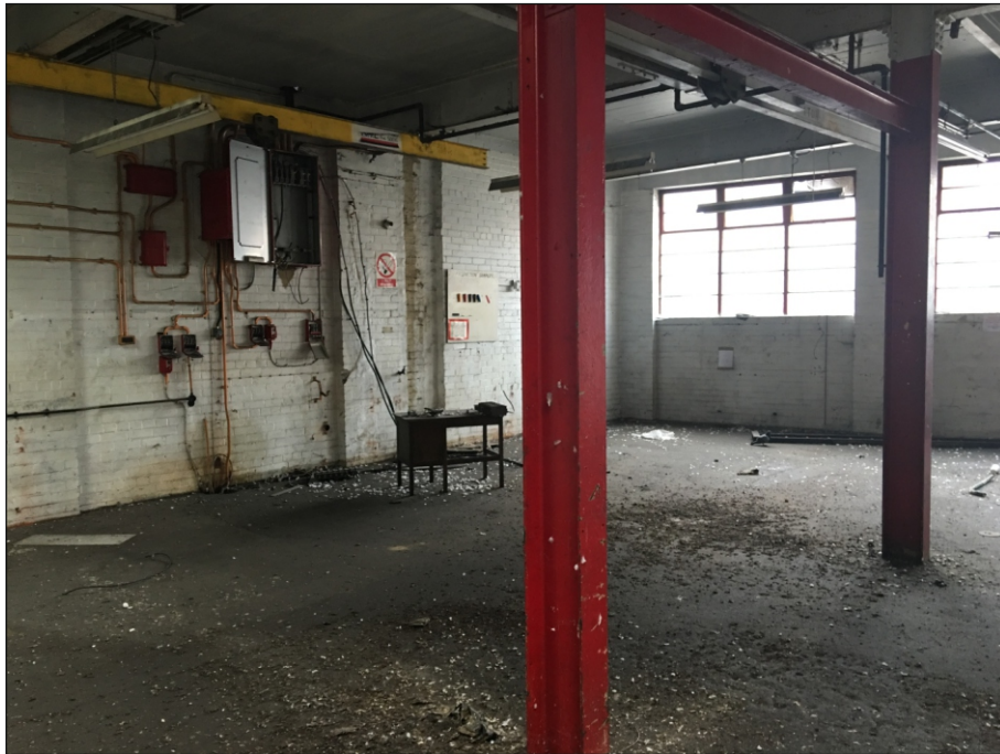
Plate 87: Eastern side of Building 13, looking south-east
