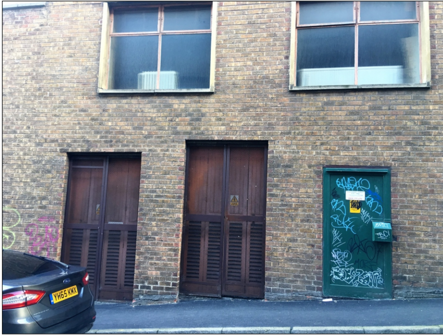
Plate 45: Detail of inserted doorways, looking south
