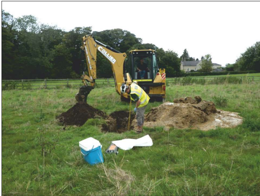
Plate 1: General shot of geotechnical test pitting
