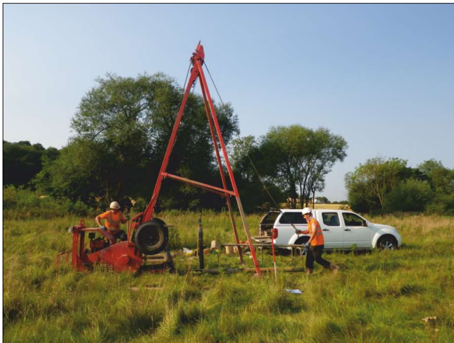
Plate 2: General shot of borehole preparation
