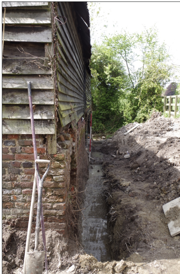
Plate 6: Underpinning trench, viewed from the west
