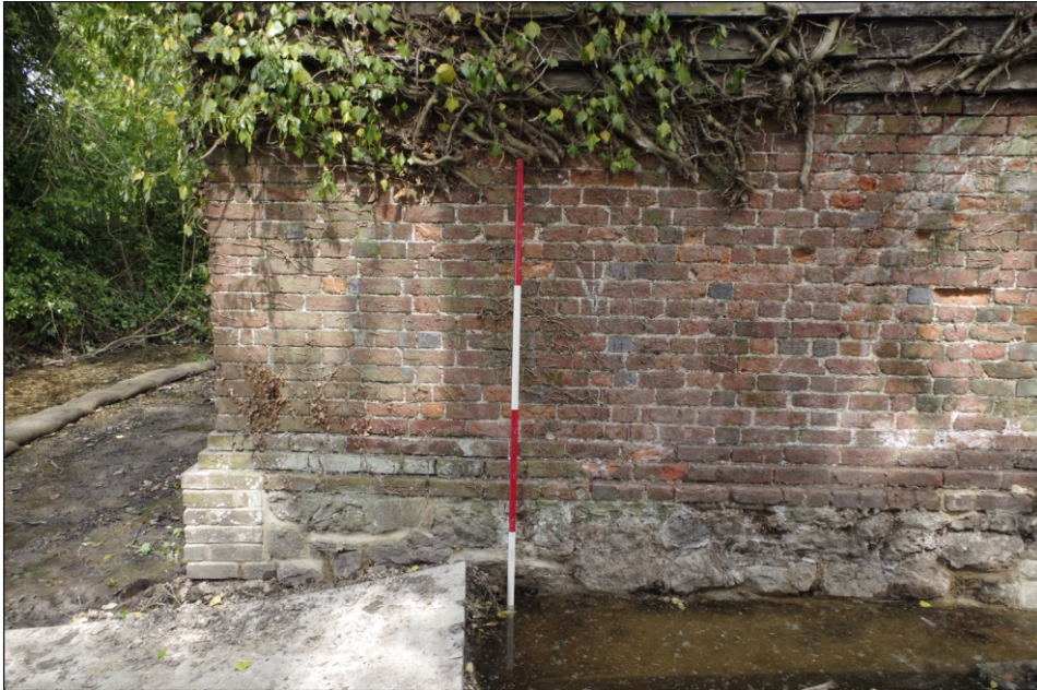
Plate 5: Barn wall and foundation, viewed from the south
